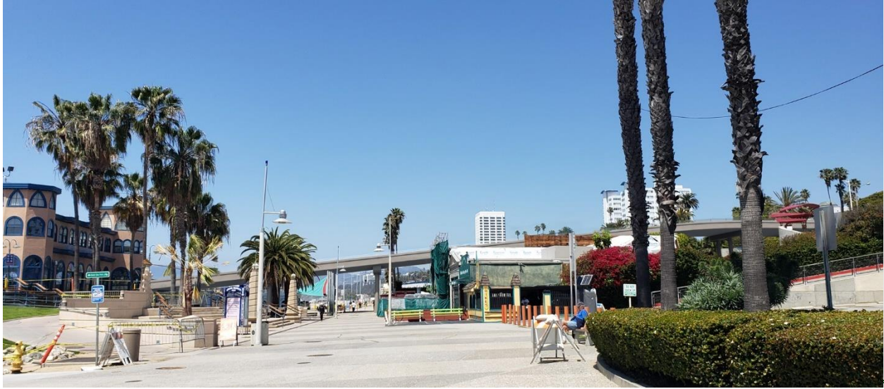
Alternative 2: View north toward Bridge from Ocean Front Walk.
