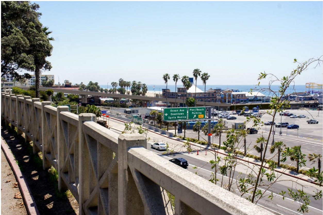
Alternative 2: View south toward Bridge and Pier from Palisades Park.
