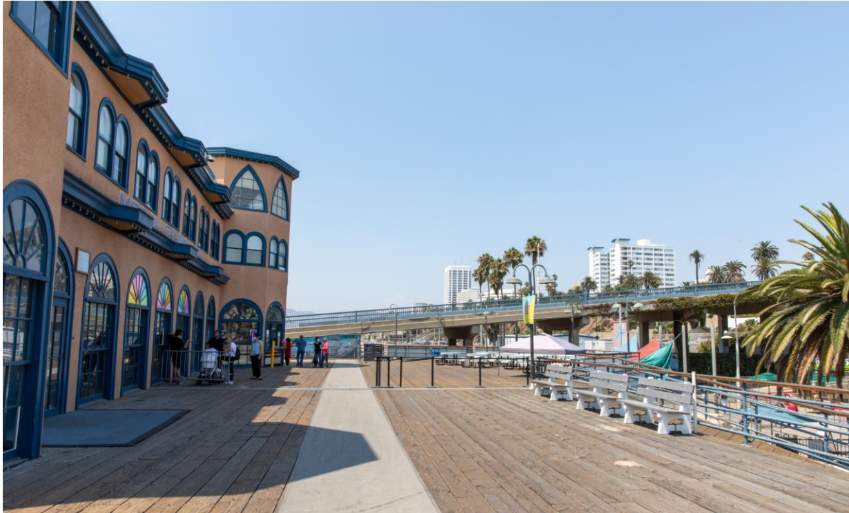
View north toward Bridge from the Pier deck in front of Loeff's Hippodrome.
