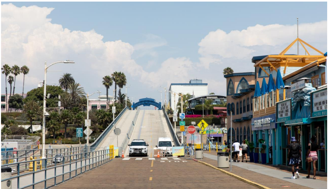
View east from Pier deck with Pier Sign in background.
