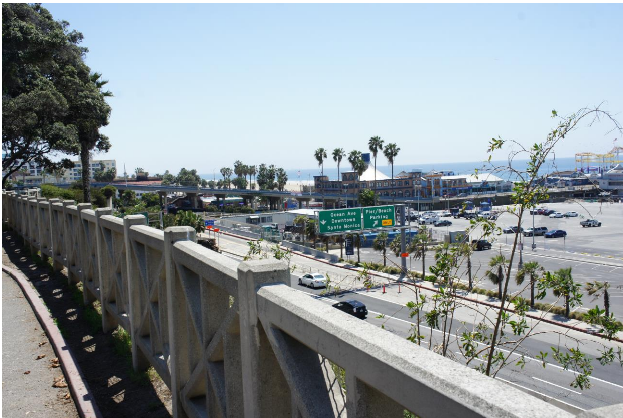
View south from Palisades Park toward Bridge and Pier.
