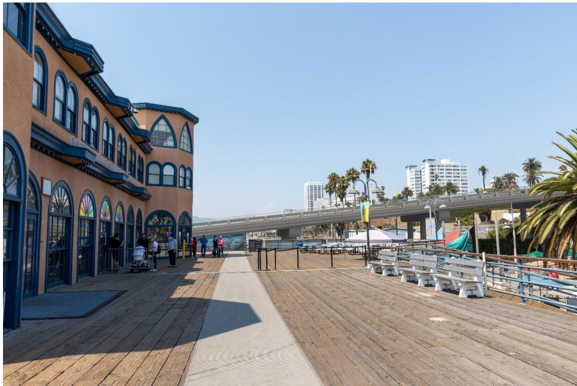
Alternative 1: View north toward Bridge from the Pier deck in front of Loeff's Hippodrome.
