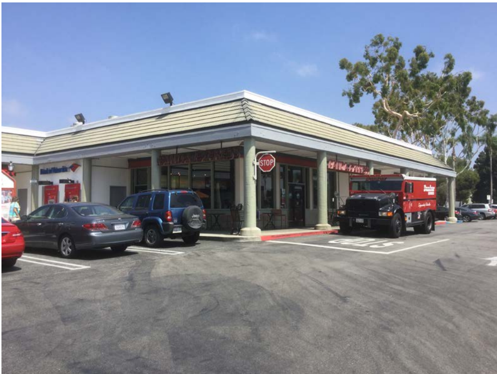
Eastern portion of the structure at 4325 Glencoe Avenue. 4325 Glencoe Avenue, Los Angeles, California 90292
