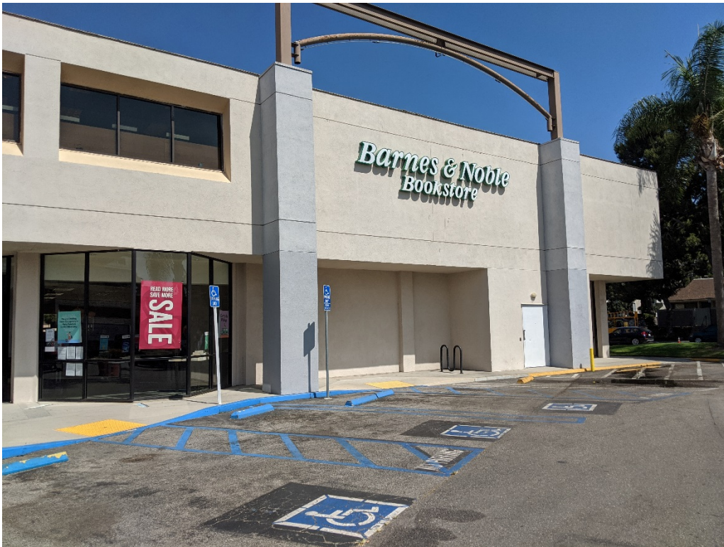
View of the structure at 13400 Maxella Avenue. 13400 Maxella Avenue, Los Angeles, California 90292
