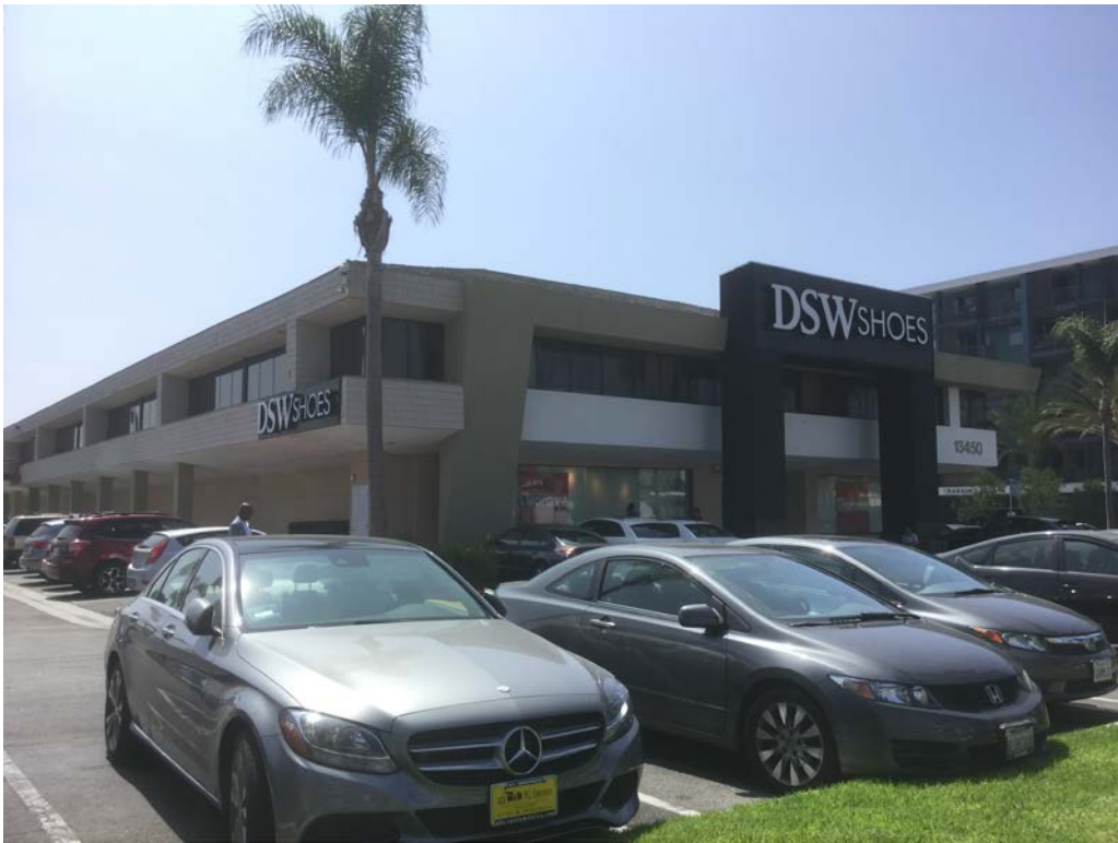
View of the structure at 13450 Maxella Avenue. 13450 Maxella Avenue, Los Angeles, California 90292
