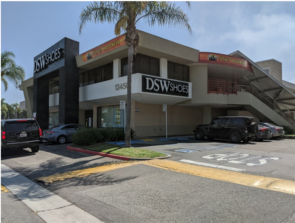
View of the structure at 13450 Maxella Avenue. 13450 Maxella Avenue, Los Angeles, California 90292
