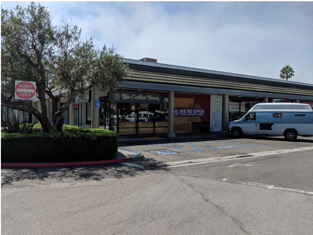
View of the structure at 4325 Glencoe Avenue. 4325 Glencoe Avenue, Los Angeles, California 90292
