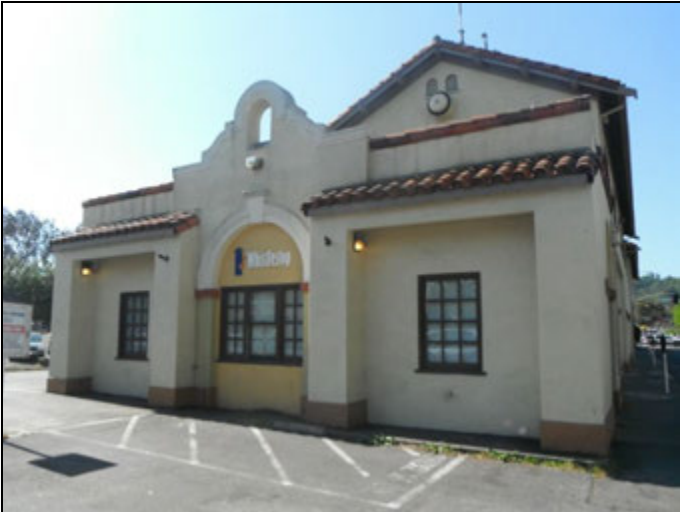
Photograph 3. Northwestern Pacific Depot. 930 Tamalpais Ave. View south.
