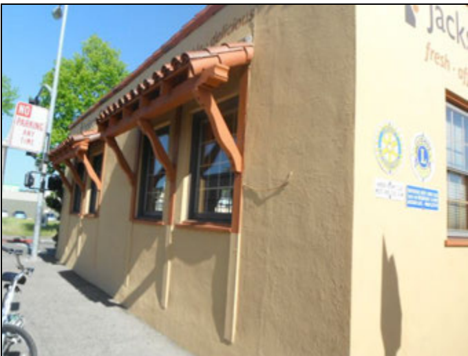
Photograph 5. Northwestern Pacific Depot. 930 Tamalpais Ave. View northwest.
