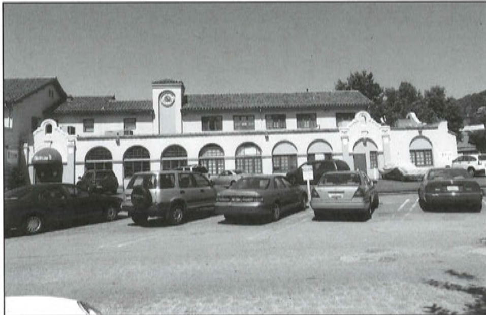
Photograph 3: Second-story addition and clock tower were constructed in 1987. Also note arched windows that were formerly an open arcade.
