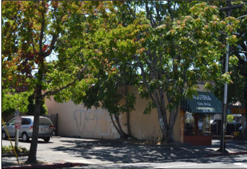
Figure 2. View of primary (north) and east façades, facing southwest. Source: ICF 8/11/2020.
