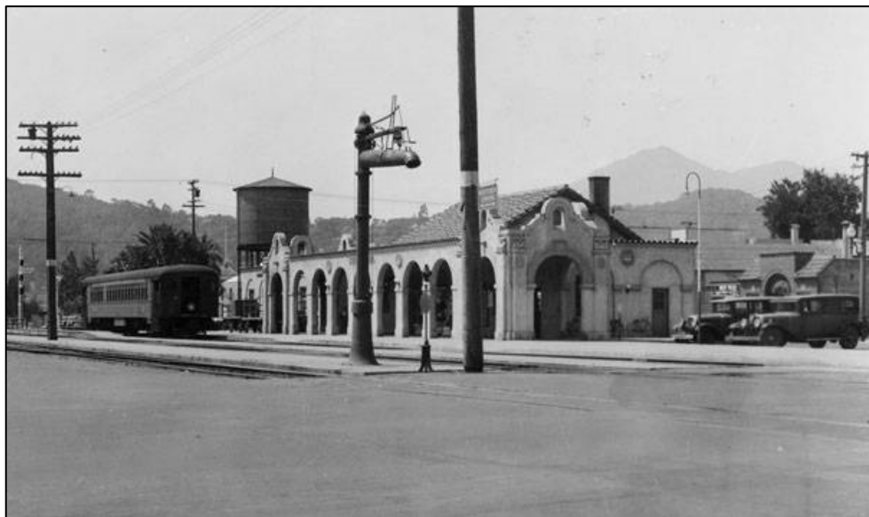
Figure 3. 1935 photo of unenclosed passenger arcade, viewed facing southwest. The gabled roof to the passenger waiting room is visible behind the mission-style parapets near the center of the image. Source: Northwest Pacific Railroad Historical Society, via San Rafael Heritage.
