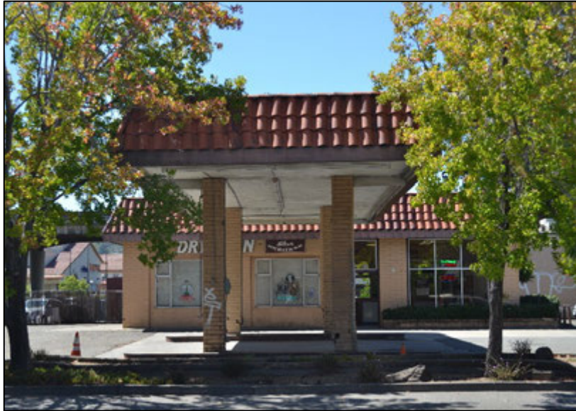
Figure 2. View of primary (east) façade and canopy, facing west. Source: ICF 8/11/2020.
