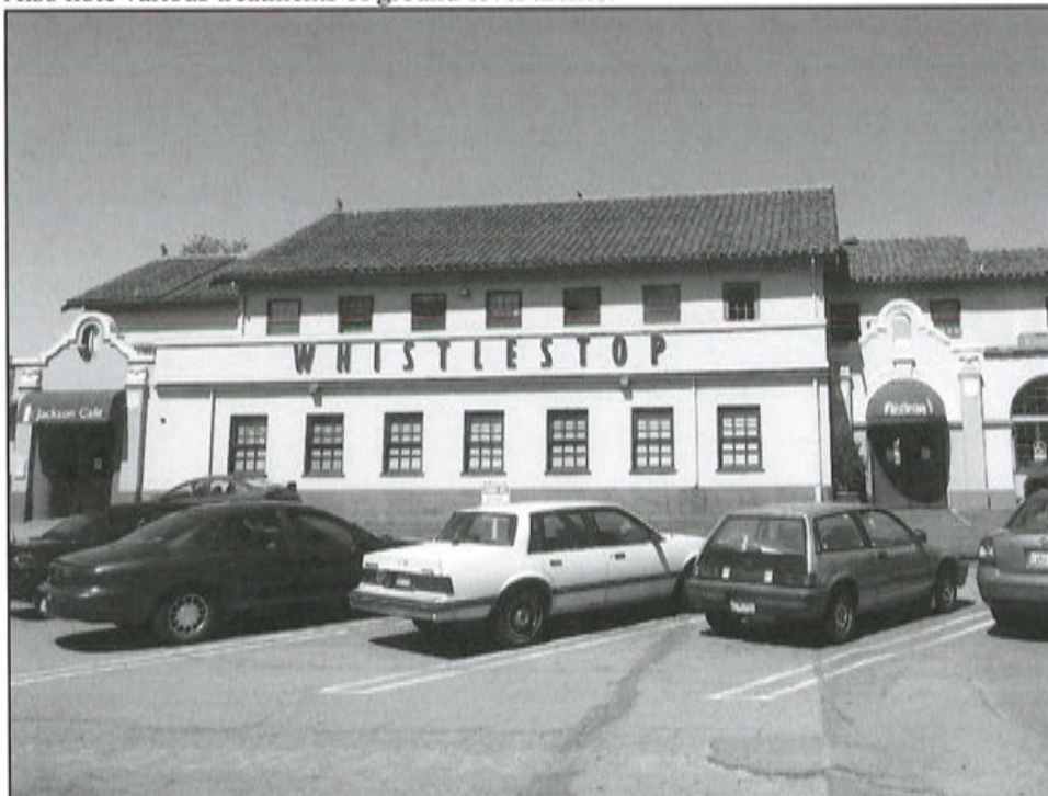
Photograph 6: Mid-section of east side. 1985 second-story addition above 1939-1946 addition, camera facing west.
