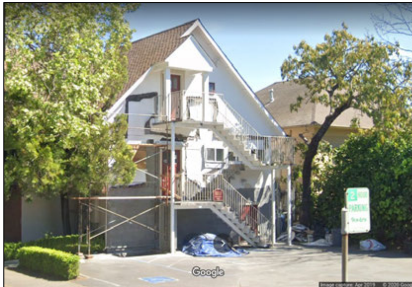
Figure 3. View of rear (west) façade, facing southeast. Source: Google, April 2019.
