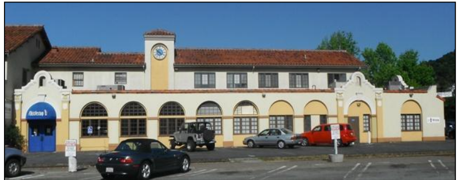
Photograph 2. East elevation of San Rafael depot showing infill of the arched arcade and an addition at the north end. Photograph taken on April 22, 2013.
