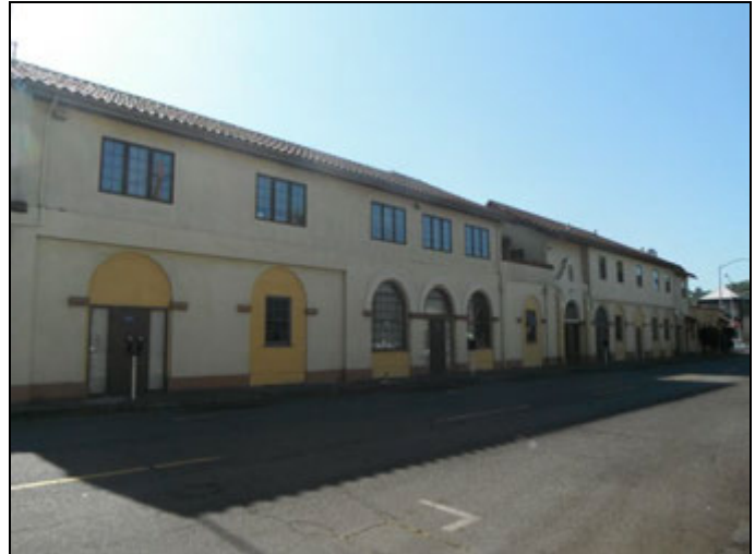
Photograph 4. Northwestern Pacific Depot. 930 Tamalpais Ave. View southeast.
