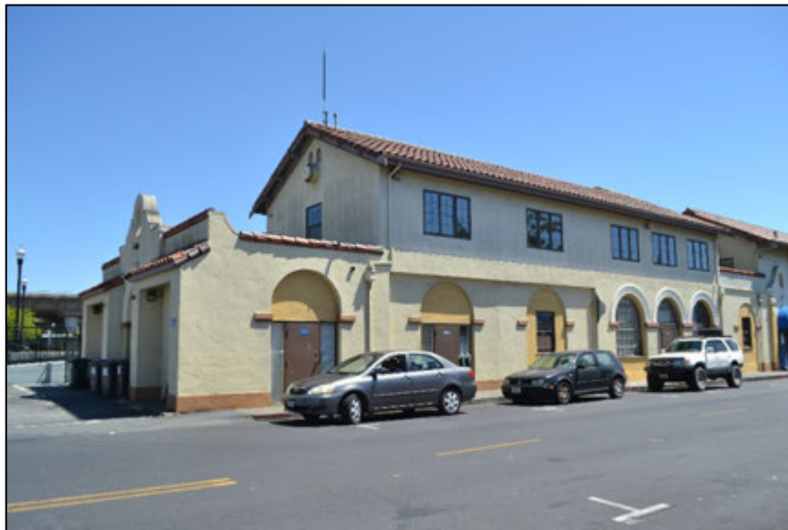
Figure 8. North end of the building, viewed facing southeast. The non-historic north addition is at left, and the 1980s-era upper-story addition is visible at the center of the image. The three divided-lite arched windows that originally belonged to the passenger waiting room are located at right; the original roof of that volume was removed to accommodate the second-story addition.
