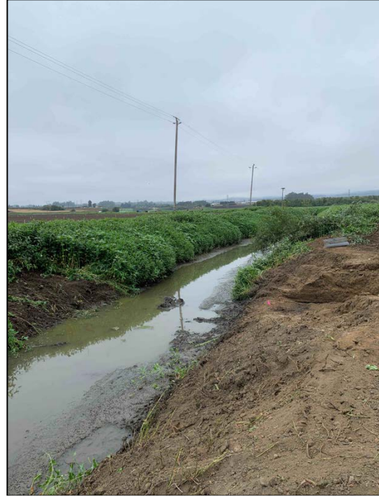
Photo 2. College Lake drainage channel 150 ft upstream of existing weir, August 11, 2020
