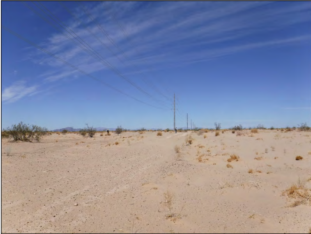
Figure 6.17. Active aeolian dune deposits on top of stabilized aeolian and dune deposits (Qe) within the gen-tie corridor.
