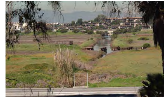
No fence at area B
