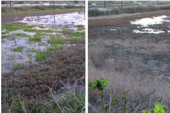
How the developers' secret drainage system wiped out Ballona's life-giving water.
