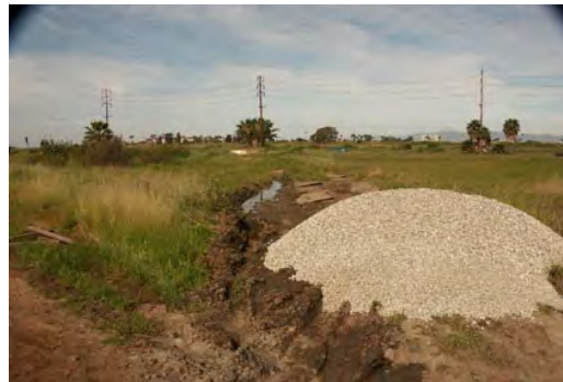
Dumping in the wetland destroys habitat
