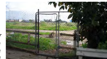
Unlocked gate at area C
