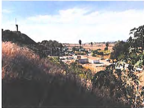
SOCALGAS GAS STORAGE FIELD TANK FARM CULVER BLVD, PLAYA DEL REY, CA
