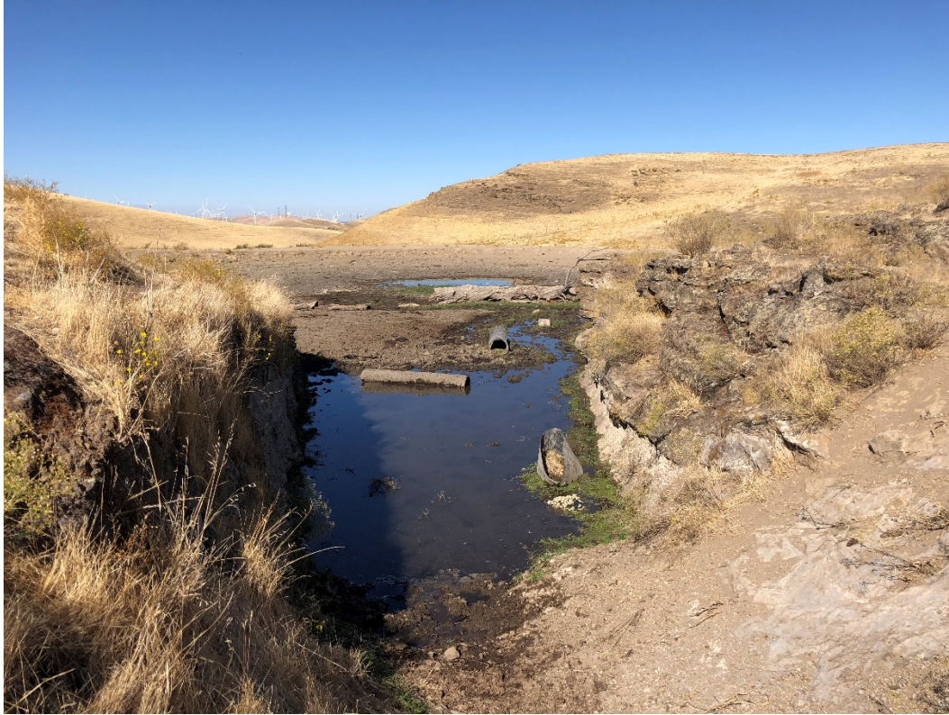
Looking north at Pond L on October 28, 2019
