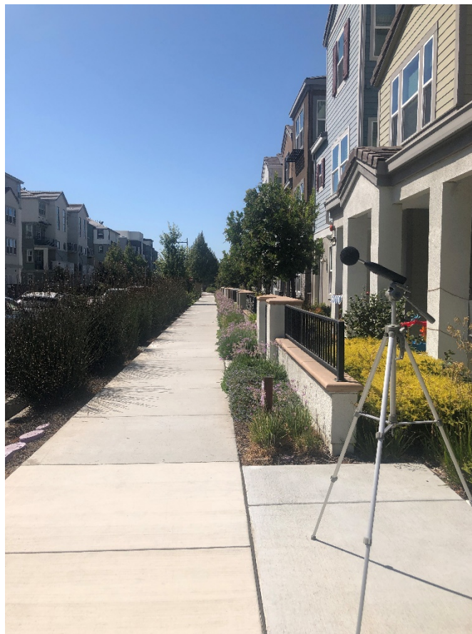
Looking west towards Garden Street/Merry Loop intersection.
