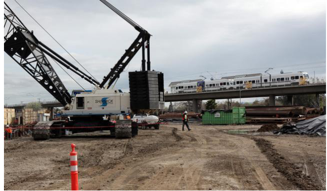
The BART extension of the Warm Springs/ South Fremont line through Milpitas began construction in 2015 and opened for service in 2020. (The Mercury News)
