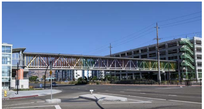
Public realm improvements near the Milpitas Transit Center include open spaces, streetscape improvements, and new pedestrian overhead bridges.
