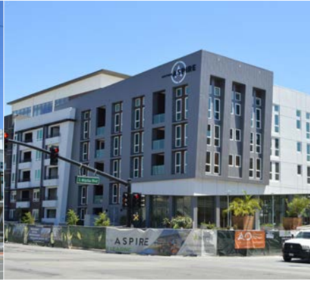
Anton Aspire Apartments: New high-density residential development in the Tango District.
