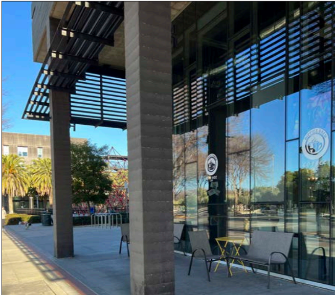
Example of the ground floor treatment on an Activity Street with visibility of active uses, and pedestrian oriented details.
