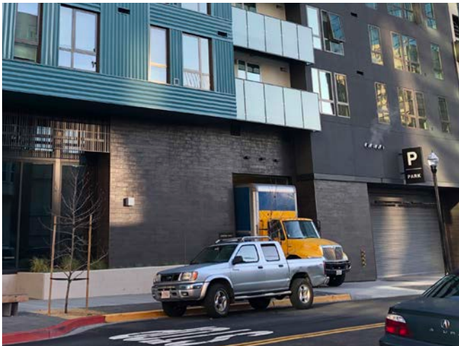
This example shows the service entrance treated with the same architectural character as the rest of the building and located away from active entries by a loading zone.
