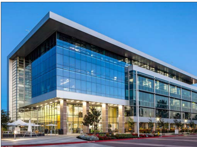
Examples of research and development building design in Northern California.
