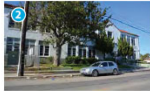
Worthington Elementary School
