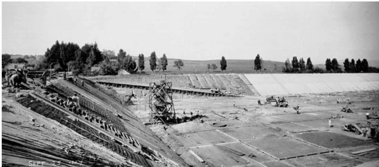
Exhibit 9. Construction of the Bay Street Reservoir in 1924 (SCPL 1924).
