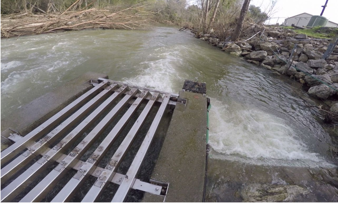
TAIT DIVERSION FACILITY – LOOKING DOWNSTREAM
