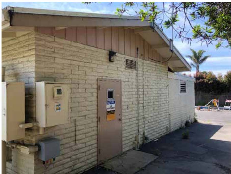
Exhibit 2. Control Building, west elevation, view looking southeast (IMG_0222).
