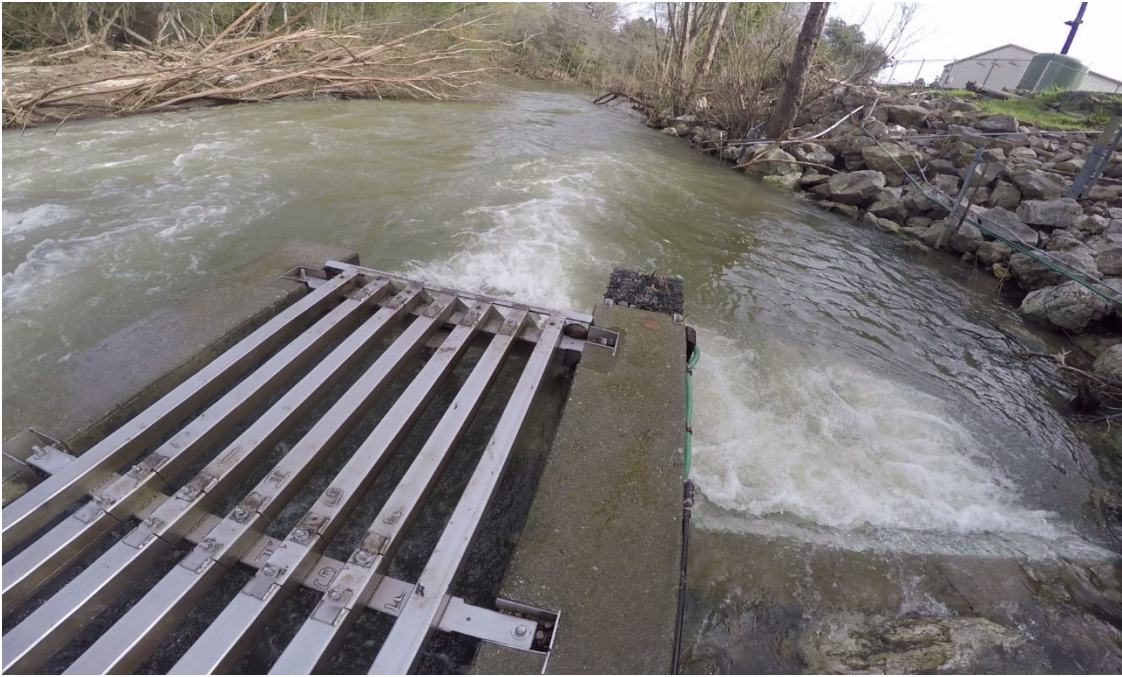
TAIT DIVERSION FACILITY – LOOKING DOWNSTREAM
