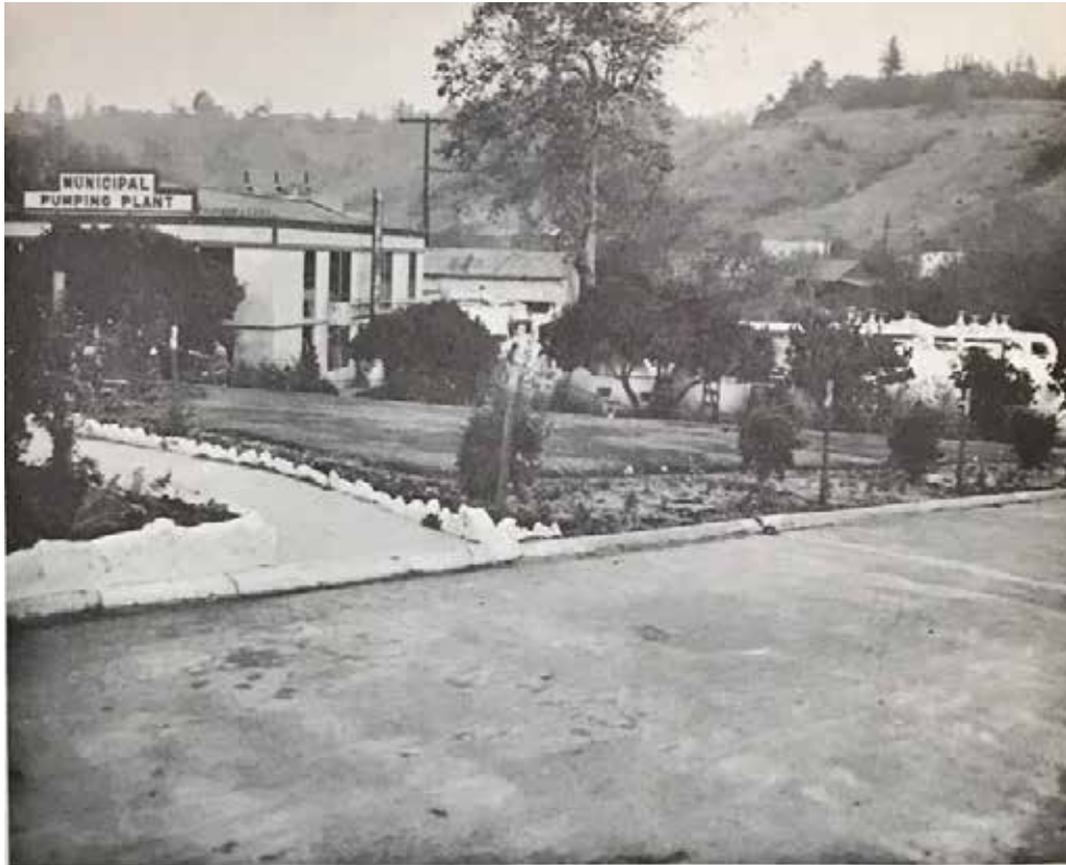
SANTA CRUZ MUNICIPAL PUMPING PLANT. Building houses low and high lift pumps and engine-driven generators. Pressure type filters are at right of building.
