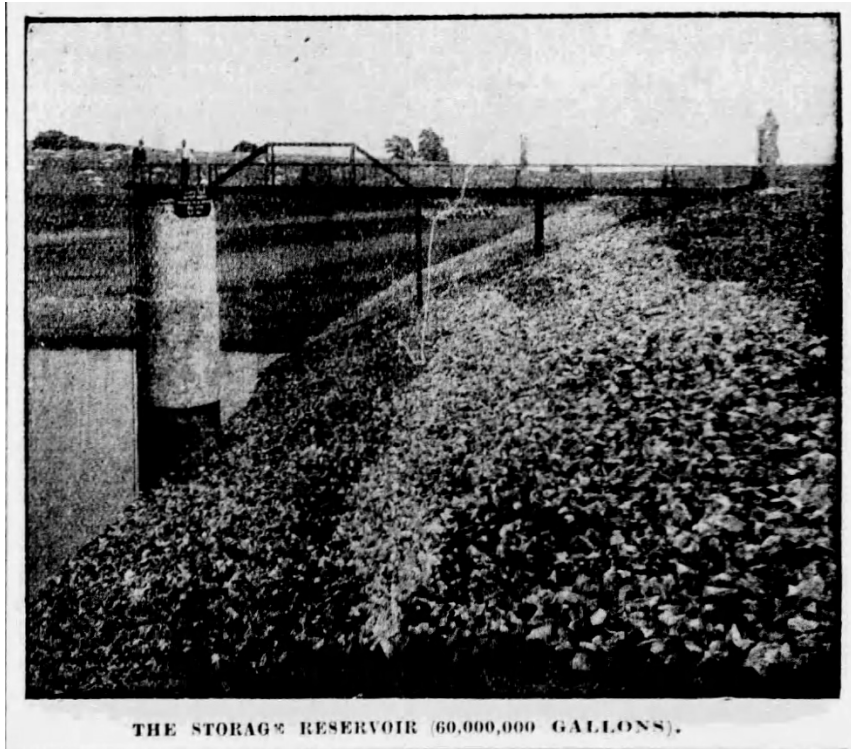
Exhibit 8. The earliest known photograph of the Cowell Street Reservoir published in the Santa Cruz Surf in 1892 ( Santa Cruz Surf 1892: 2).
