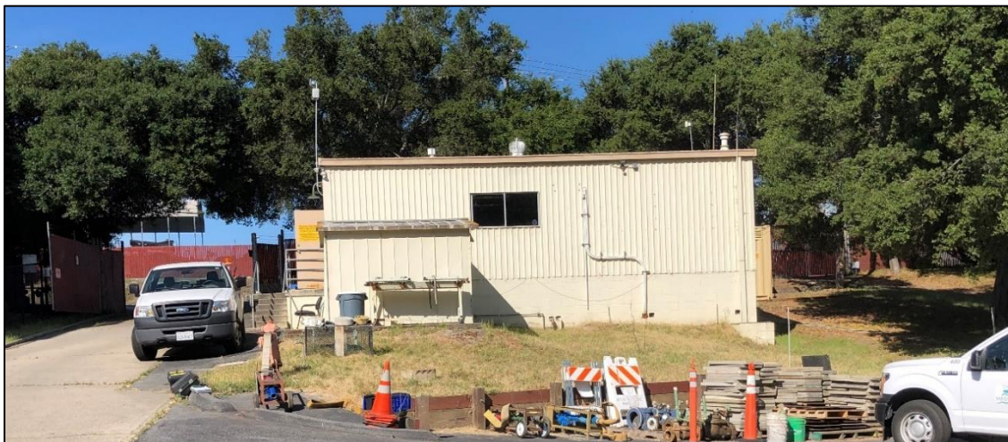
Exhibit 20. Meter Shop, northeast elevation, view looking west (IMG_0184)
