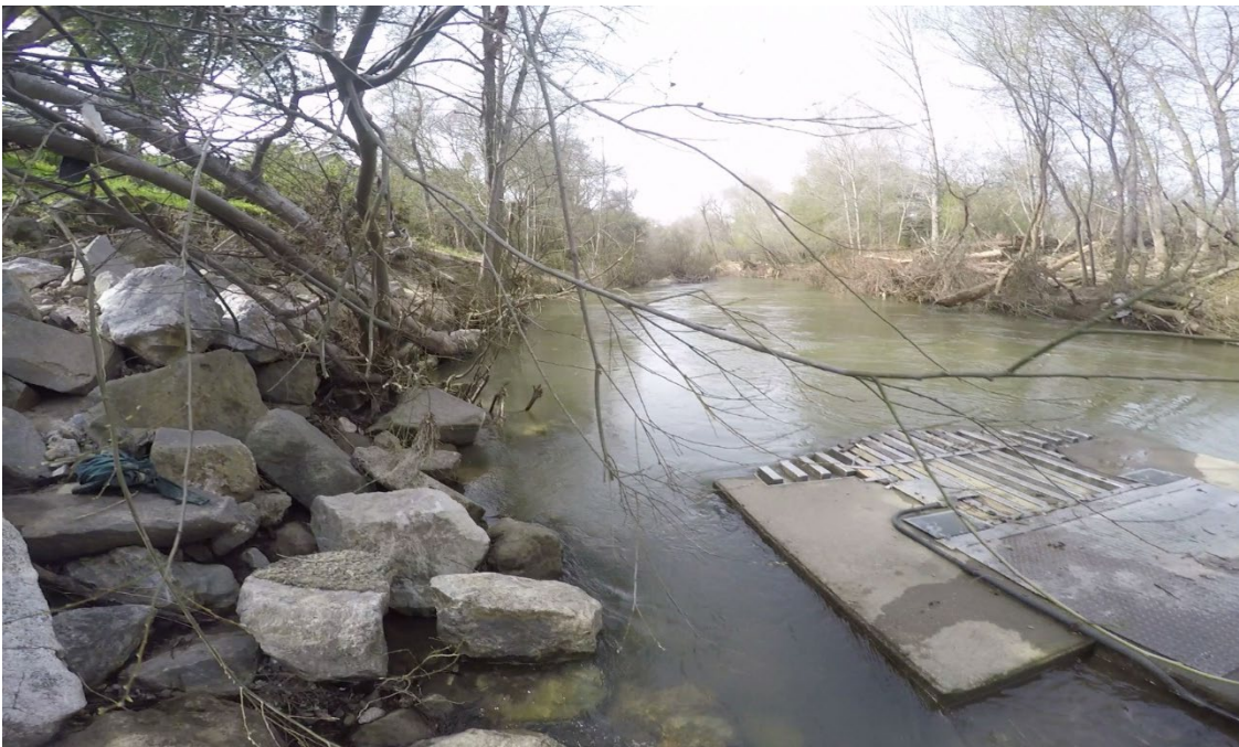
TAIT DIVERSION FACILITY- LOOKING UPSTREAM
