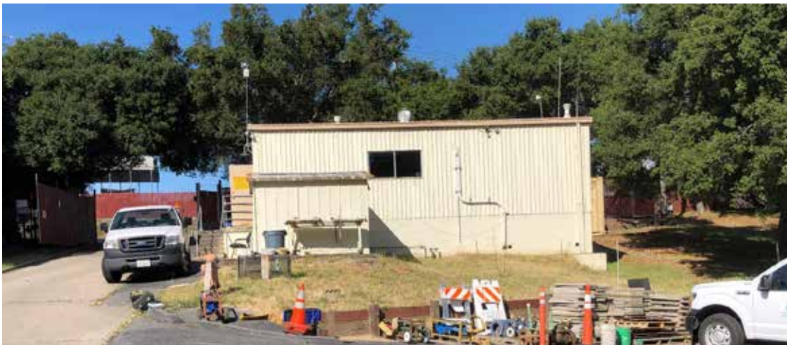
Exhibit 4. Meter Shop, northeast elevation, view looking west (IMG_0184)
