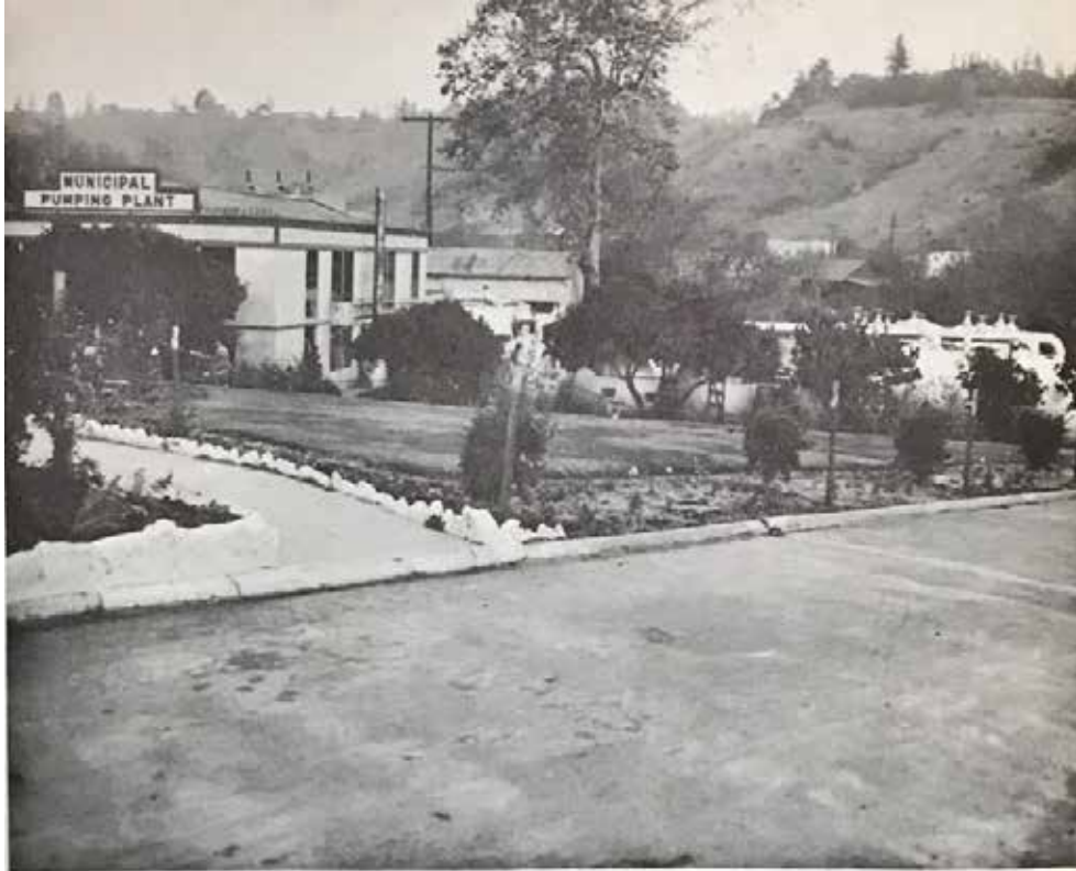
SANTA CRUZ MUNICIPAL PUMPING PLANT. Building houses low and high lift pumps and engine-driven generators. Pressure type filters are at right of building.
