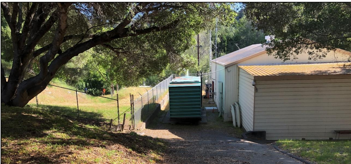
Exhibit 18. Rear of Coast Pump Station showing view looking northeast (IMG_0162).
