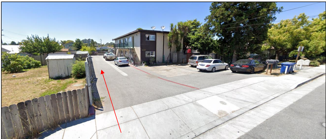
Exhibit 8. Beltz 8 access driveway off 38th Avenue showing point of entry (red arrow), view looking northwest (Google Earth 2020).
