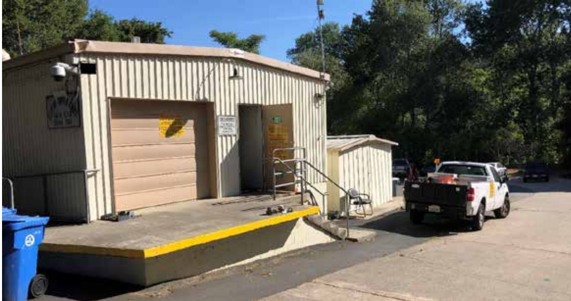
Exhibit 3. Meter Shop, southeast (main) elevation, view looking north (IMG_0181).
