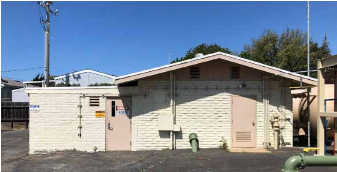
Exhibit 1. Control Building, east elevation, view looking west (IMG_0217).
