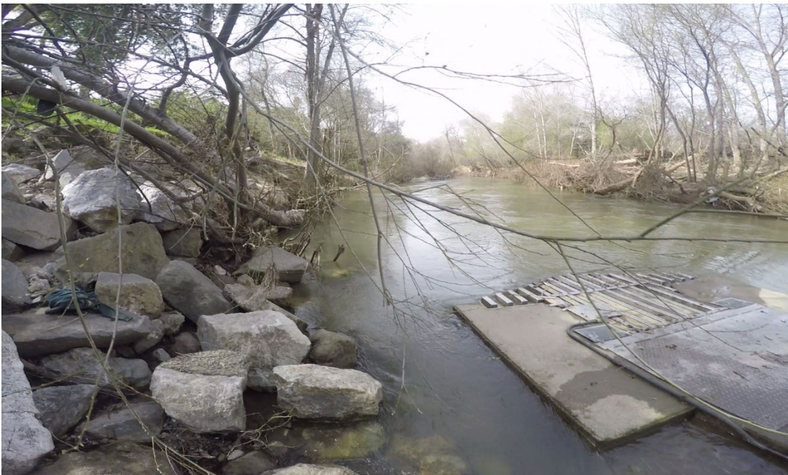
TAIT DIVERSION FACILITY- LOOKING UPSTREAM
