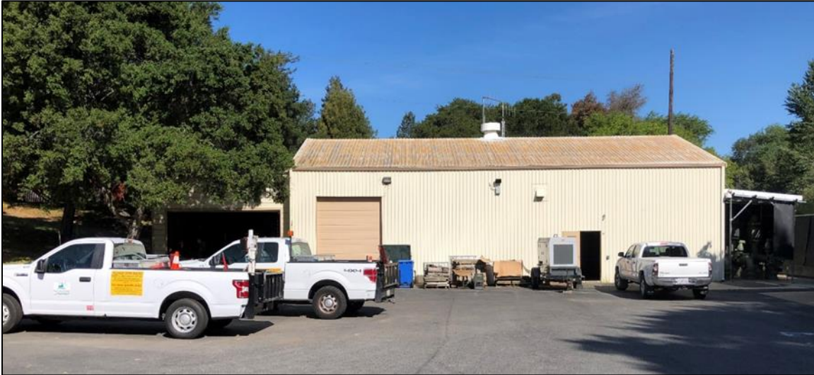
Exhibit 17. The Coast Pump Station, southeast (main) elevation view looking northwest (IMG_0185).
