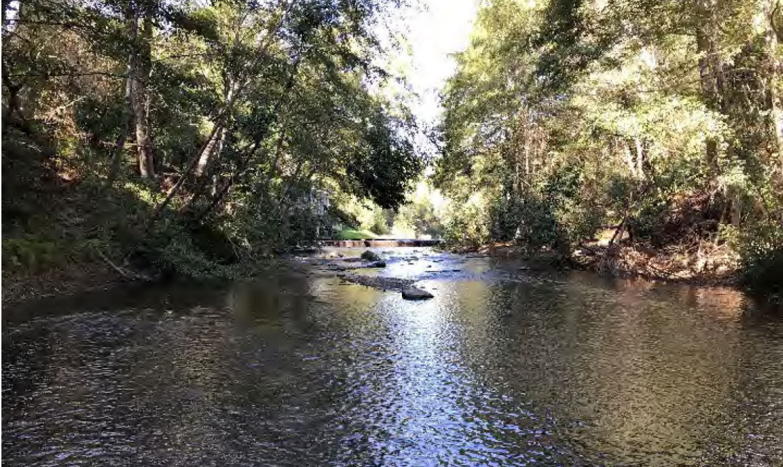
FELTON DIVERSION FACILITY- LOOKING DOWNSTREAM
