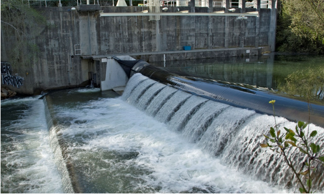
FELTON DIVERSION FACILITY
