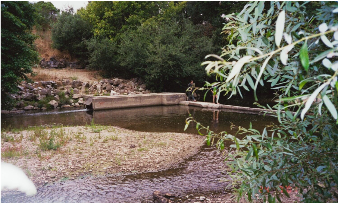
TAIT DIVERSION DAM JANUARY 2019
