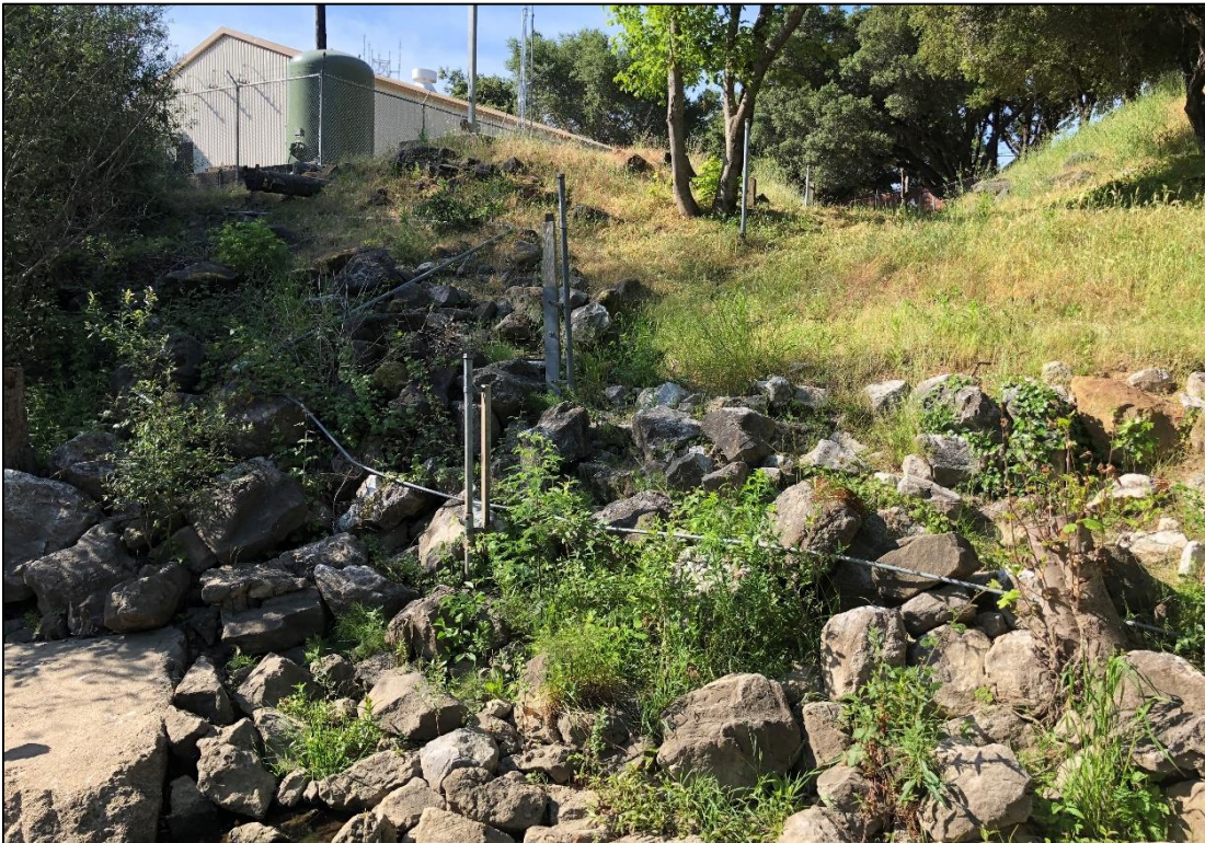
Exhibit 16. Path down from Coast Pump Station (pictured) to Tait Diversion, view looking south (IMG_0162).
