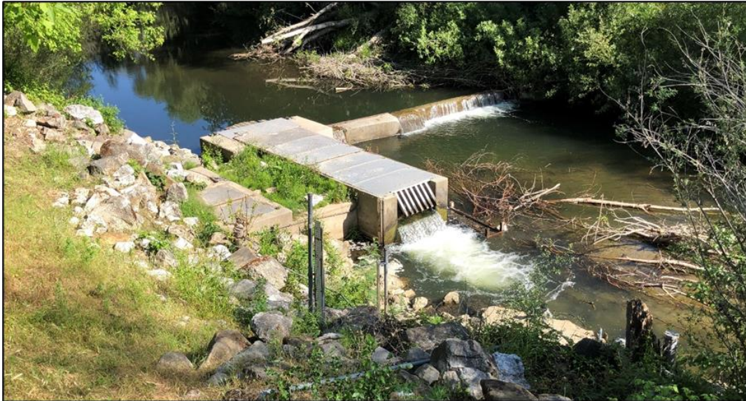
Exhibit 21. Tait Diversion, overview showing the 1983 intake in the foreground and the remaining section of the original concrete diversion dam stretching across the San Lorenzo, view looking north (IMG_0175).
