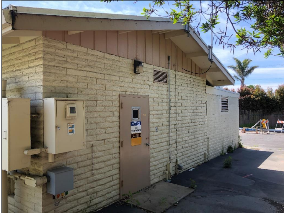
Exhibit 10. Control Building, west elevation, view looking southeast (IMG_0222).
