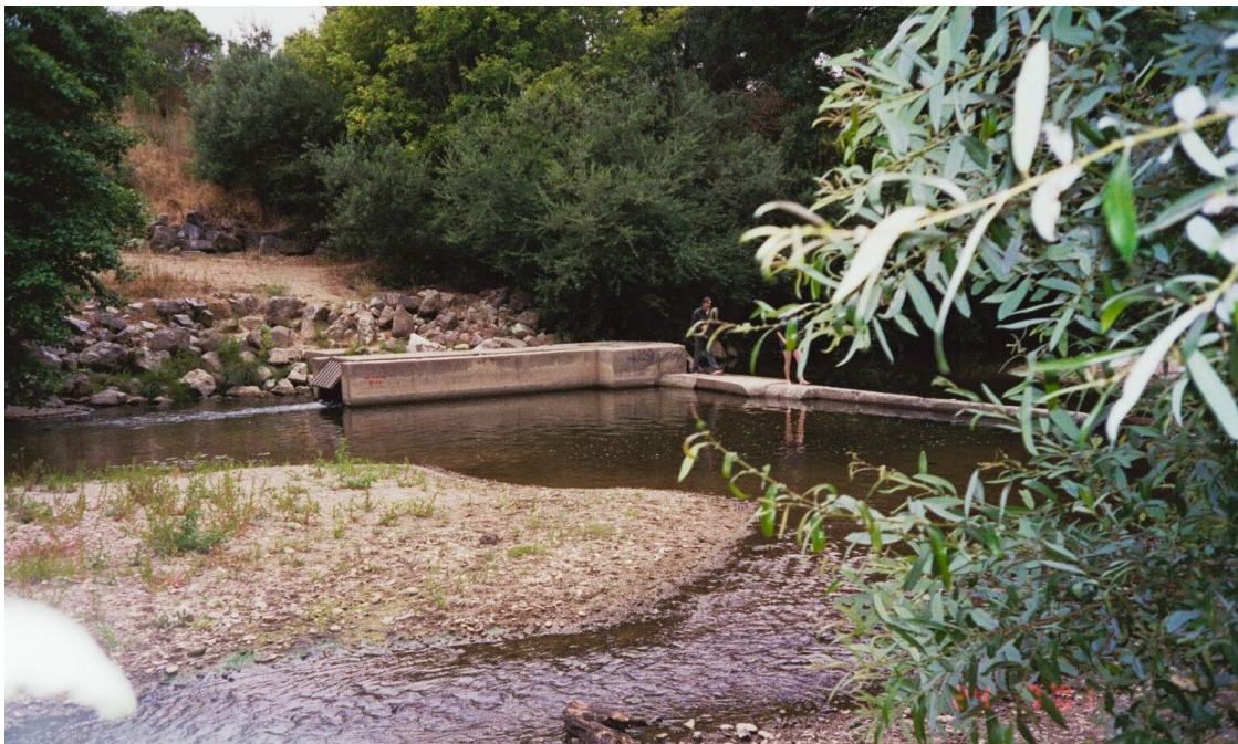
TAIT DIVERSION DAM JANUARY 2019
