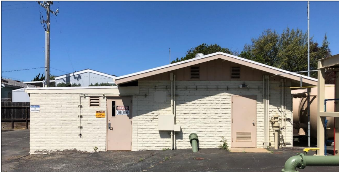
Exhibit 9. Control Building, east elevation, view looking west (IMG_0217).
