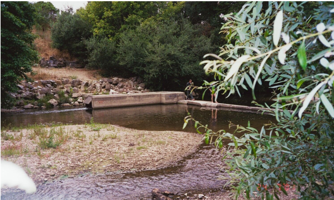
TAIT DIVERSION DAM JANUARY 2019
