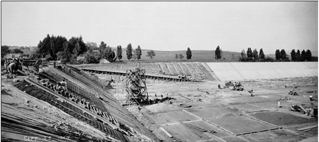
Exhibit 3. Construction of the Bay Street Reservoir in 1924 (SCPL 1924).
