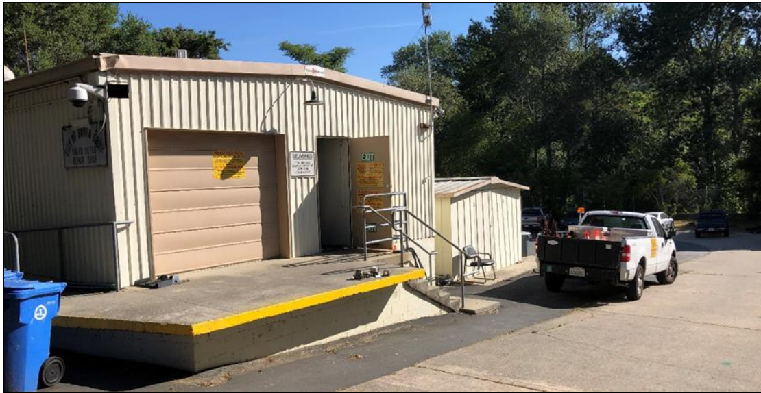
Exhibit 19. Meter Shop, southeast (main) elevation, view looking north (IMG_0181).
