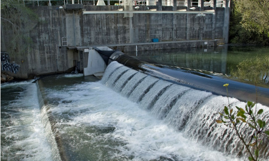
FELTON DIVERSION FACILITY
