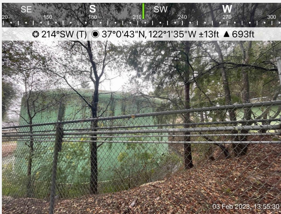
Photo Number 6. Pasatiempo tank site.
