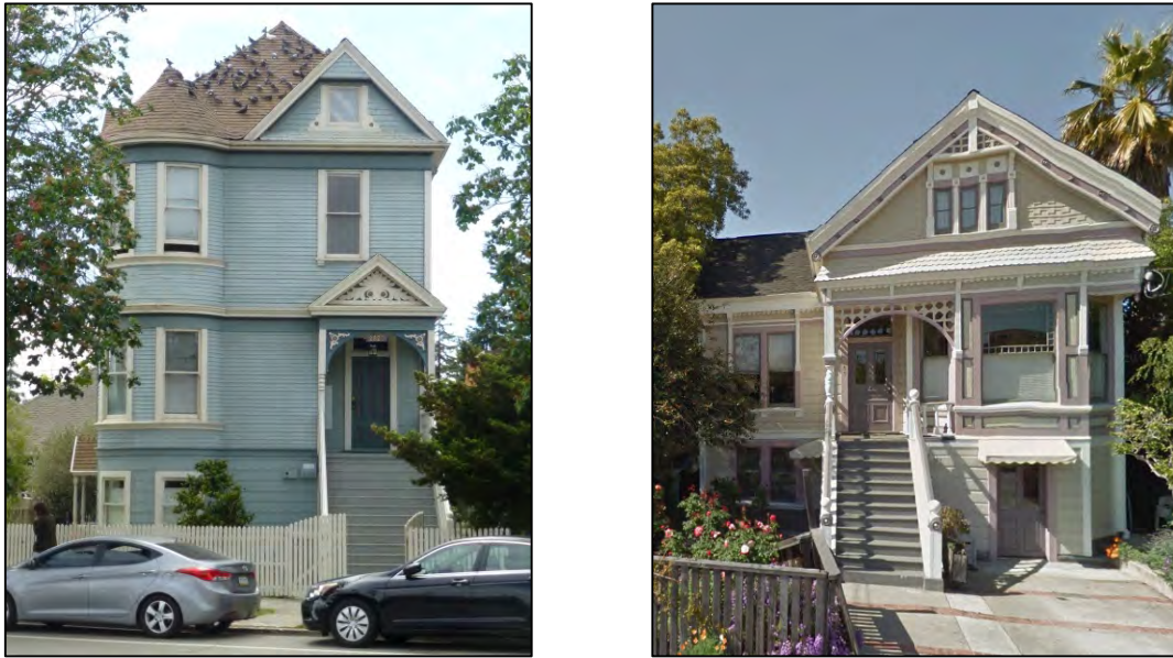
Figure 8. Nineteenth century Queen Anne-style residences at 2820 Adeline Street (left) and 2005 Stuart Street.
