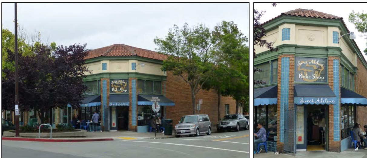
Figure 14. 1920 Spanish Colonial Revival style commercial building at 3350 Adeline Street.
