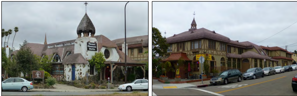
Figure 12. Storybook/Tudor Revival style buildings at 3031-3051 Adeline Street, built in 1922.
