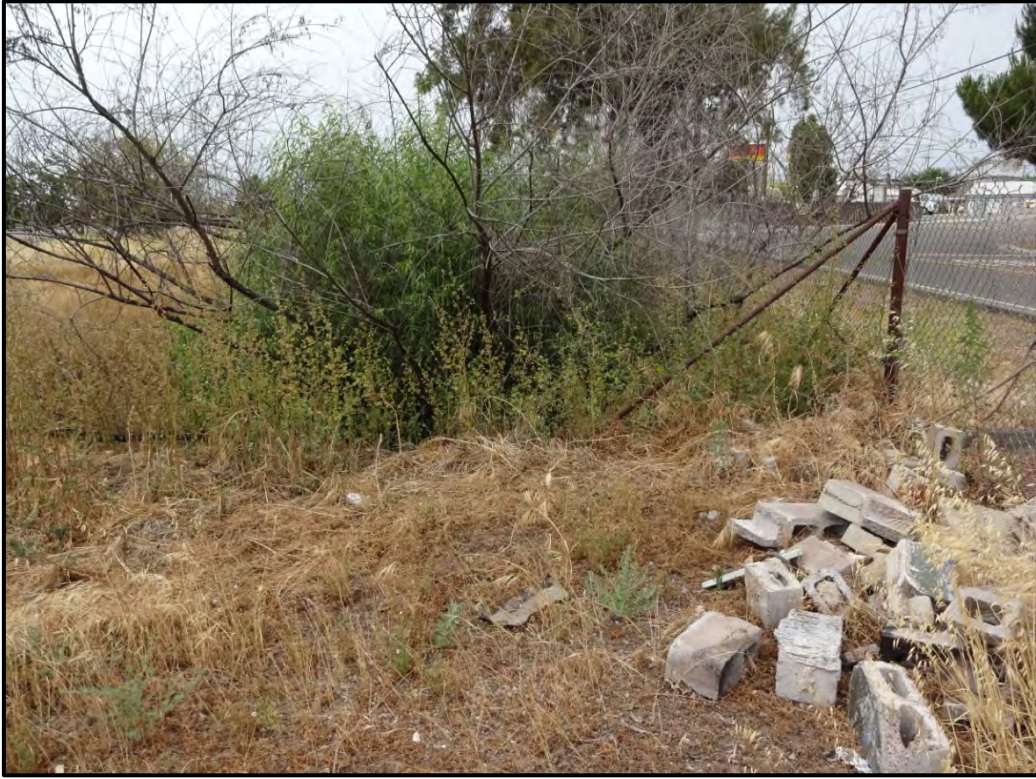
Old detention basin along Nunes Road, looking west; 06/10/15. This small basin is in the vicinity of the old foundations and was likely constructed when the site was previously developed.
