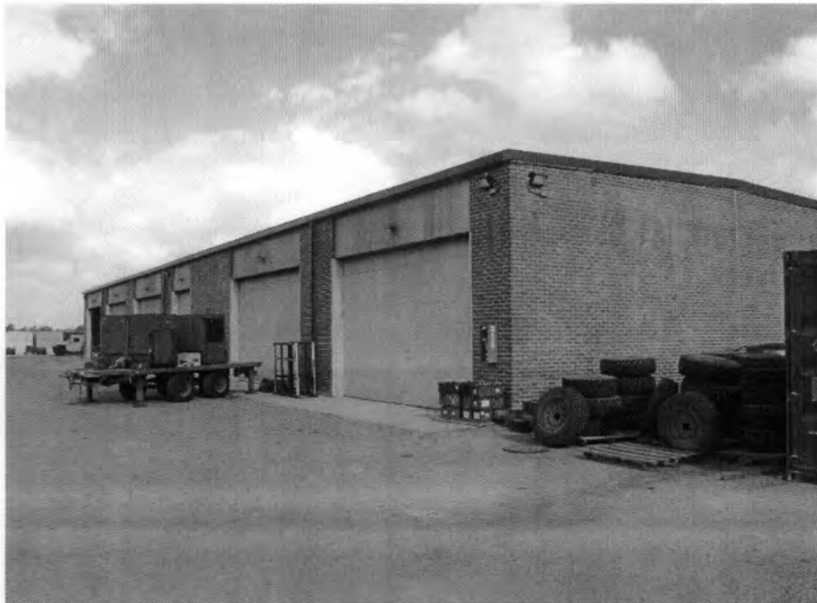
View northwest of south elevation of maintenance shop, 2/15/2006, OCo-TS-05-5037-005.jpg
