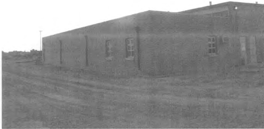
View southeast of north elevation of maintenance shop, 2/15/2006, OCo-TS-05-5037-007.jpg
