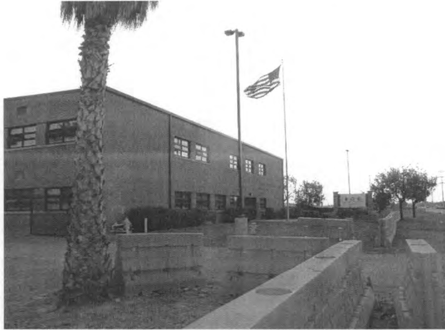
View east of south elevation, 2/15/2006, OCo-TS-05-5037-011.jpg
