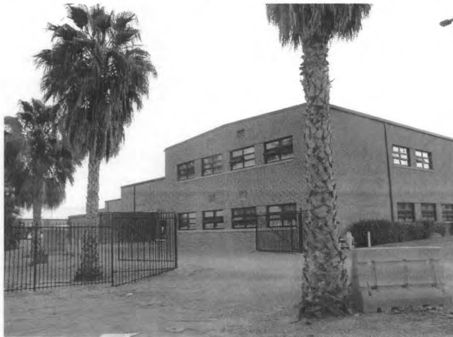
View east of west elevation, 2/15/2006, OCo-TS-05-5037-010.jpg
