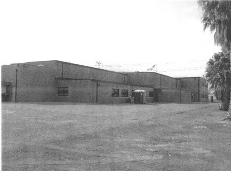
View south of west elevation, 2/15/2006, OCo-TS-05-5037-009.jpg
