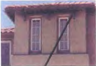
Exposed rafter tails
