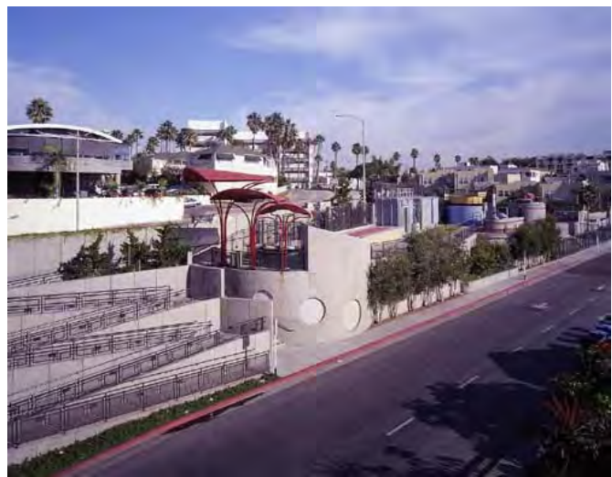
Dry weather runoff from the City's Pico-Kenter and Pier Storm Drains is ultimately treated at the SMURRF. The SMURRF is designed to treat and recycle up to 0.5 million gallons per day (MGD) of urban runoff.
