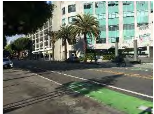
The building at 1333 2 nd Street located across from the eastern boundary of the Project site is a source of indoor illumination and glare due to the high reflectivity of its glassy façade.
