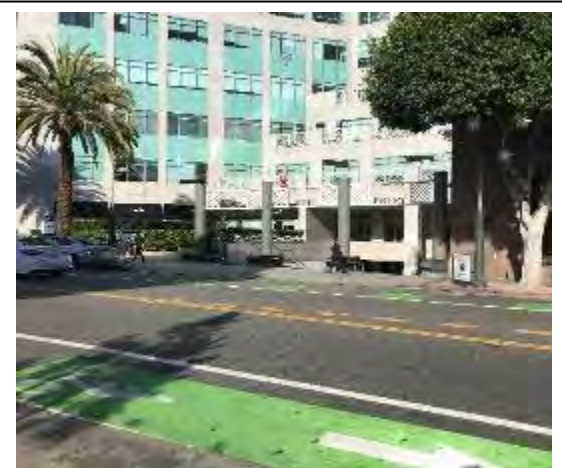
Green painted bicycle lanes are along 2 nd Street on either side of the paved width.
