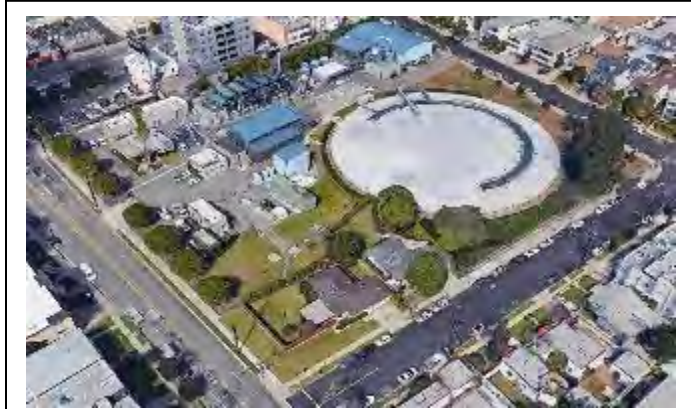
The Arcadia Water Treatment Plant is located near the intersection of Wilshire Boulevard and Bundy Street, and will be expanded to increase capacity to provide domestic water to the City of Santa Monica.
