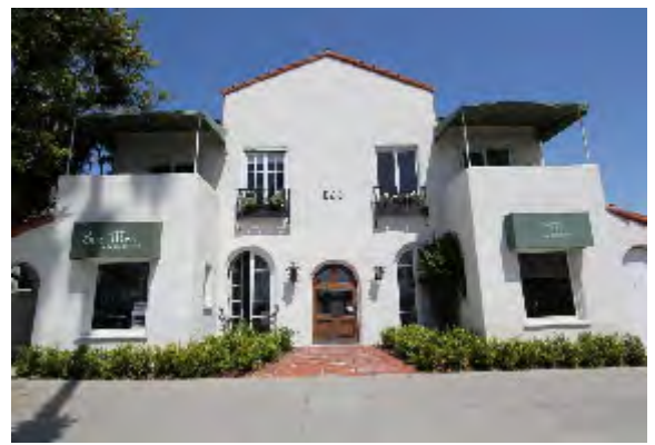
The Spanish Colonial Revival Landmark building at 1337 Ocean Avenue represents the expansion of commercial development along the residential-dominated Ocean Avenue in the early 20 th century.
