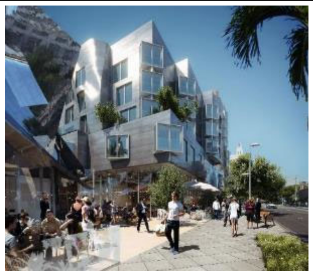
Ground floor commercial spaces with retail windows and outdoor dining areas in the Santa Monica Boulevard Building would activate the Project site along Santa Monica Boulevard.
