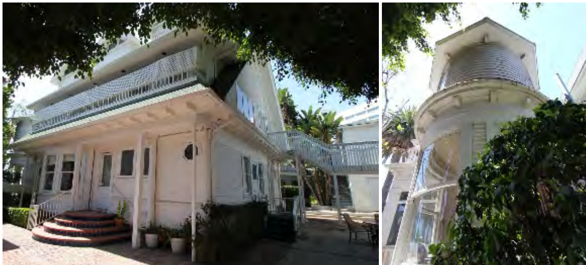
Left: Queen Anne Landmark, south elevation, view northwest. Right: Queen Anne Landmark tower, south elevation, view north.
