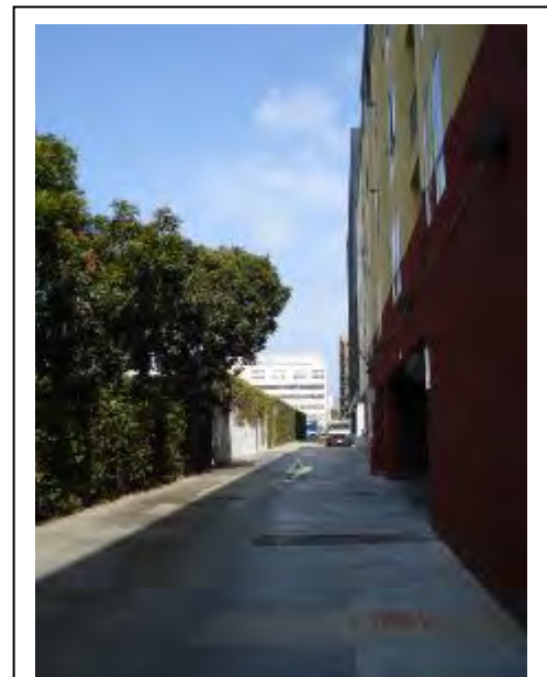
The residential buildings located across 1 st Court to the north and east of the Project site would experience increased periods of shade from the proposed Project, particularly during winter months.
