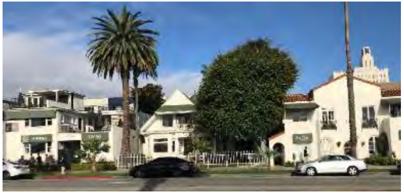
The three commercial buildings along Ocean Avenue within the Project site (1327, 1333, and 1337 Ocean Avenue) are all painted white and provide visual interest via windows, setbacks, and colored trim.
