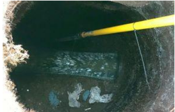
Manhole Before Install
