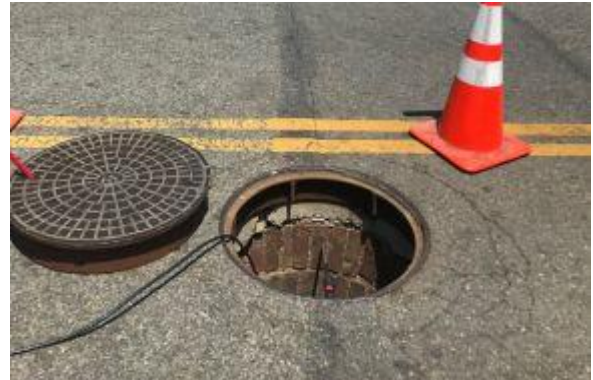
Manhole Before Install
