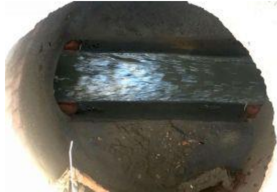
Manhole Before Install
