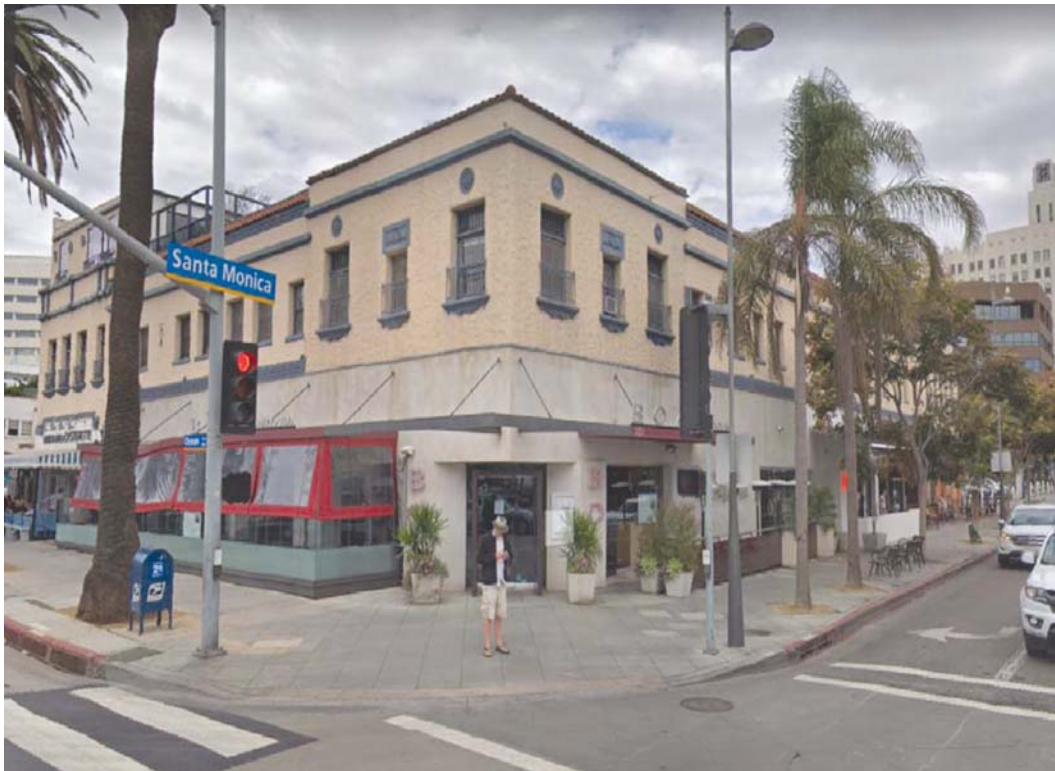
1) View of the Site looking north.
