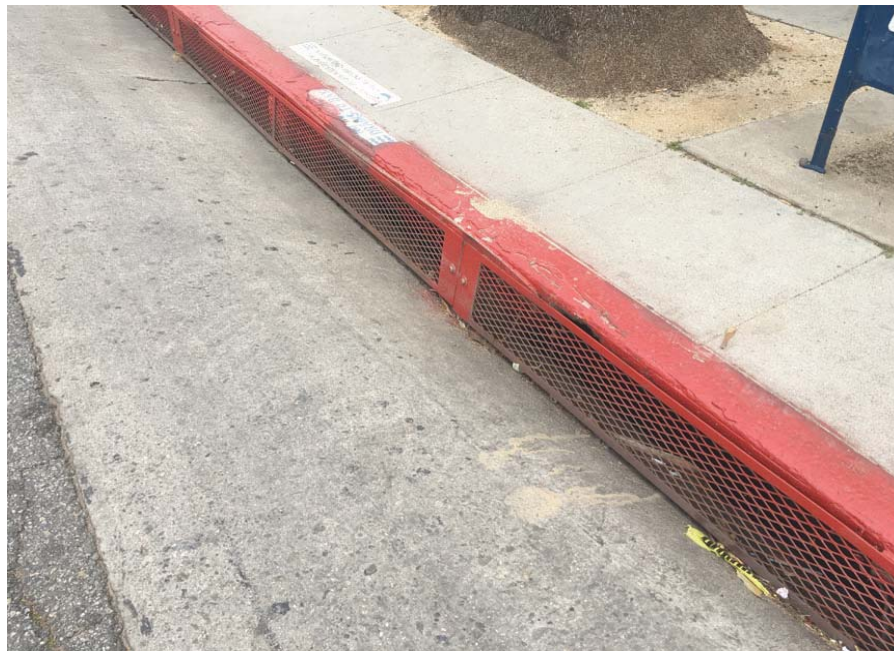
2) View of a storm drain located along Ocean Avenue.
