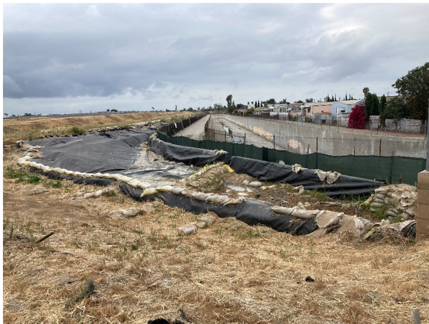
Site Photograph 2 - View of dry retention/detention basin and Torrance Lateral in the background. Photo taken facing south.
