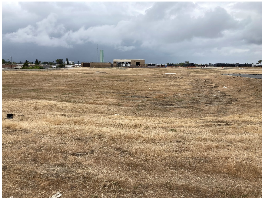
Site Photograph 3 – View of ruderal habitat on site. Gas burning facility and water treatment plant that is under construction in the background. Photo taken facing west.
