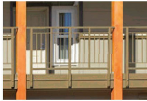
METAL BALCONY RAILING
