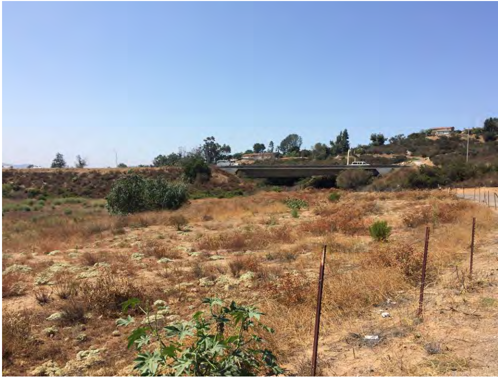
Photograph 7 – View looking towards the west-southwest, from the central region of the subject property; along N. Nutmeg Street.
