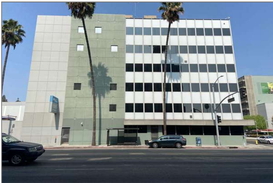
ABOVE: Photo E: View north to six-story medical office building on Site 3 (1505 North Edgemont Street)
