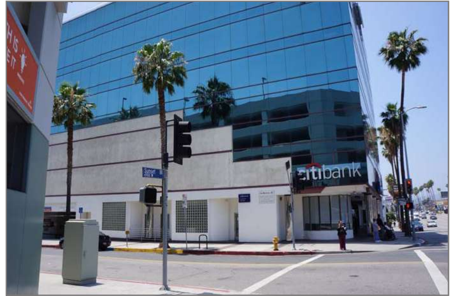
ABOVE: Photo 11: View west from Sunset Boulevard to Commercial Office Building
