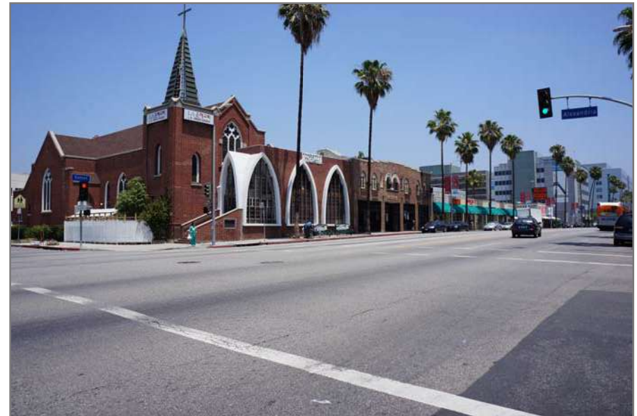
BELOW: Photo 12: View northeast from Sunset Boulevard to brick Church Facility
