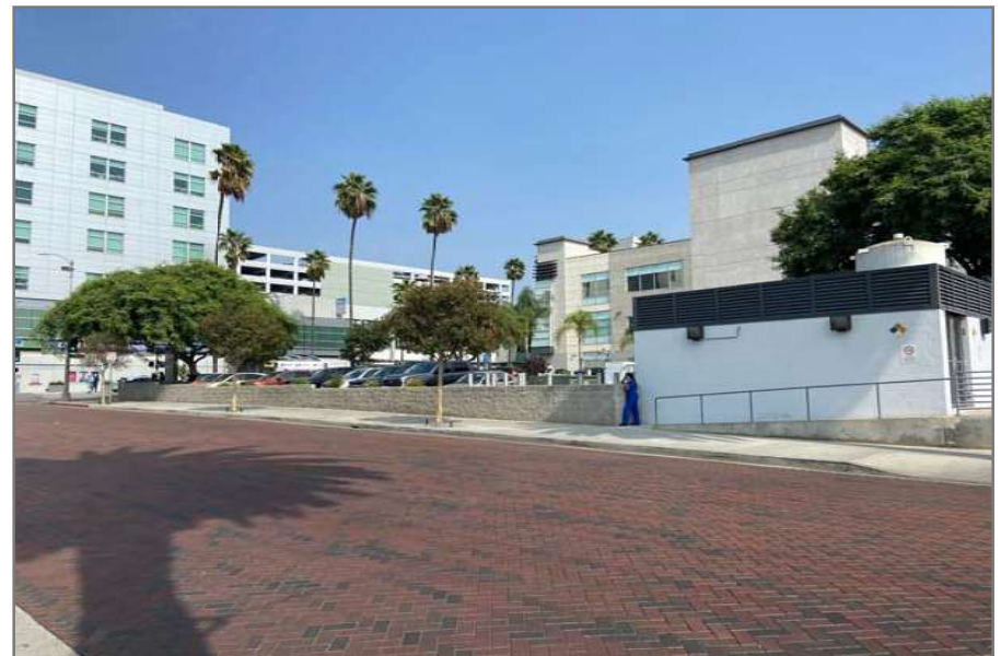
BELOW: Photo D: View northeast from L Ron Hubbard Way to parking lot and hospital utility building on Site 2 (4760 Sunset Blvd)
