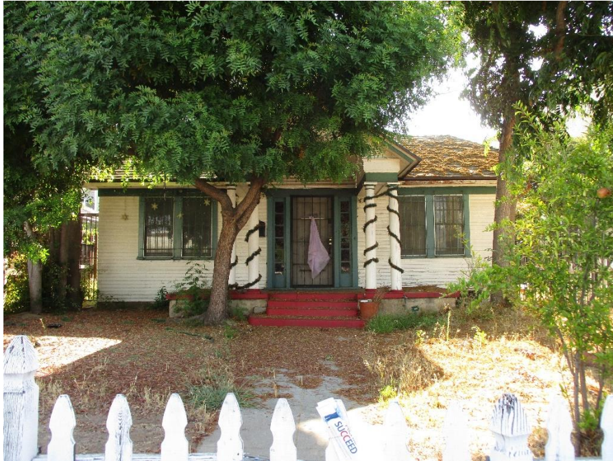
Figure 15. Overview of the Main (west) Elevation of 1328 North New Hampshire Avenue, Looking East, 8/15/2018 (IMG_0761)
