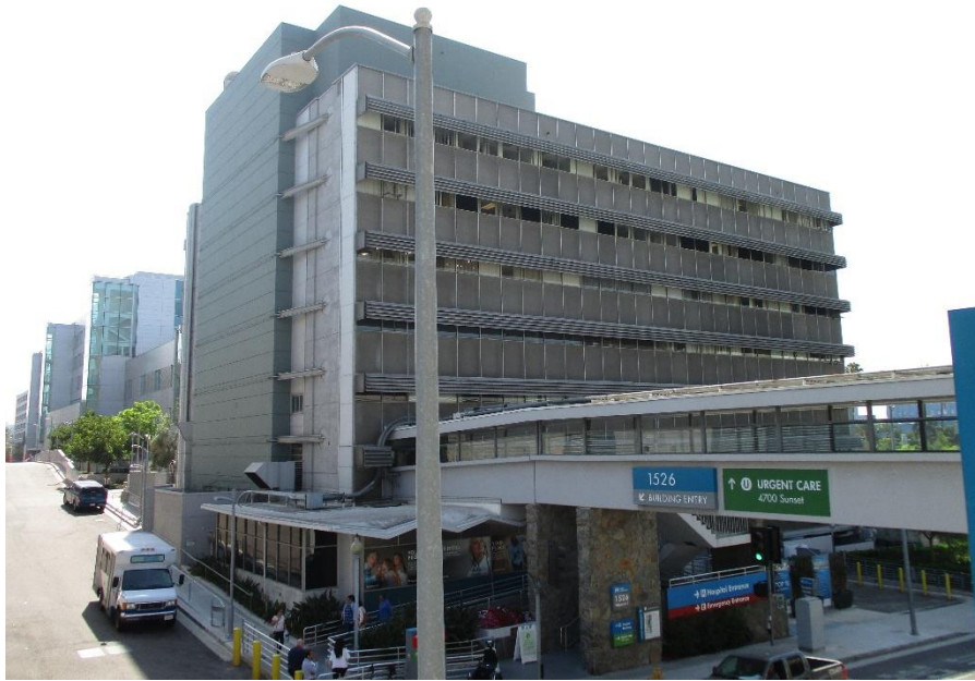
Figure 9. Overview of the North Elevation (left) and West/Main Elevation (right) of 1526 North Edgemont Street, Looking Southeast, 8/15/2018 (IMG_0837)
