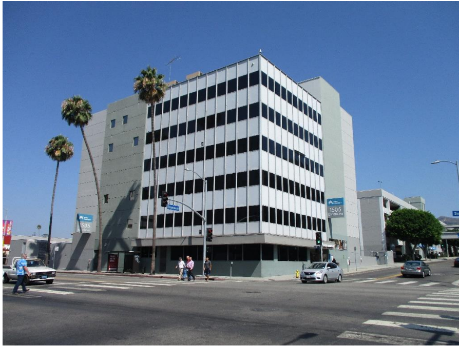
Figure 11. Overview of the South Elevation (left) and East (Main) Elevation (right) of 1505 North Edgemont Street, Looking Northwest, 8/15/2018 (IMG_0865)
