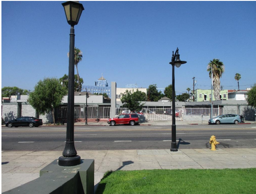
Figure 13. Overview of the East Elevation of the Three-Building Complex at 1321 North Vermont Avenue, Looking West, 8/15/2018 (IMG_0813)
