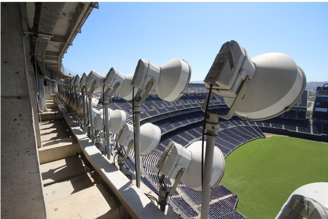
Figure 3-35: View from the continuous lighting ring that wraps the original U-shaped portion of the stadium.
