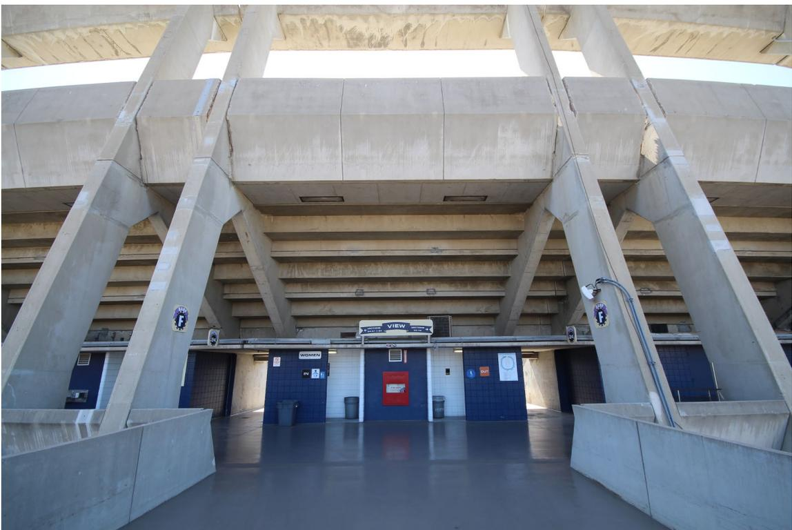
Figure 3-29: The view level at the top of ramp F. Note the original paired structural piers on each side.
