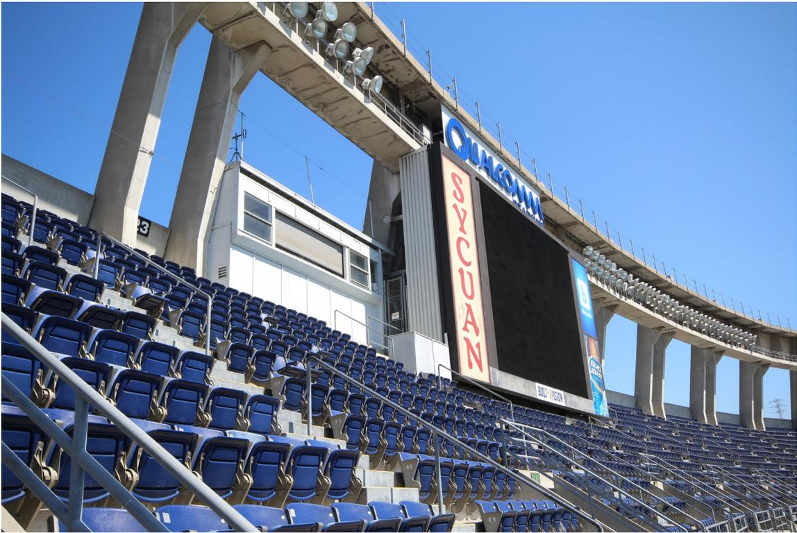
Figure 3-34: View of the west scoreboard/screen and non-original wood security booth. The safety rails at the top of the light ring were added recently.
