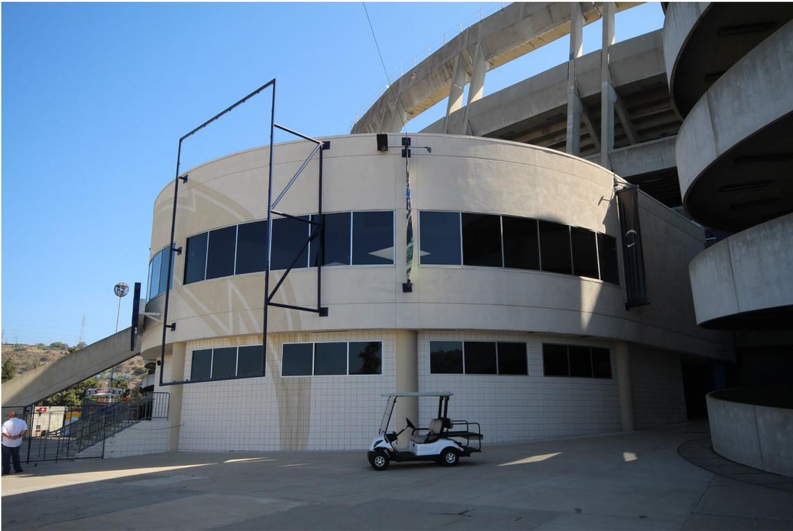
Figure 3-22: One of four 1997 curved additions added in the spaces between the original ramps and escalators.
