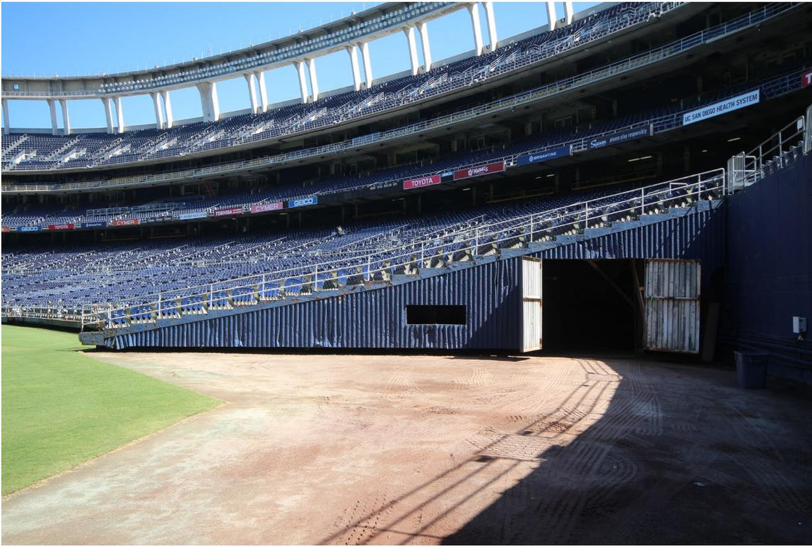
Figure 3-37: View from the field looking at the end of an original metal-clad movable seating section.
