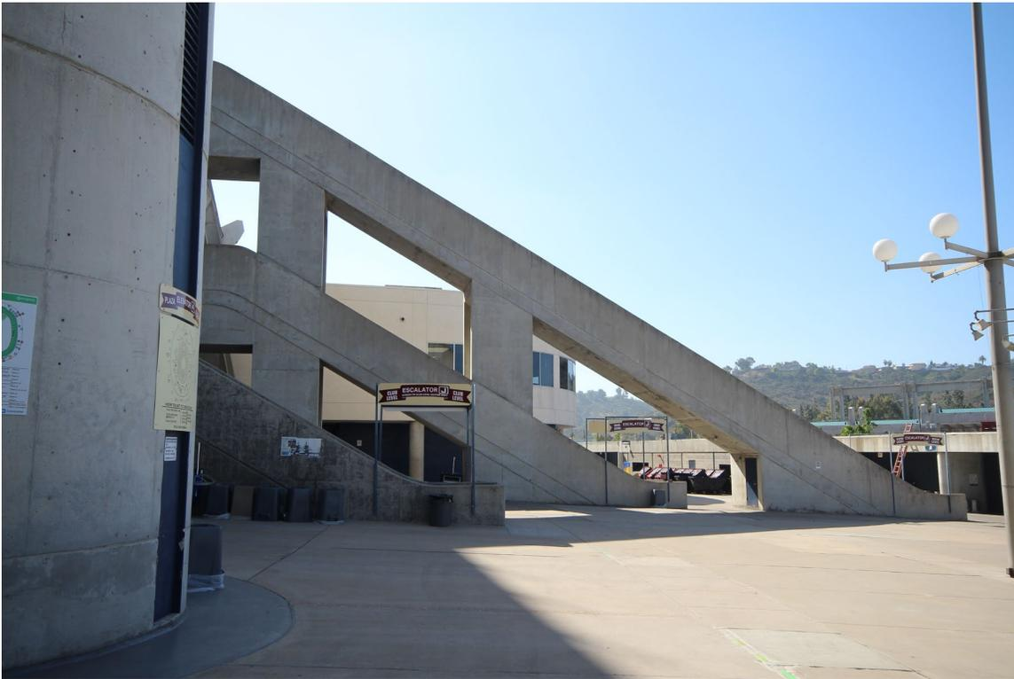
Figure 3-15: Original stacked escalators serving the loge and view levels. The smaller escalator in the foreground was added in 1997 to serve the club level.
