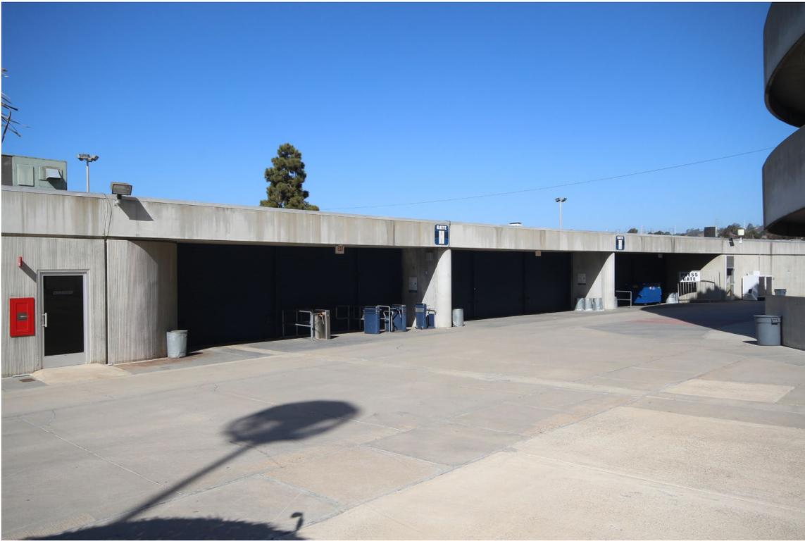
Figure 3-9: View of Gate H from the interior showing the original cast-concrete walls and steel roll-up gates.
