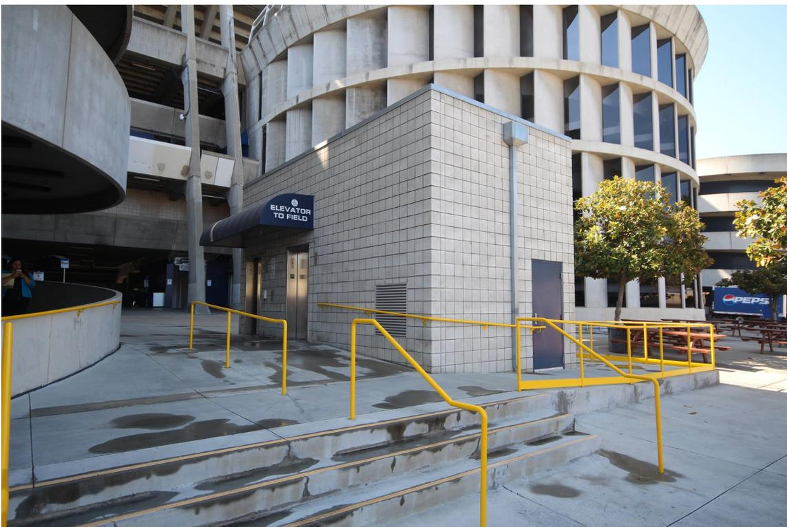
Figure 3-25: An elevator structure with ramps added after in 2002 to serve the disabled.
