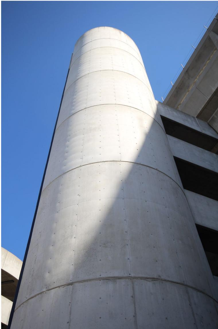
Figure 3-19: Close up of an elevator tower. Note the grid of concrete form tie holes and unpainted finish.
