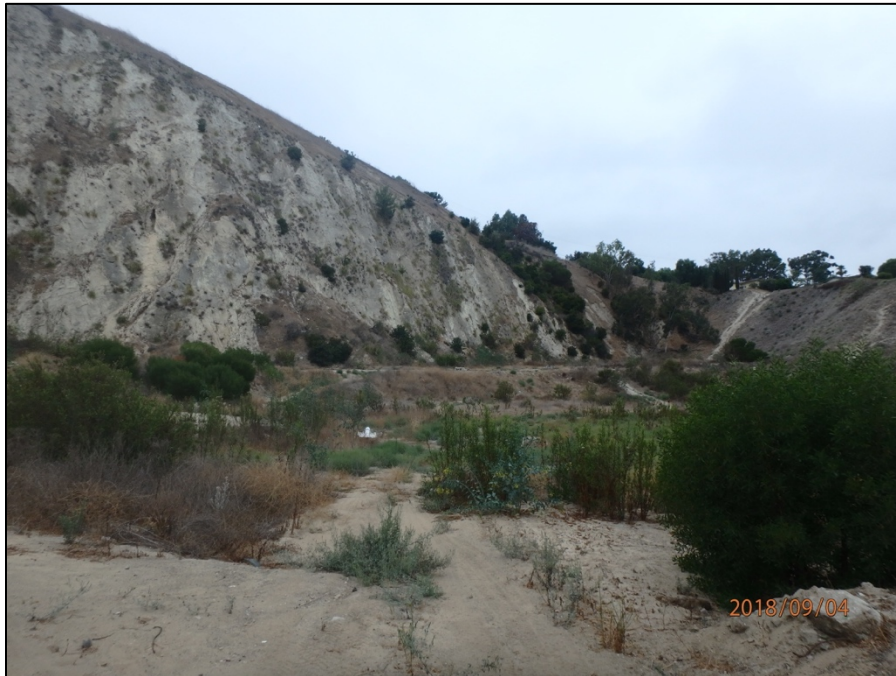
Figure 4. Overview of excavation cut. View west.
