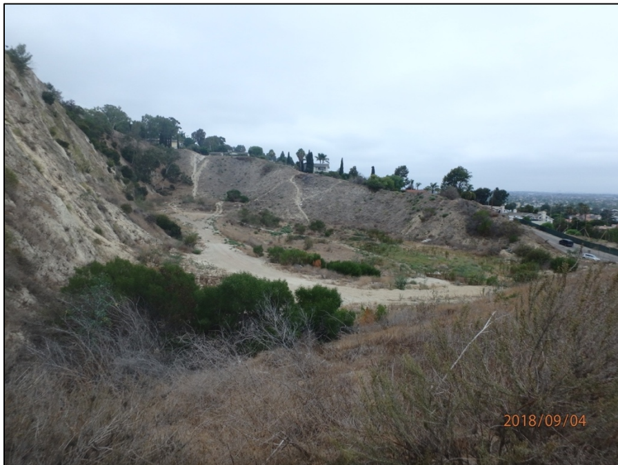
Figure 6. Project overview from southeastern portion. View west.
