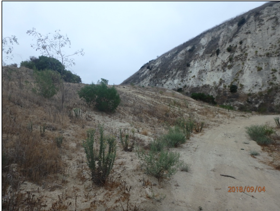
Figure 3. Overview of excavation cut. View south-southeast.
