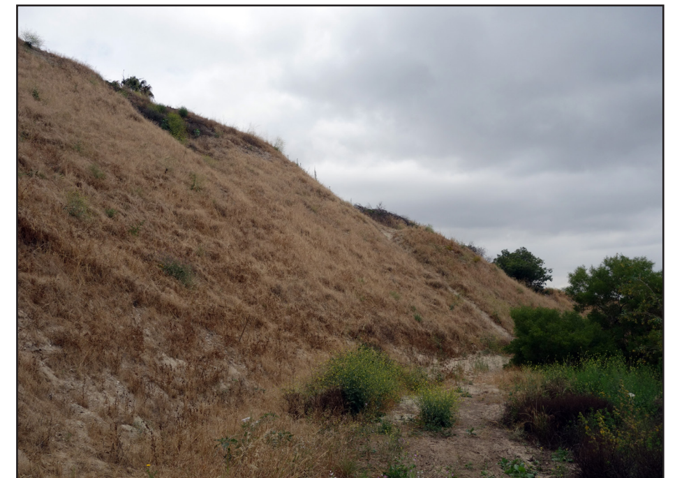
④ Side view of Slope 2 looking southeast from the northwest part of the development area.
