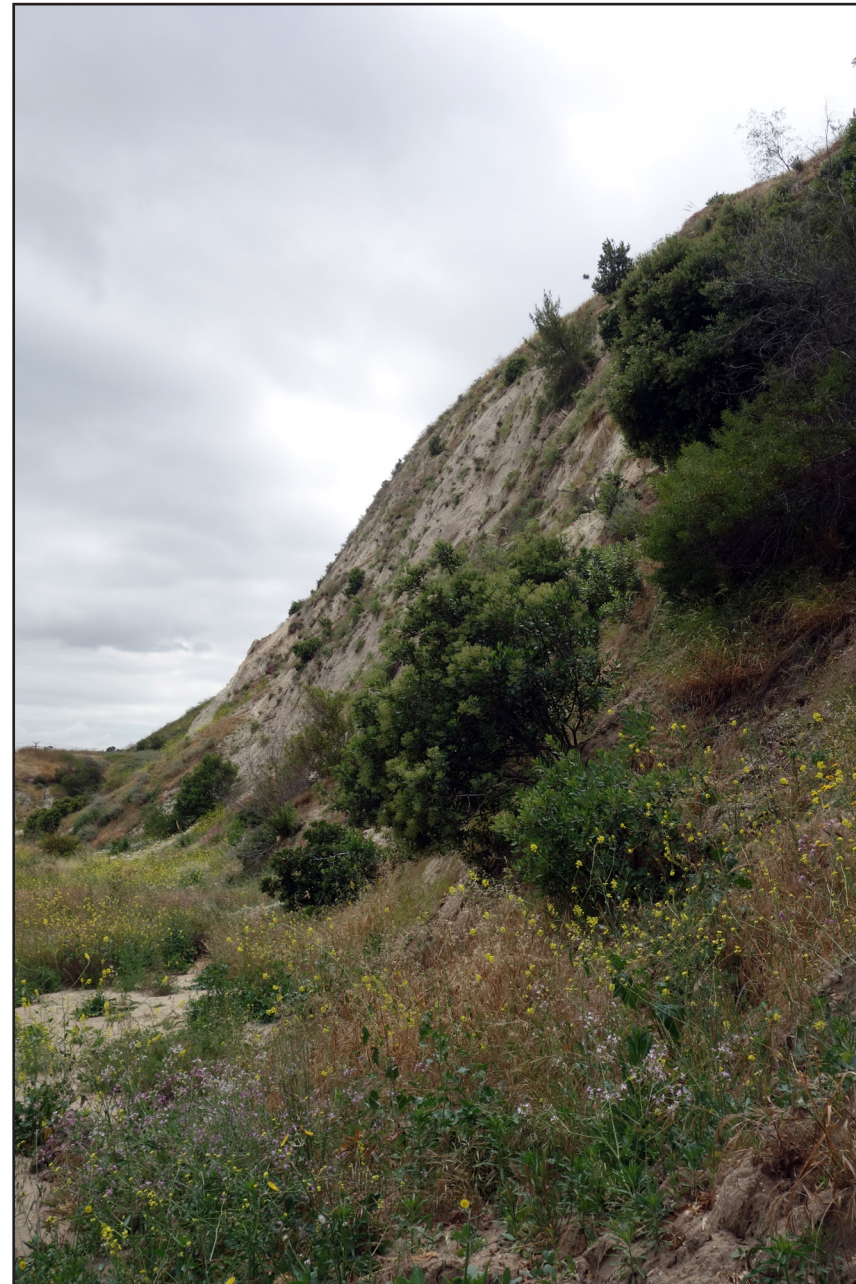
② Side view of Slope 3 looking southeast from the northwest part of the development area.
