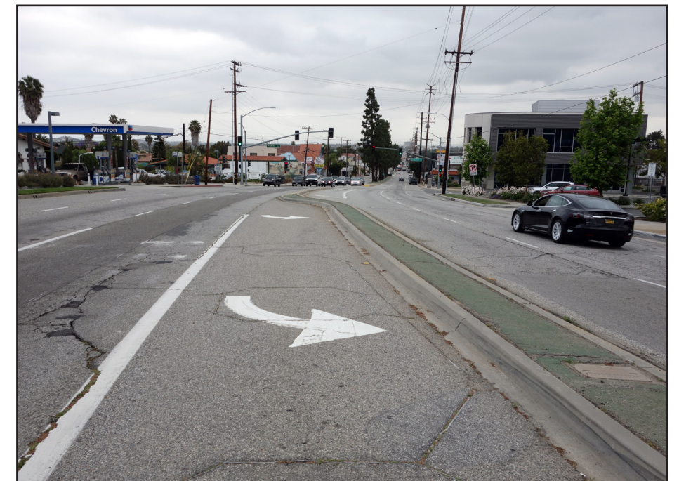
④ View looking north along Hawthorne northeast on the project site.
