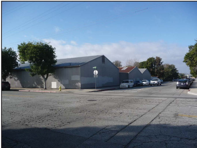
View 11: View looking southwest on the intersection of Date Avenue and Orange Avenue of the existing structures on the northeastern portion of the Project Site.
