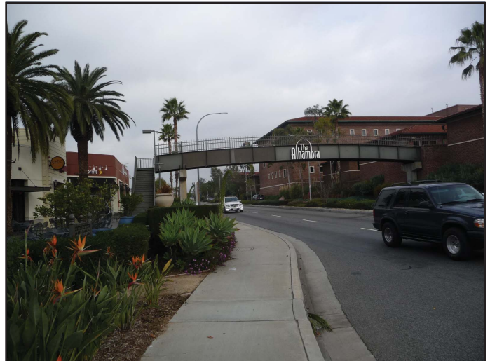
View 20: View looking northeast on Fremont Avenue of existing structure and pedestrian bridge adjacent to the southwestern portion of the Project Site.
