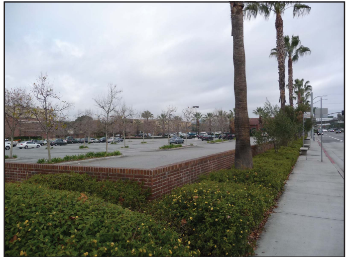
View 44: View looking northwest on Fremont Avenue of existing shopping center and mixed-use buildings adjacent to the southwestern portion of the Project Site.
