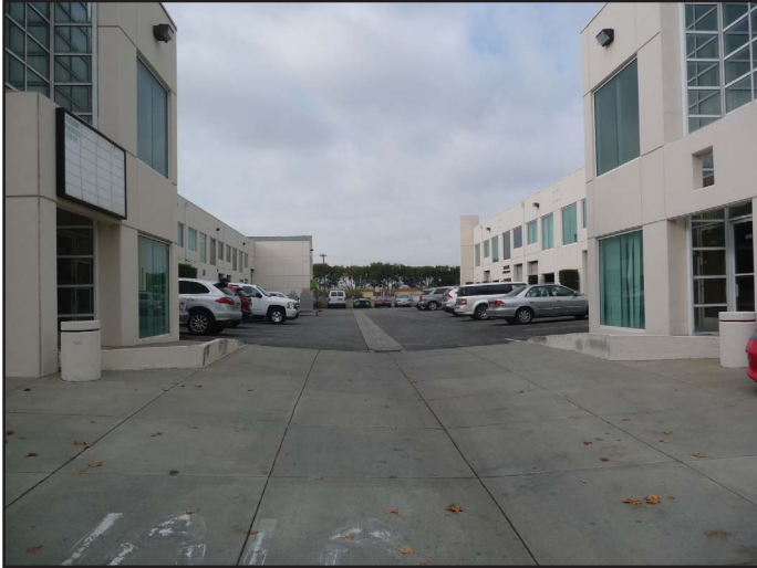
View 41: View looking west on Fremont Avenue of existing office buildings adjacent to the northwestern portion of the Project Site.
