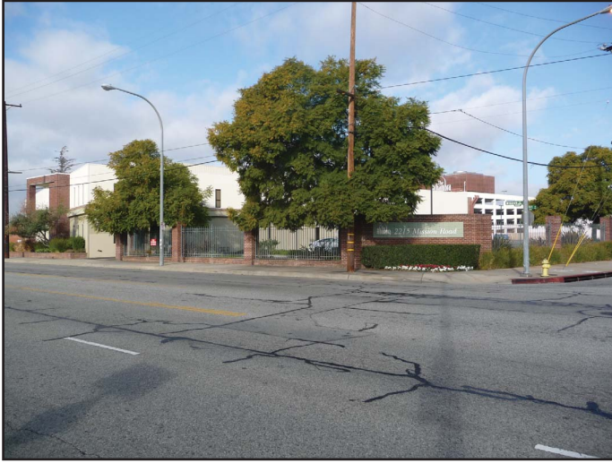
View 5: View looking northwest on the intersection of Mission Road and Date Avenue of the existing structures on the southeastern portion of the Project Site.
