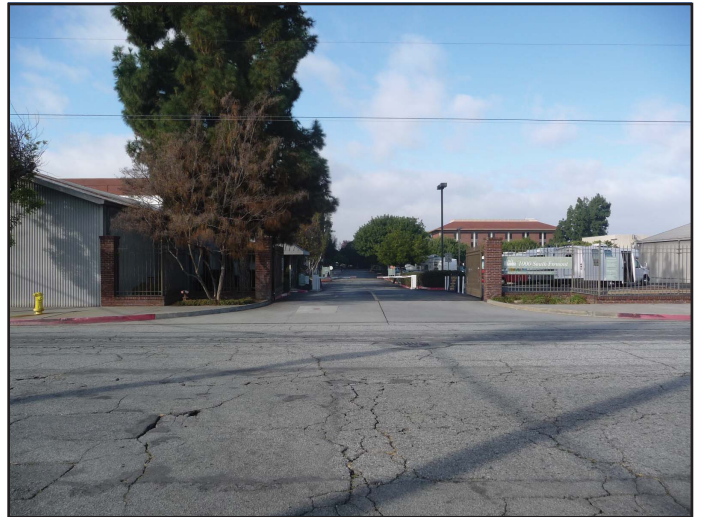
View 8: View looking west on Date Avenue of vehicle entryway and existing structures on the eastern portion of the Project Site.
