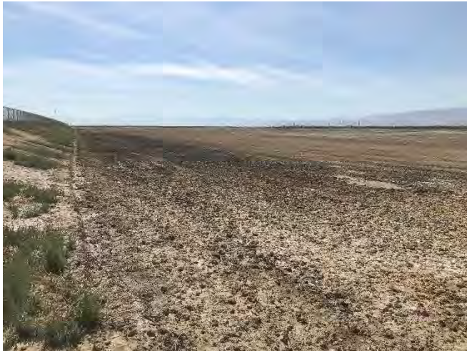
Photo 7. Looking east from the southwest corner of the plant.
