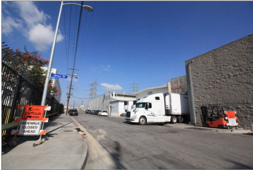
Northern section of the building's primary (west) elevation, view northeast
