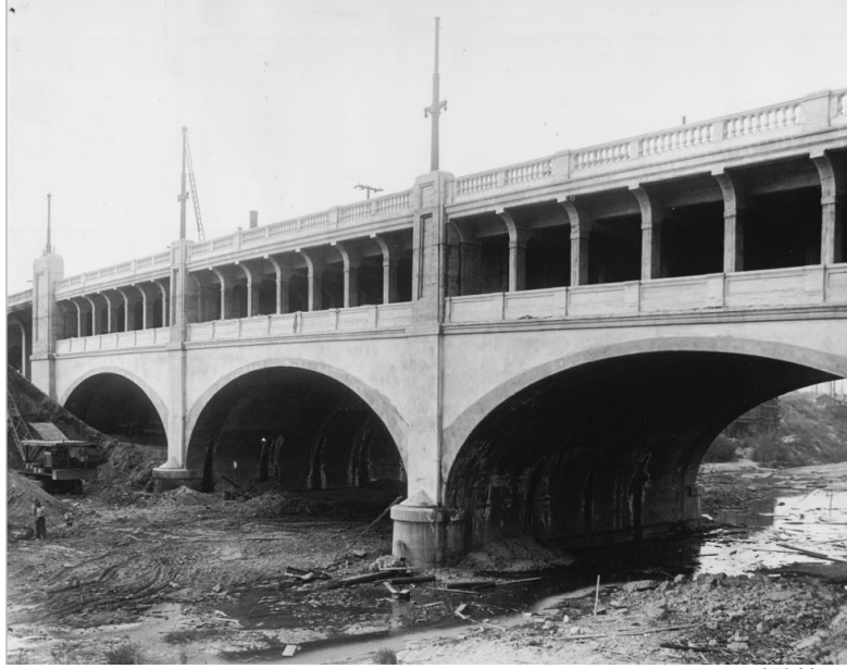
Figure 20 Construction of the second upper deck on the 7 th Street Bridge, 1927
