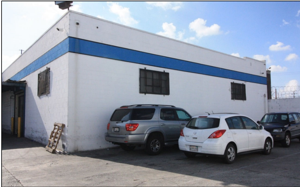
View of the building's projecting mass, north elevation, view south
