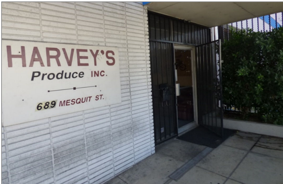
Closer view of the entryway on the primary (north) elevation, view south
