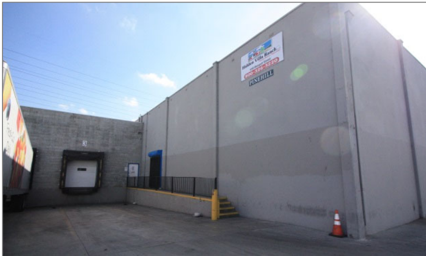
Tilt-up concrete addition constructed in 1985, view southeast
