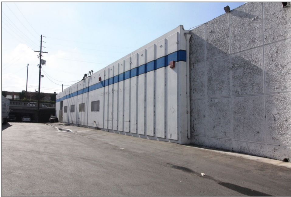
Secondary (east) elevation, view southwest
