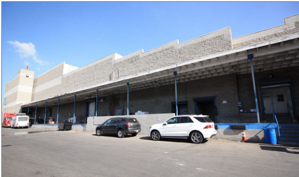
Primary (west) elevation, view of additional loading bays, view northeast
