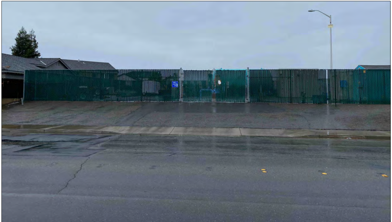
Figure 9. Photograph of the Project site at Well 10, looking north, showing the paved and fenced well pad and adjacent single-family homes.
