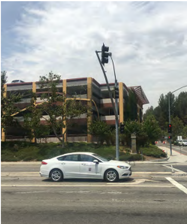
View of Parking Structure 1 (PS-1) from the southwestern corner of the McBean Parkway and Avenida Navarre intersection.
