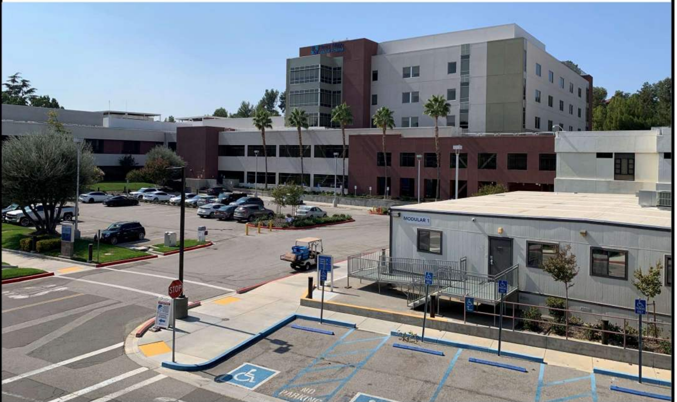
Existing conditions at Lot D and Lot I (2020).
