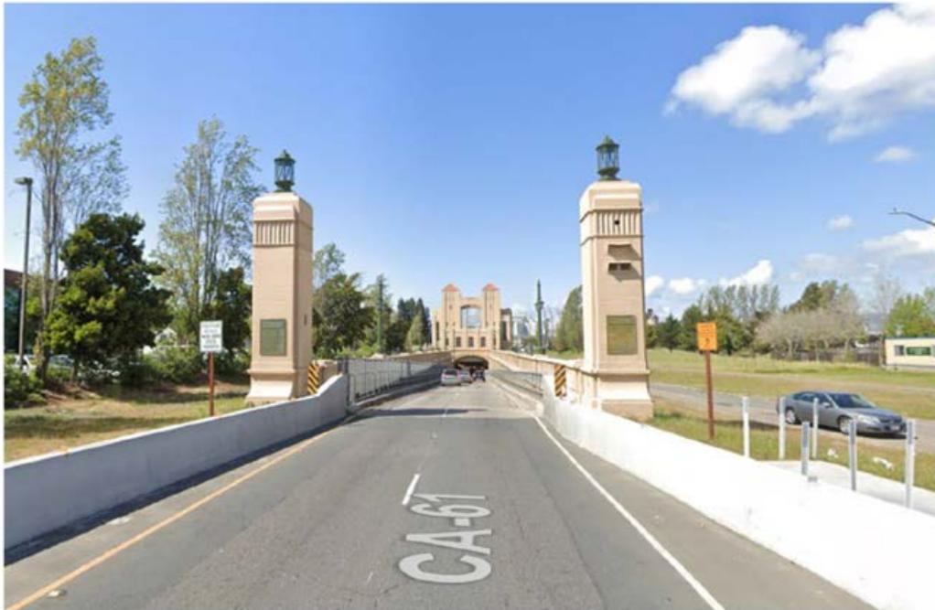
**Remnants of original pillars on Oakland side of tunnel, shortened to make way for freeway structure, View 1**
