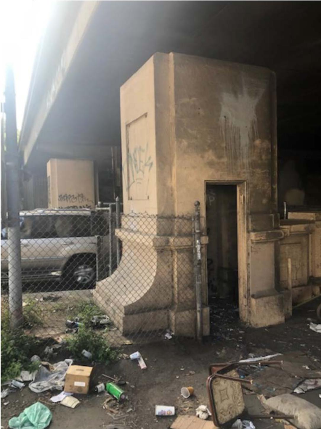
**Remnants of original pillars on Oakland side of tunnel, shortened to make way for freeway structure, View 2.**
