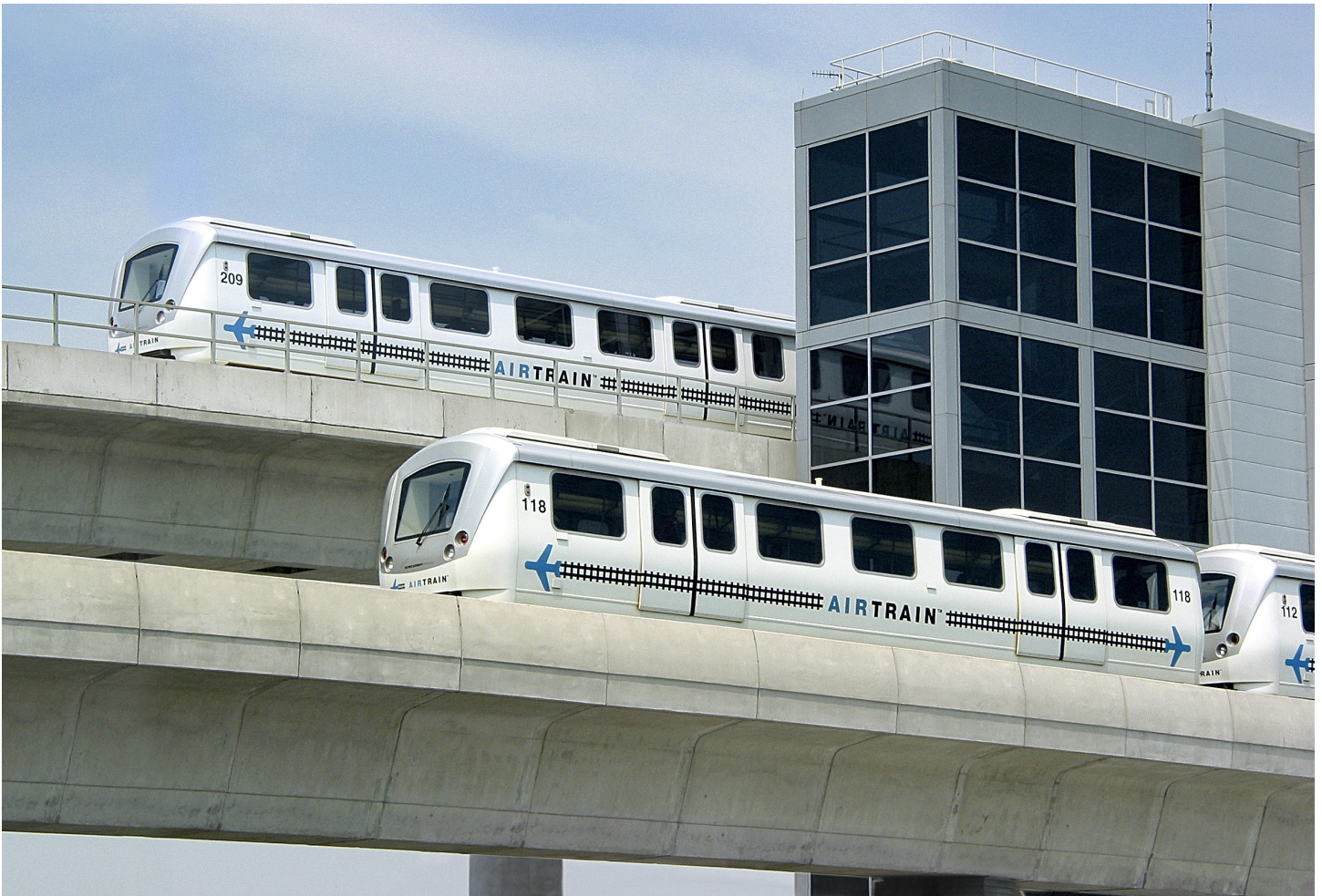
Figure 2.6-6: Large Steel Wheel-Rail APM Examples
