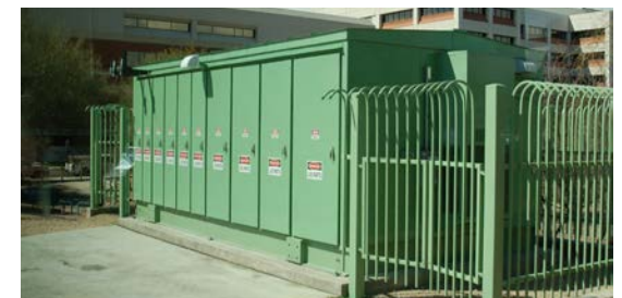
Figure 2.8-2 Example Traction Power Substation
