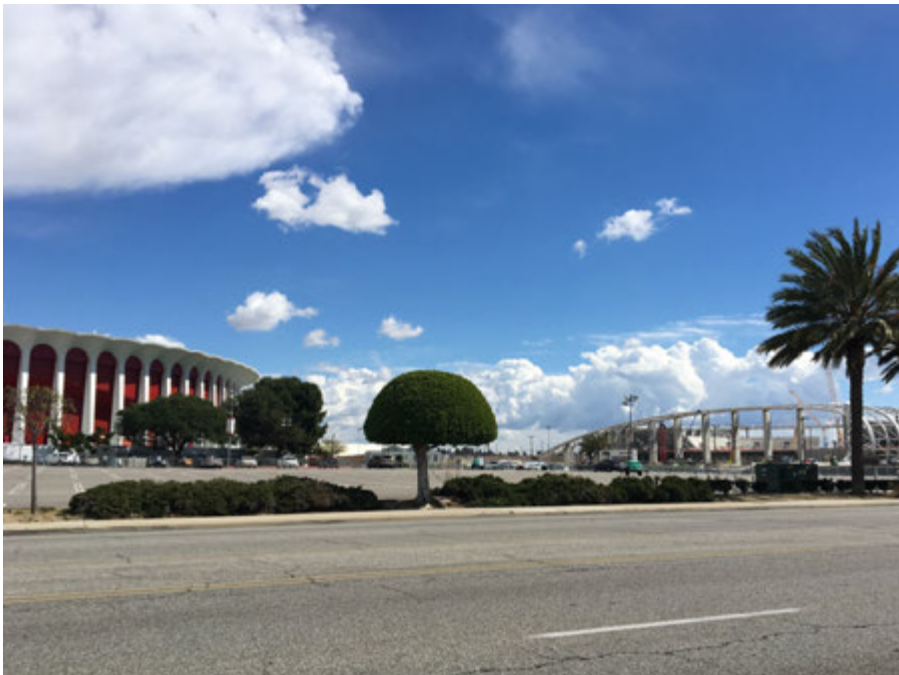
The Forum, 3900 W. Manchester Boulevard, with SoFi Stadium (Southeast view).
