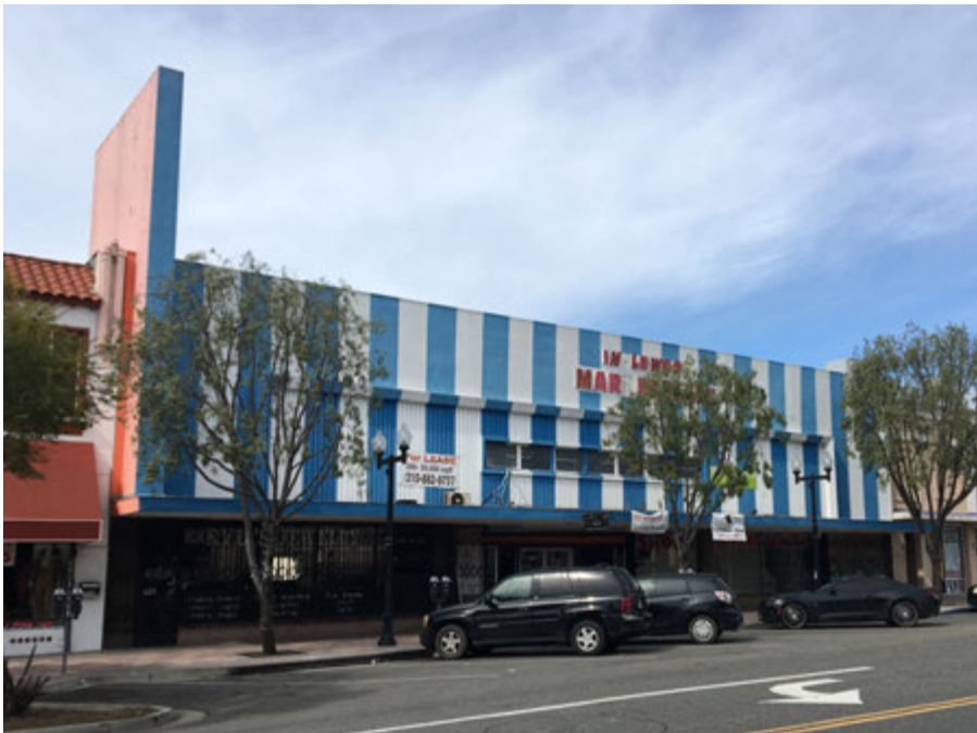
Former J.C. Penney, 129-139 S. Market Street ( Northwest view ).
