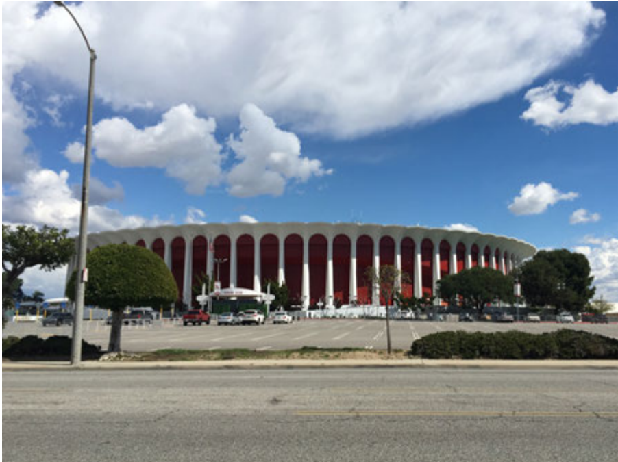
The Forum, 3900 W. Manchester Boulevard ( East view ).
