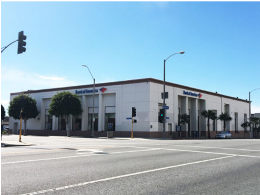
Bank of America, 320-330 E. Manchester Boulevard (Southwest view).
