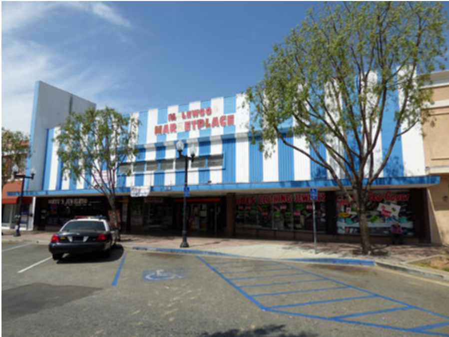
Former J.C. Penney, 129-139 S. Market Street, ( Southwest view ).
