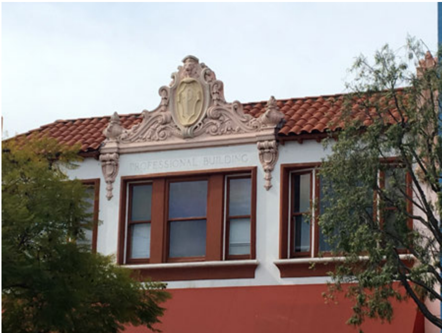
Professional Building, 149-155 S. Market Street/231-239 E. Manchester Boulevard (Southwest view, detail).
