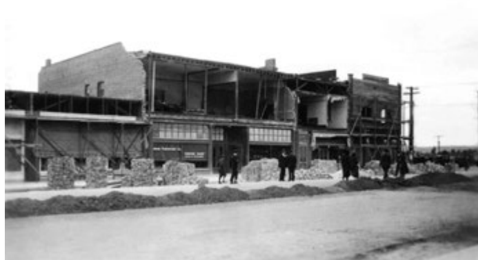
Damaged buildings from Inglewood Earthquake, June 21, 1920. ( California Historical Society Collection, USC )
