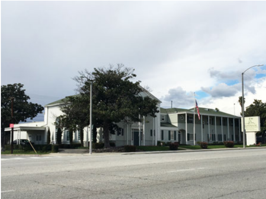
Lighthouse McCormick Mortuary, 619-635 S. Prairie Avenue ( Northwest view ).
