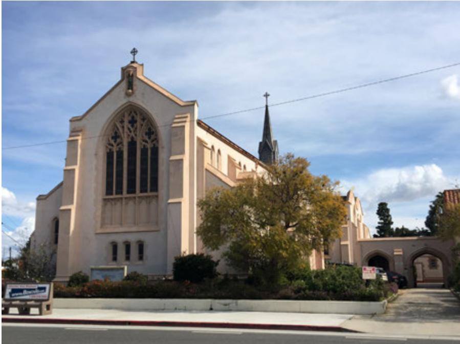
Holy Faith Episcopal Church, 260 N. Locust Street ( Northeast view ).
