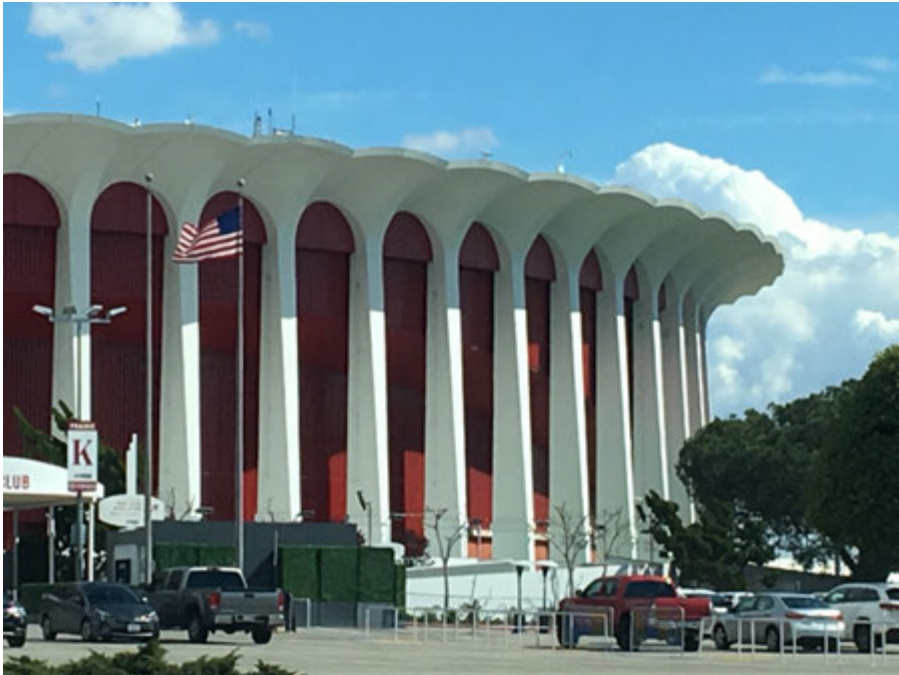
The Forum, 3900 W. Manchester Boulevard (East view, detail).
