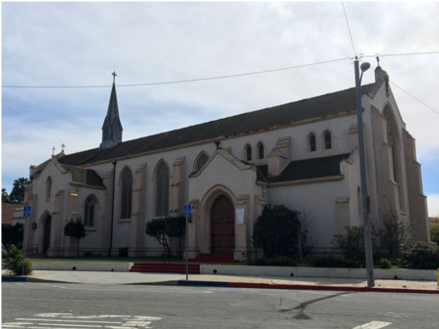
Holy Faith Episcopal Church, 260 N. Locust Street ( Southeast view ).
