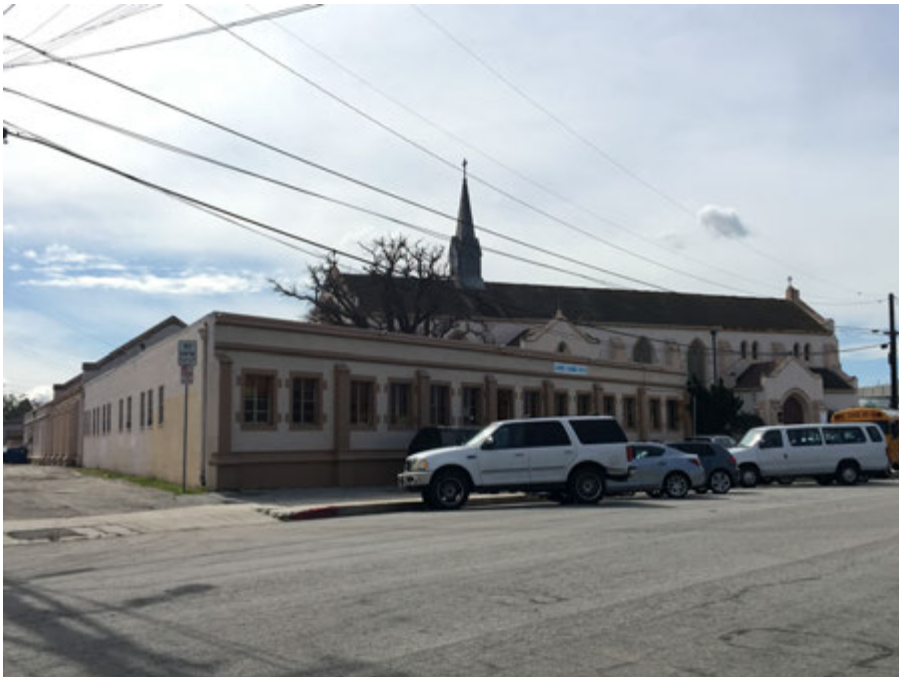
Holy Faith Episcopal Church and School, 260 N. Locust Street ( Southwest view ).
