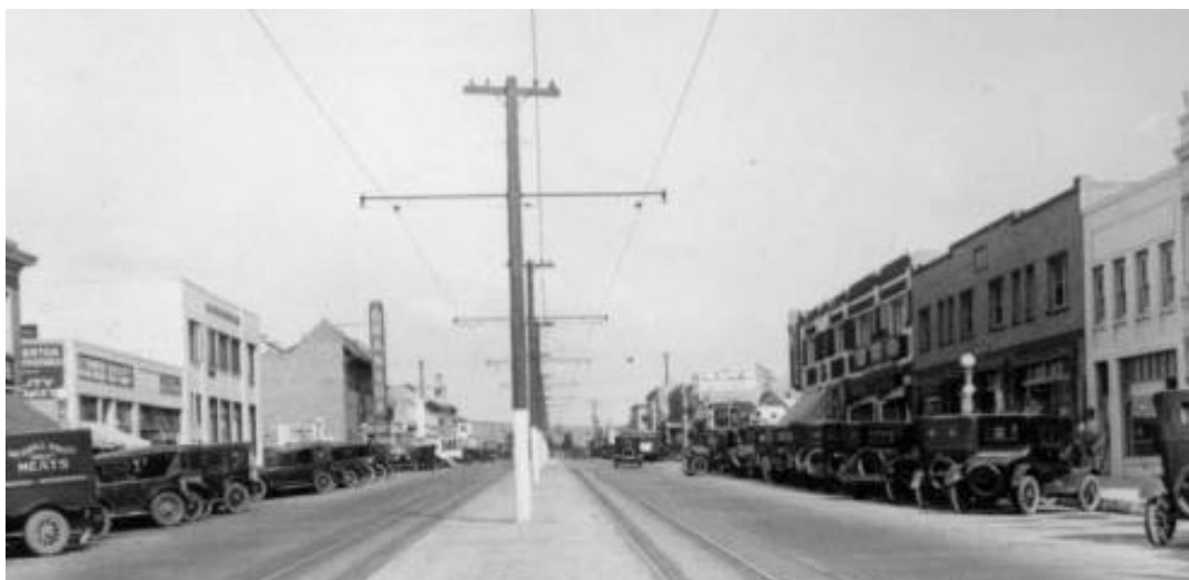
Market Street, looking north, 1925. ( Security Pacific National Bank Collection, LAPL )
