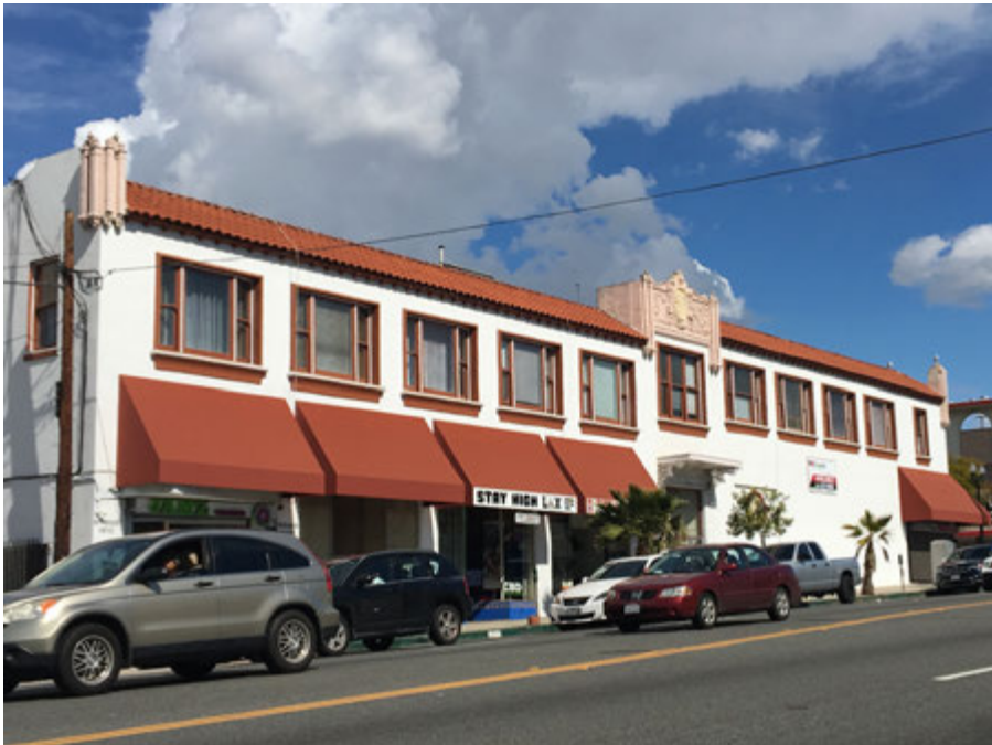
Professional Building, 149-155 S. Market Street/231-239 E. Manchester Boulevard, (Northeast view).
