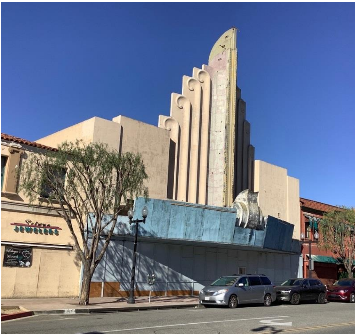
Figure 3 Fox Theatre Inglewood, East Elevation View Facing Northwest
