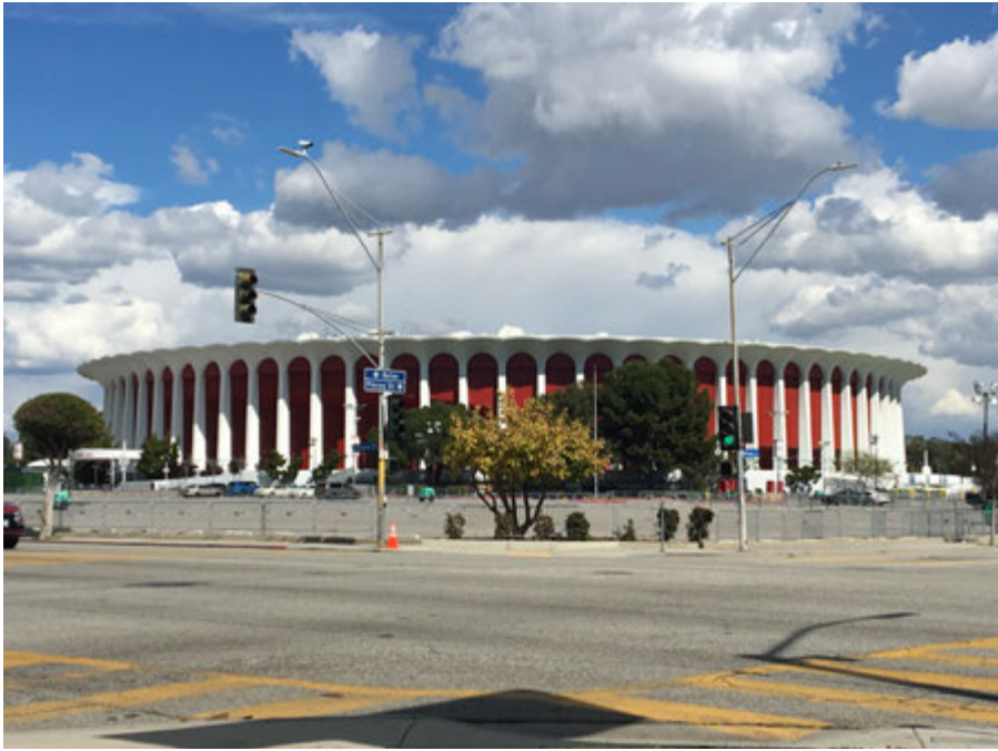
The Forum, 3900 W. Manchester Boulevard (East view) .
