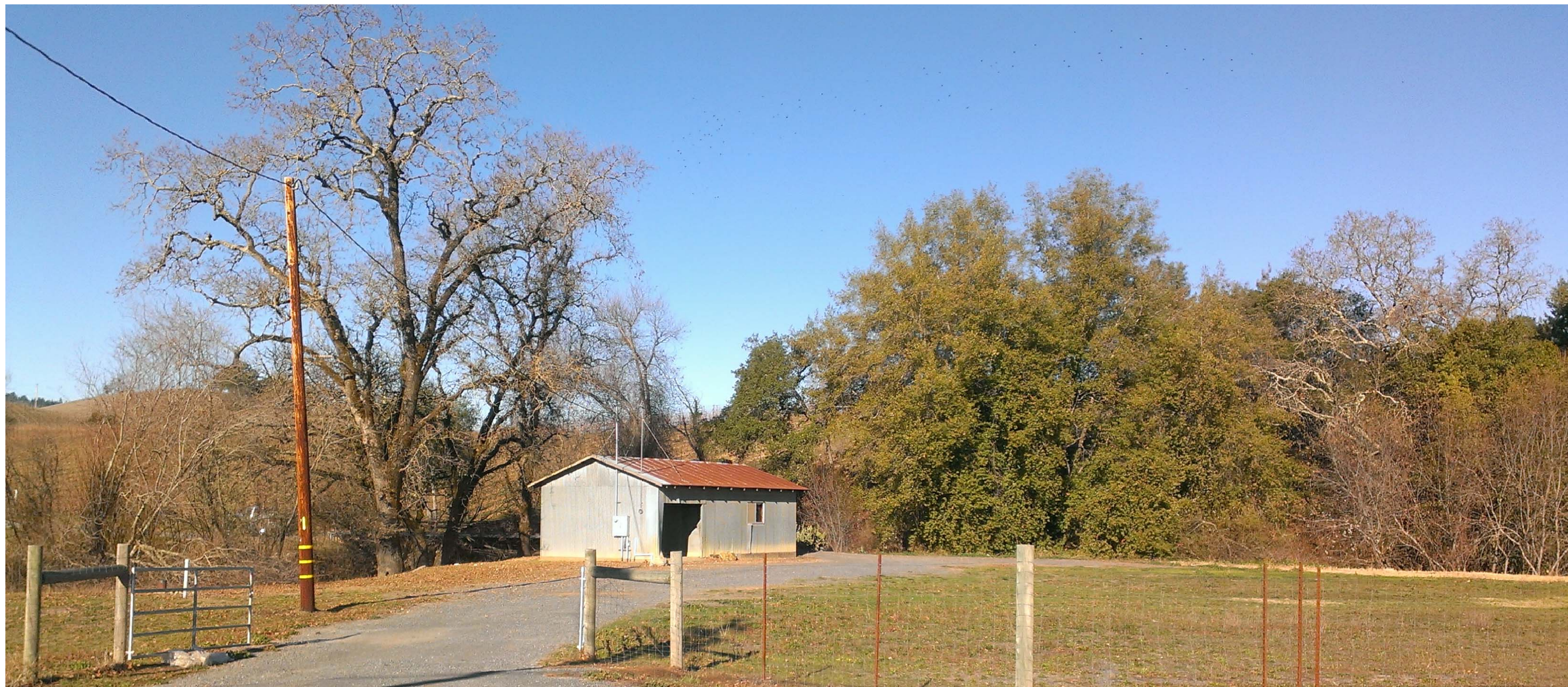
1 BEFORE – EXISTING GATE & AGRICULTURAL BUILDING
