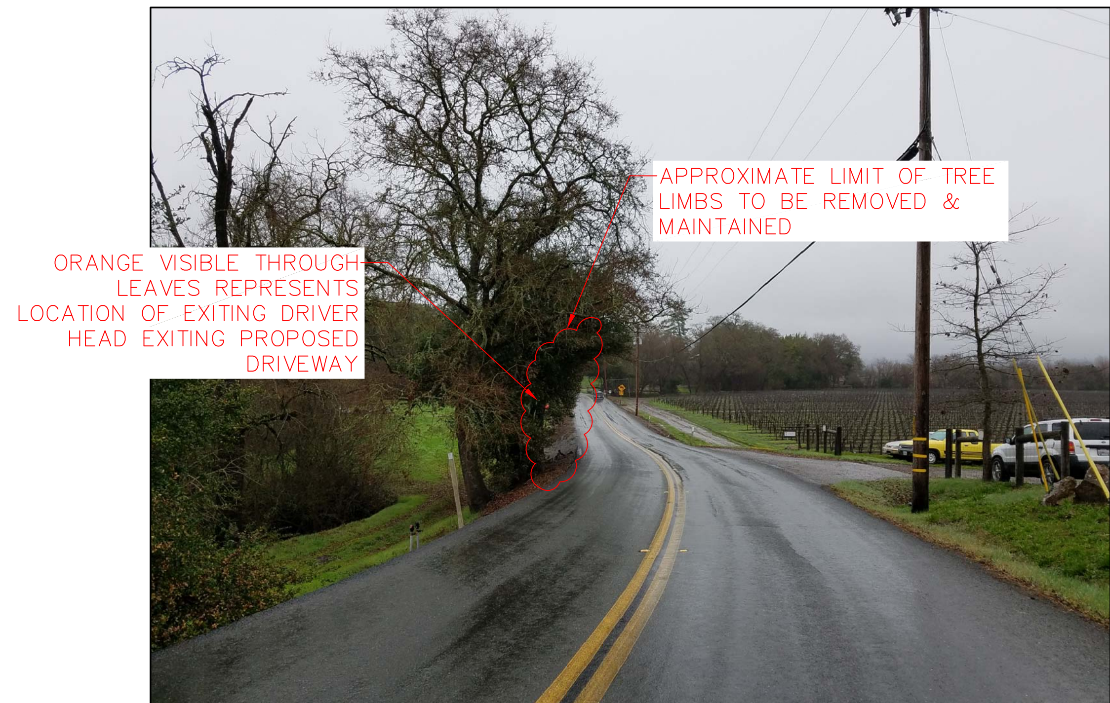
NORTHBOUND STOPPING SITE DISTANCE AT 343 FEET TO PROPOSED DRIVEWAY
