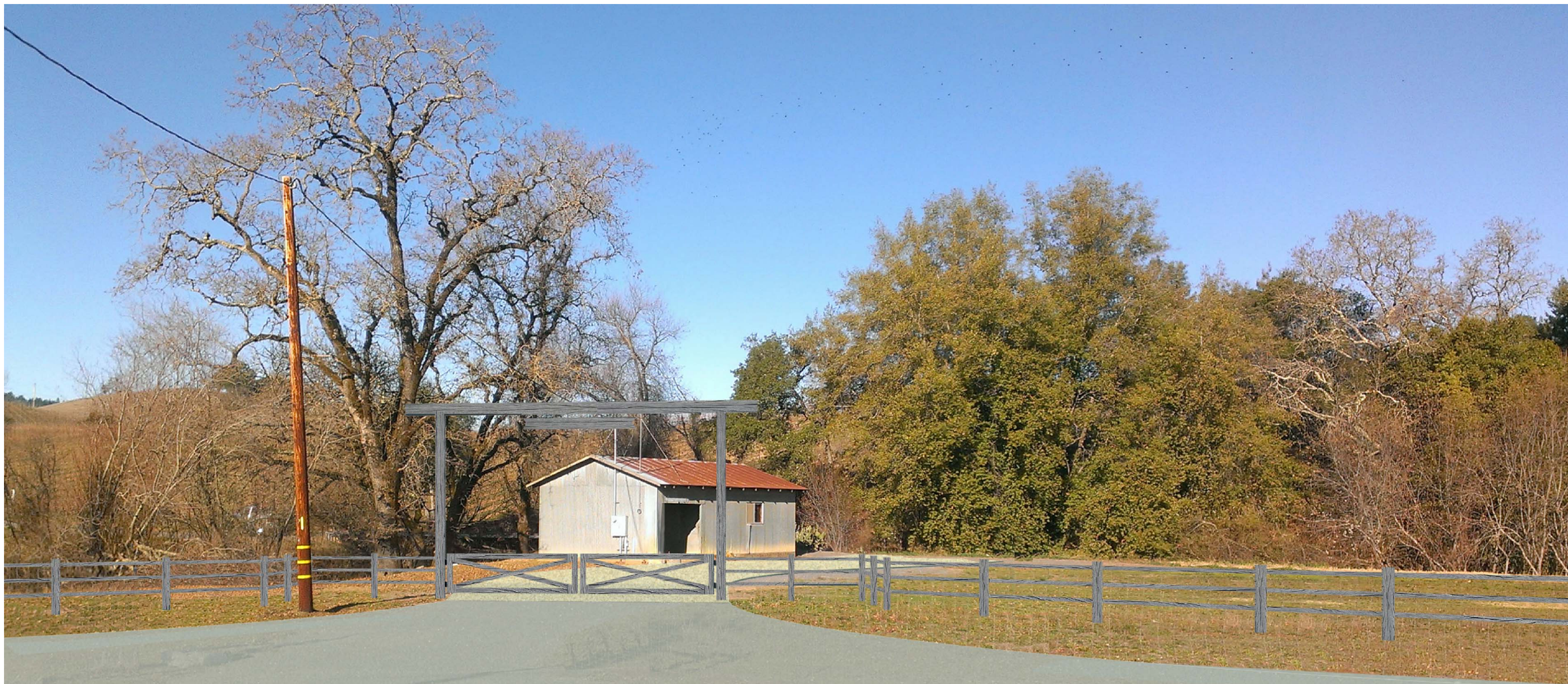
2 AFTER – NEW ENTRY GATE AND FENCE, AGRICULTURAL BUILDING TO REMAIN AS IS
