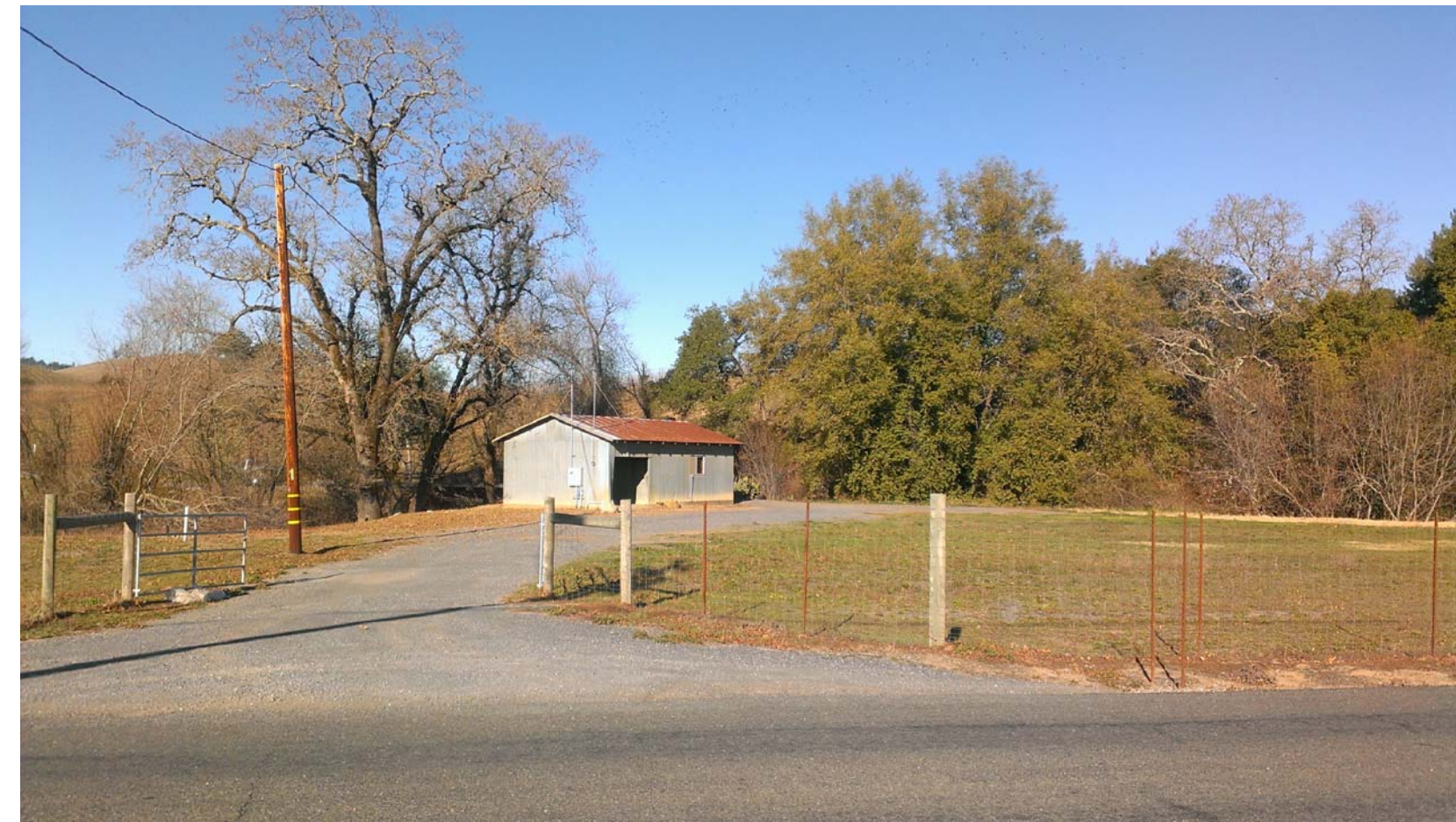
PHOTOGRAPH #1 EXISTING GATE TO ENTER SITE WILL BE UPGRADED W/ NEW FENCE & GATE
