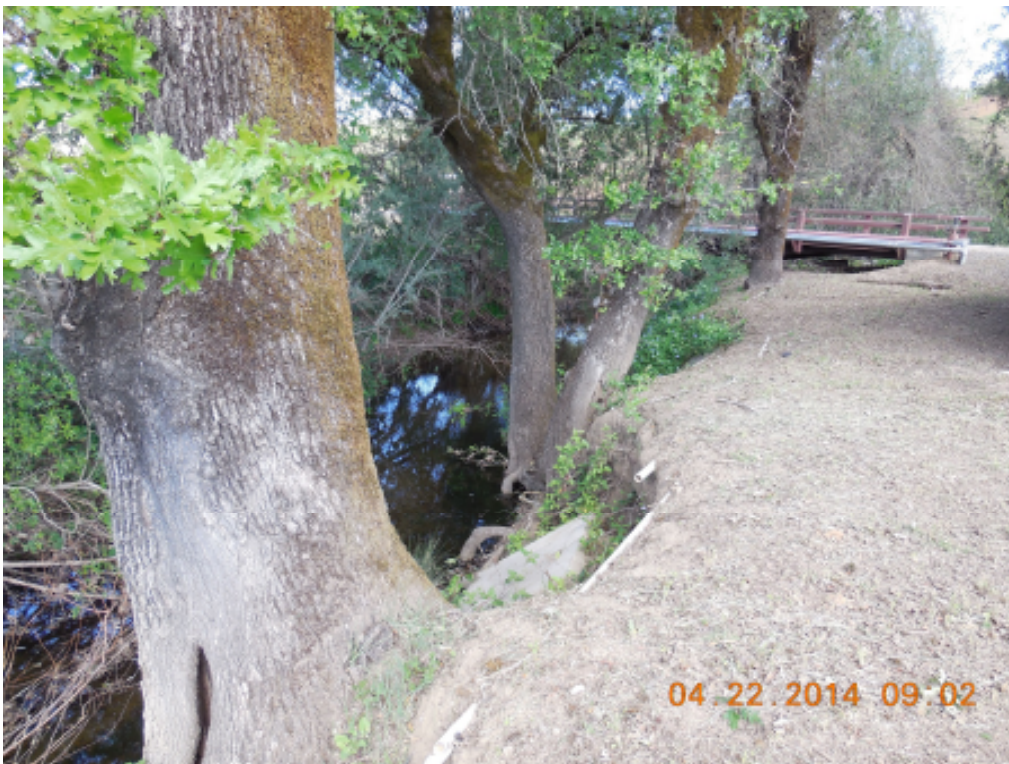
Figure 3. Approximate area of bridge crossing.
