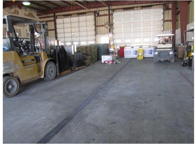
20. View east of the interior of the onsite Maintenance building and interior trench drain
