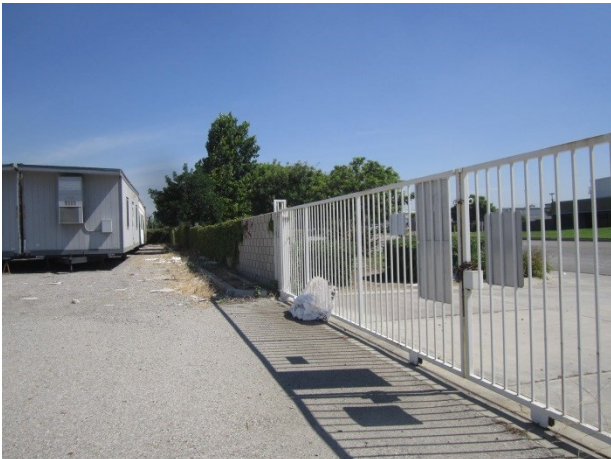
11. View of northern entrance on the east side of the subject property accessed from Beech Avenue
