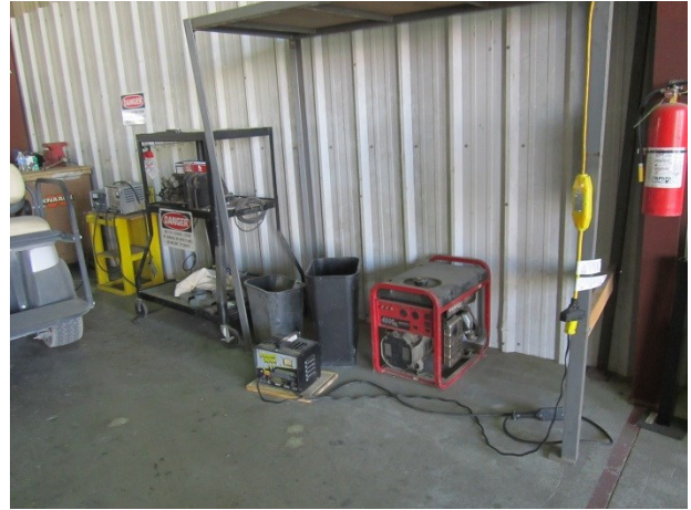
26. Portable electrical generator, welding equipment and forklift charger in the Maintenance Building
