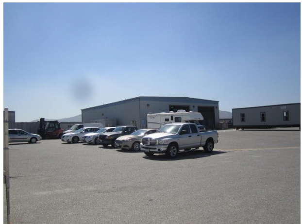
18. View to southeast of the maintenance building located near the center of the subject property
