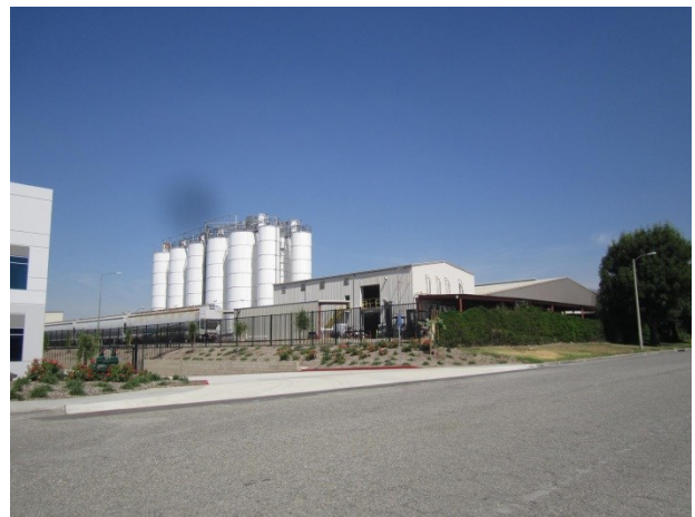
34. View to northwest of the adjacent property and railroad spur to the northwest
