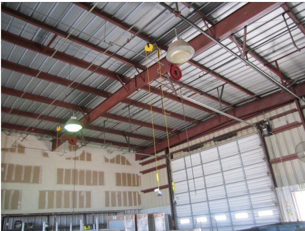
21. View of the interior ceiling of the Maintenance Building
