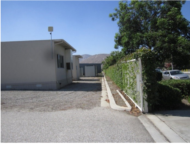
19. View south along the southern portion of the western boundary of the subject property
