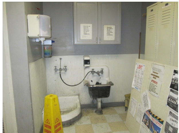
28. Janitorial storage closet in the maintenance building
