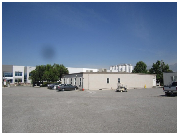
2. View west of the onsite modular office trailer used as the onsite headquarters
