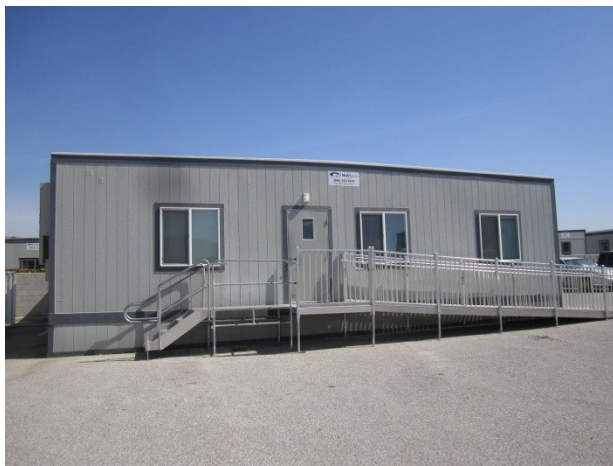
3. View to north of the "model" modular office trailer previously used for offices and storage
