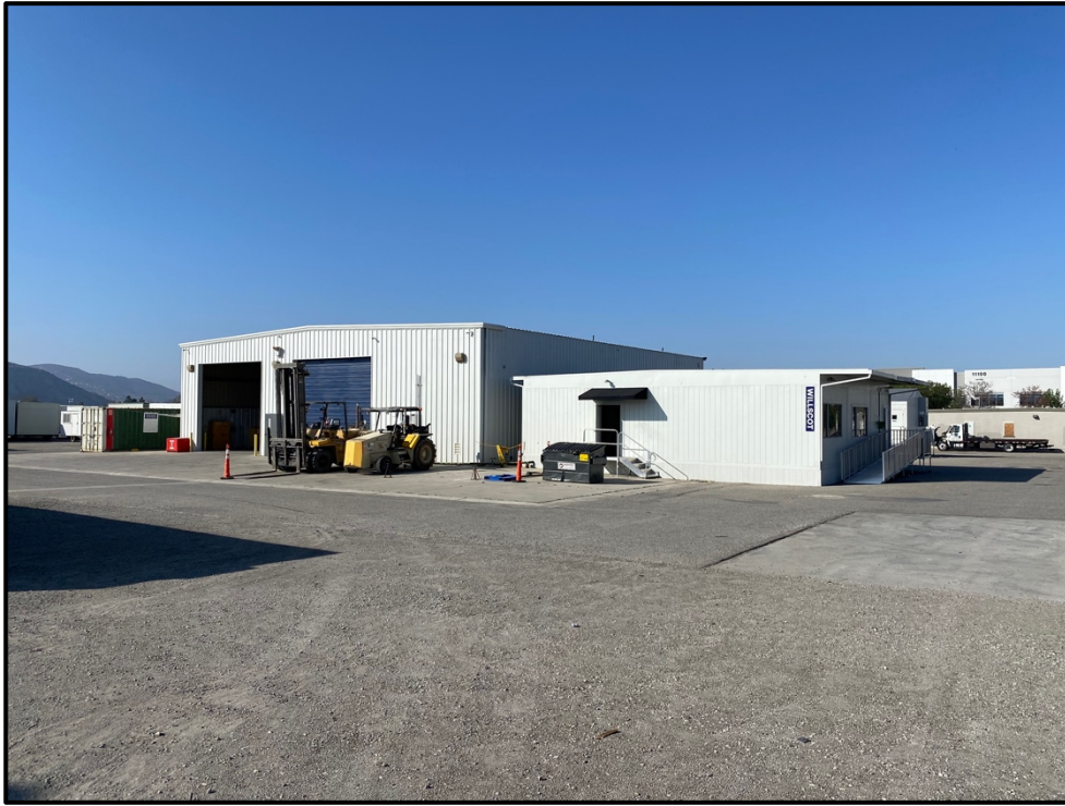
Plate 3.2–3: View of the steel warehouse and prefabricated buildings in the center of the property, facing southeast.
