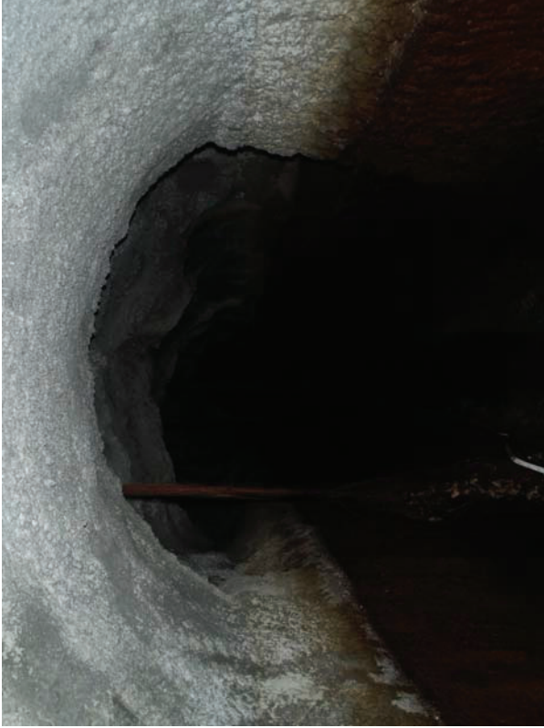
About 35' into tunnel, end cut/cover area
