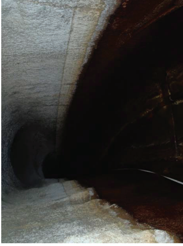
Curve area about 20' into tunnel
