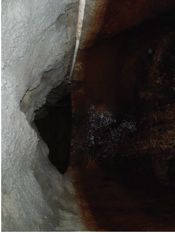
About 85' into tunnel - concrete dam
