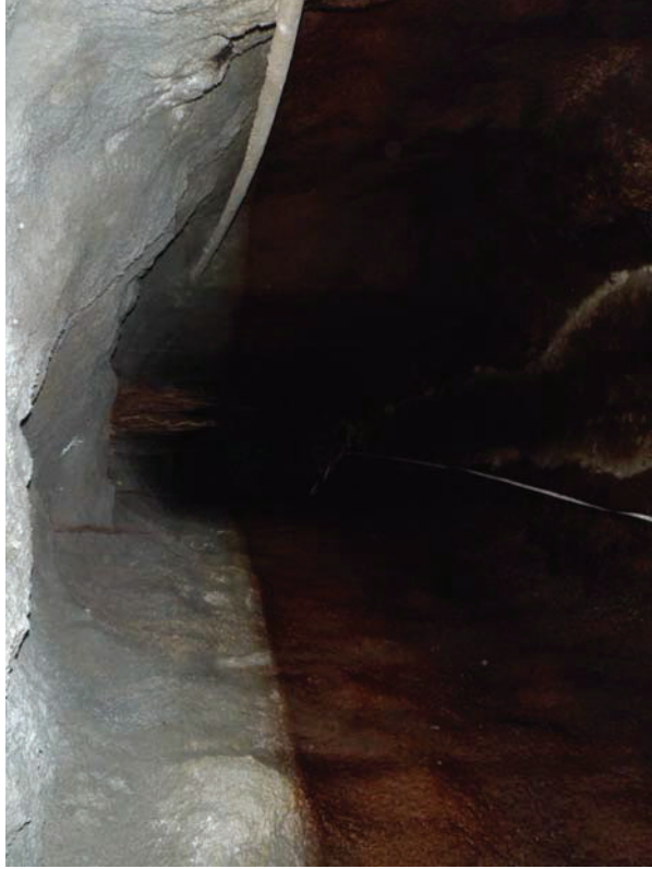
About 75' into tunnel
