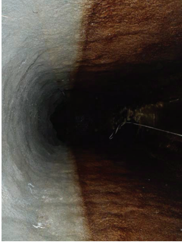
About 80' into tunnel
