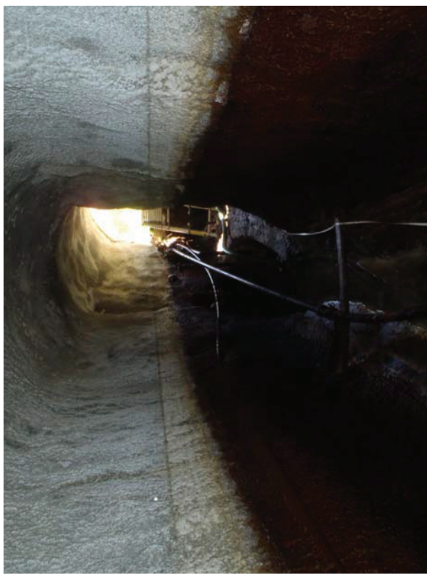
Inside tunnel at curve - view towards portal
