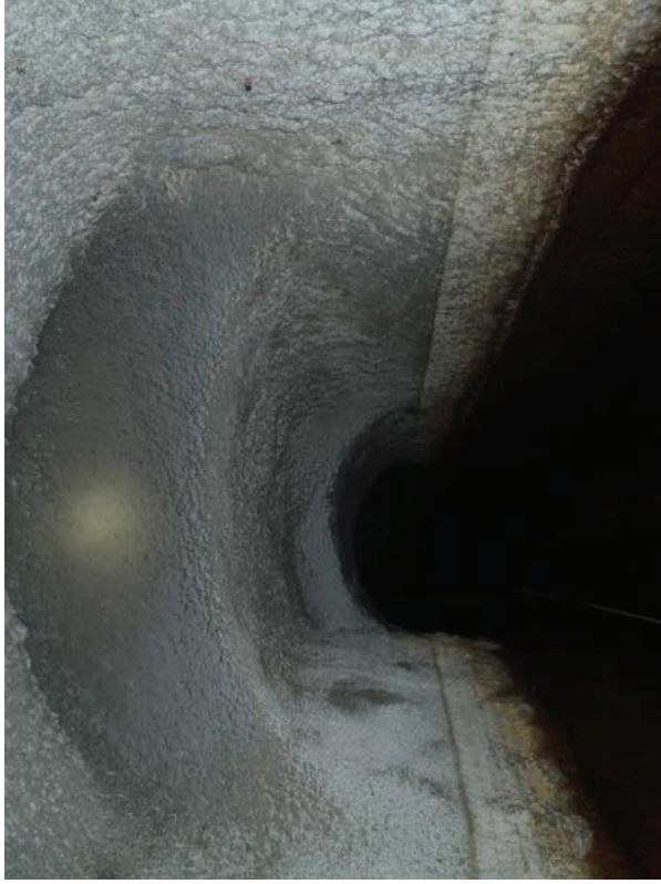
Curve area about 20' into tunnel
