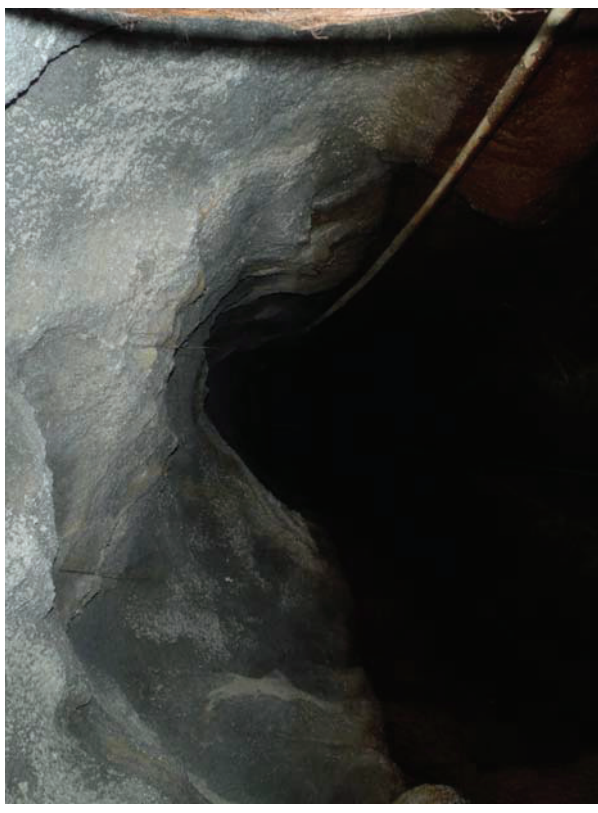
About 60' into tunnel
