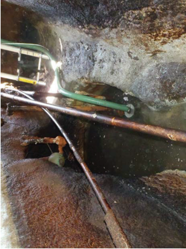
Sump inside portal
