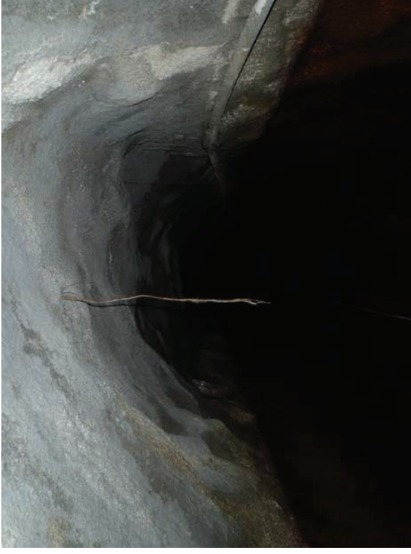
About 70' into tunnel
