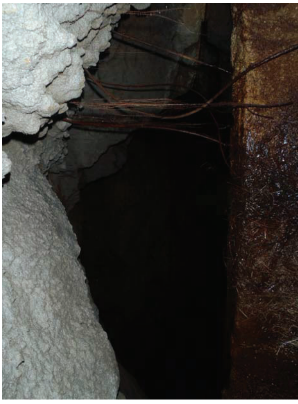
Top of dam to crown of tunnel about 12"
