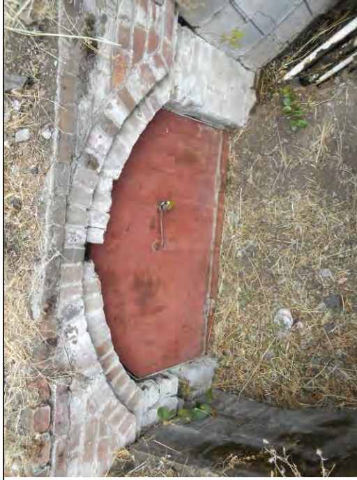
Close view of fresh water spring access door
