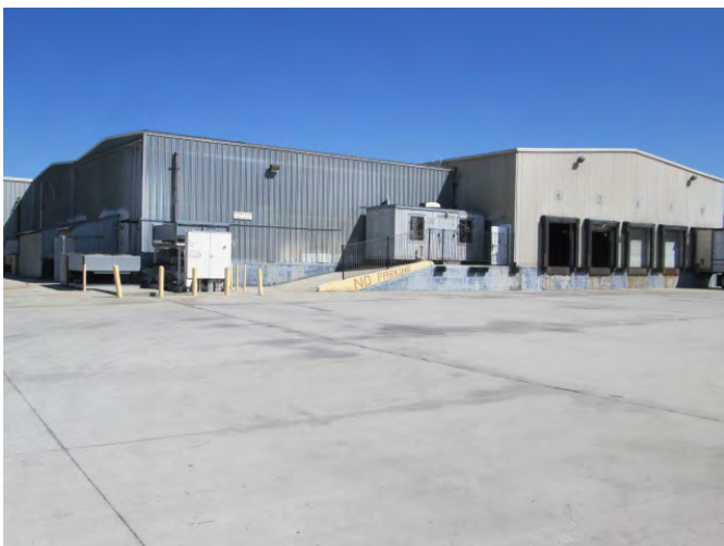
11. View of the southern portion of the warehouse.
