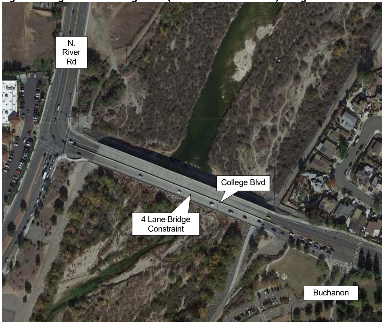
Figure 31: Segment #12 College Blvd (N. River Rd to Buchanon) Bridge Constraints
