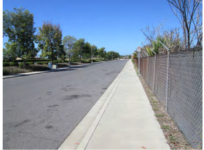
8. Western view along the southern fence line of the Site along Calle Joven.
