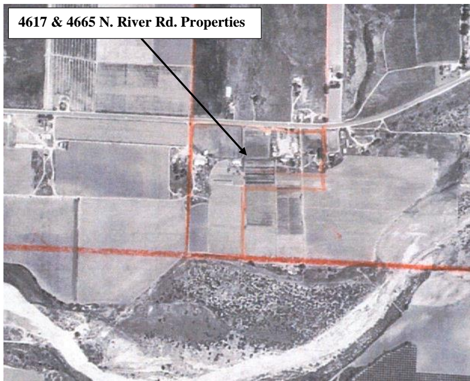
Figure 9 Proposed Project Location on 1967 Aerial Photograph
