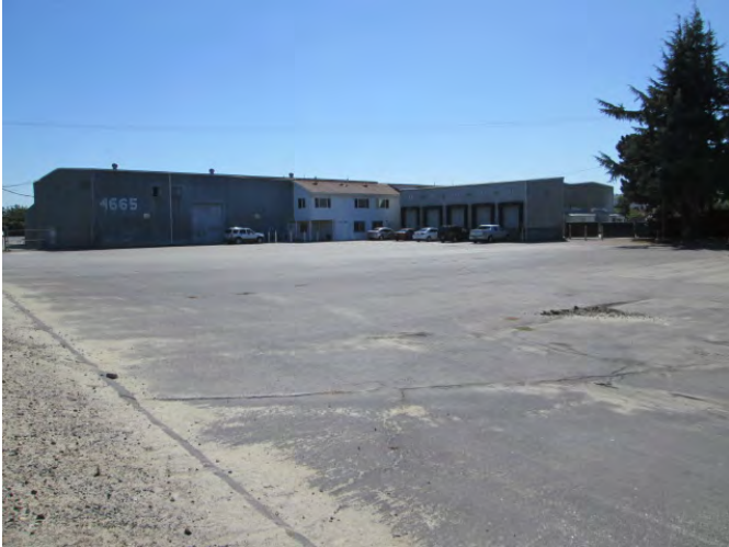
1. Southeastern view of the Site.
