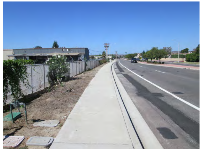
6. Western view along N River Road View from the northeast corner of the Site.
