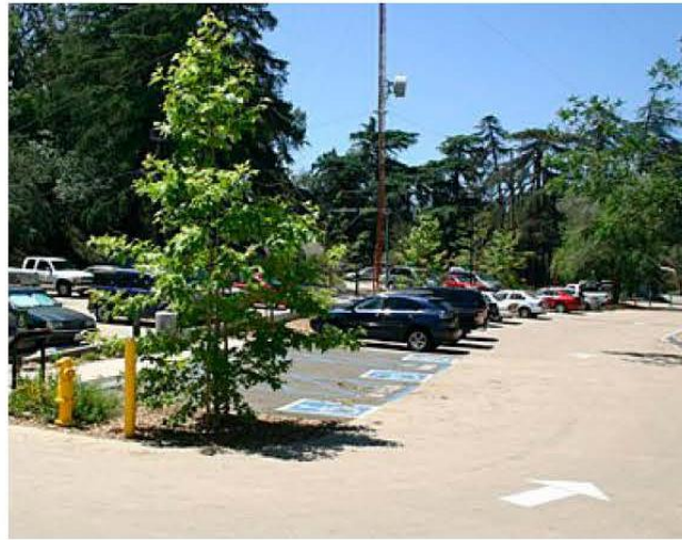
ASPHALT AND AGGREGATE PAVING
