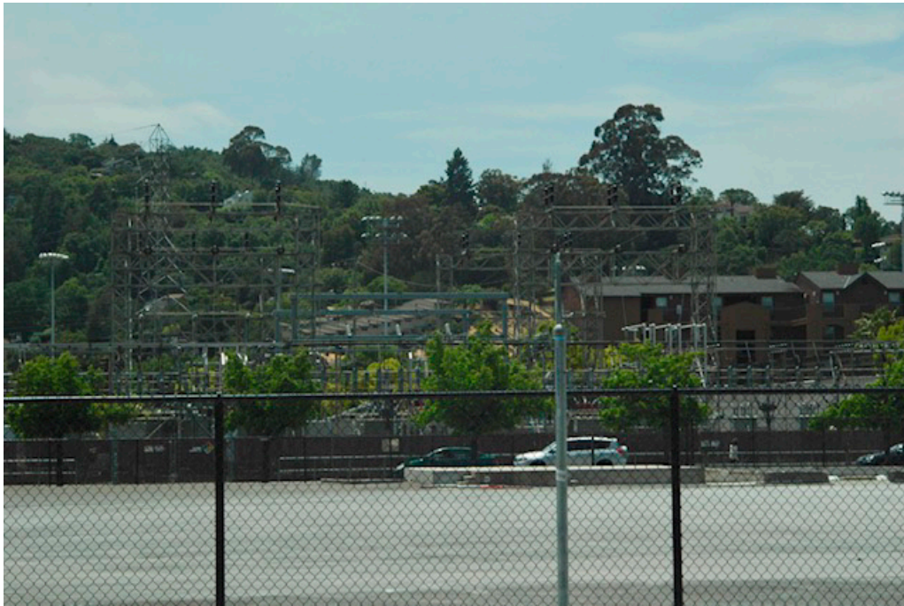
a. View south across site from 3rd Street with apartments in background (right) and PG&E substation towers in background (left).
