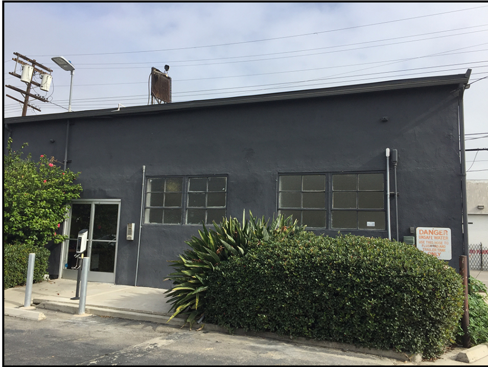
Figure 4: The west side of the S. Hewitt Street frontage building.
