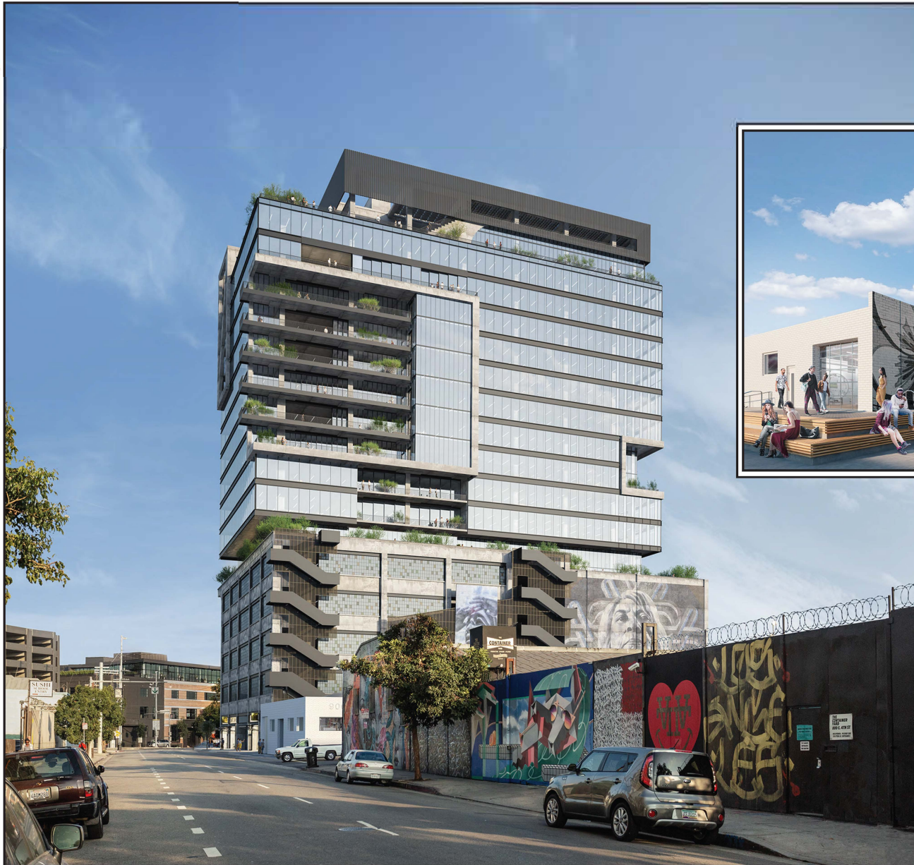
View of the west elevation from East 4 th Street.
