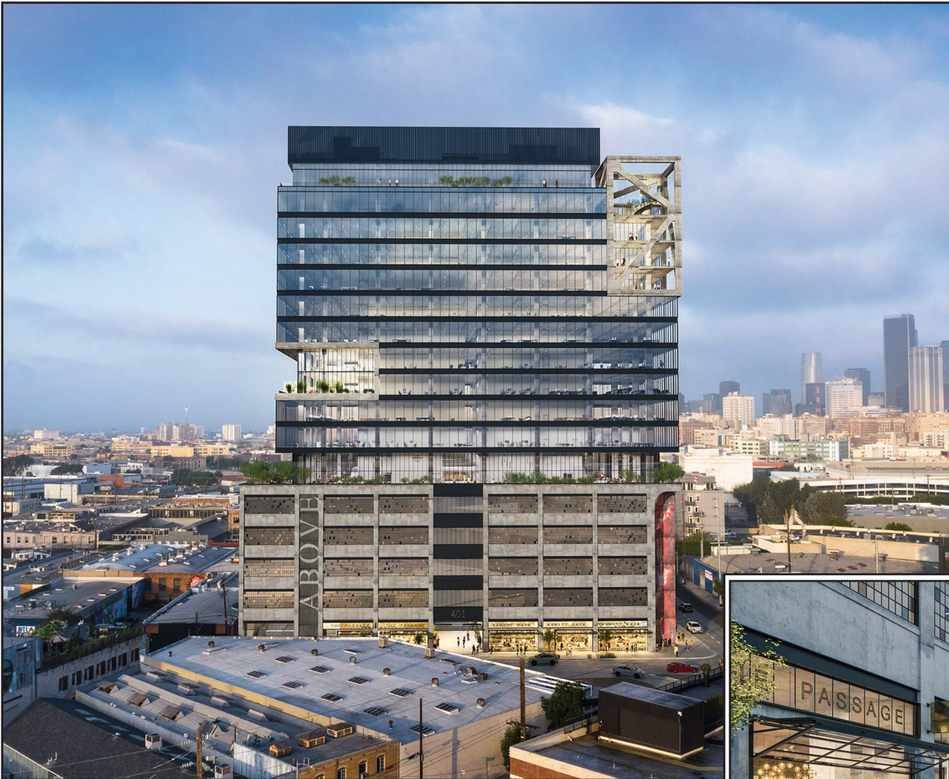
View of the South Hewitt Street (east) elevation.
