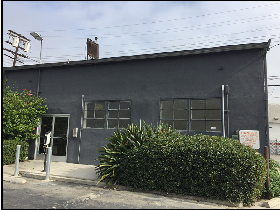
Figure 4: View of the west side of the South Hewitt Street frontage building.
