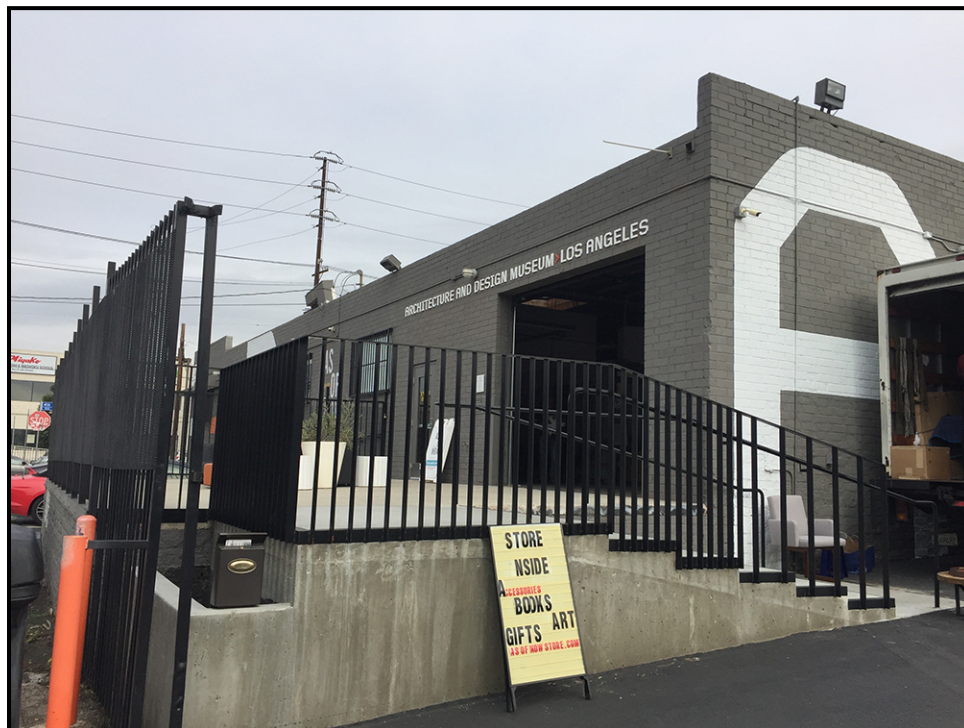
Figure 3: View of the west side of the building formerly occupied by the A+D Museum that fronts Colyton Street.
