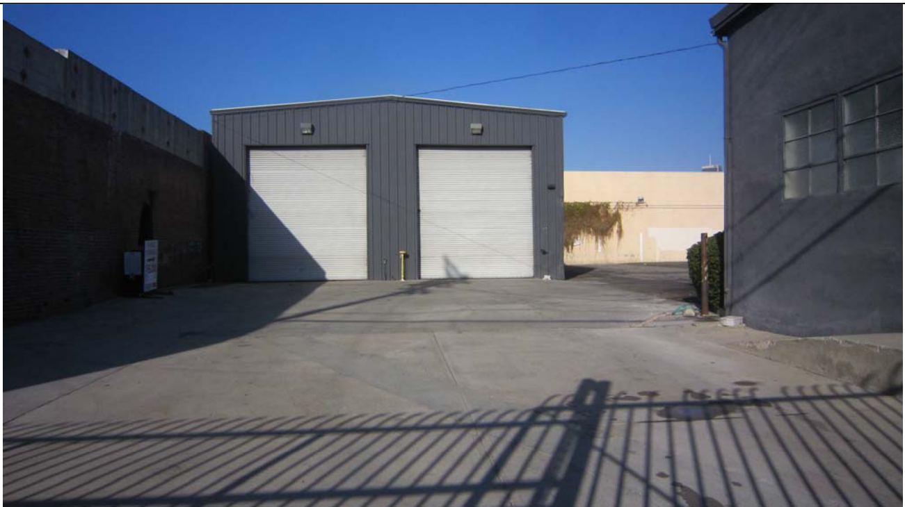
PHOTO 6: View of the Site garage building, looking west.
