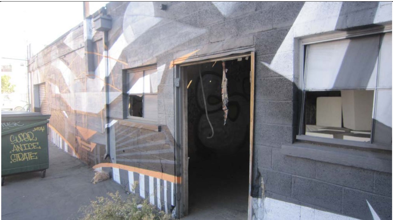
PHOTO 16: Another view of the storage structure, looking northeast.
