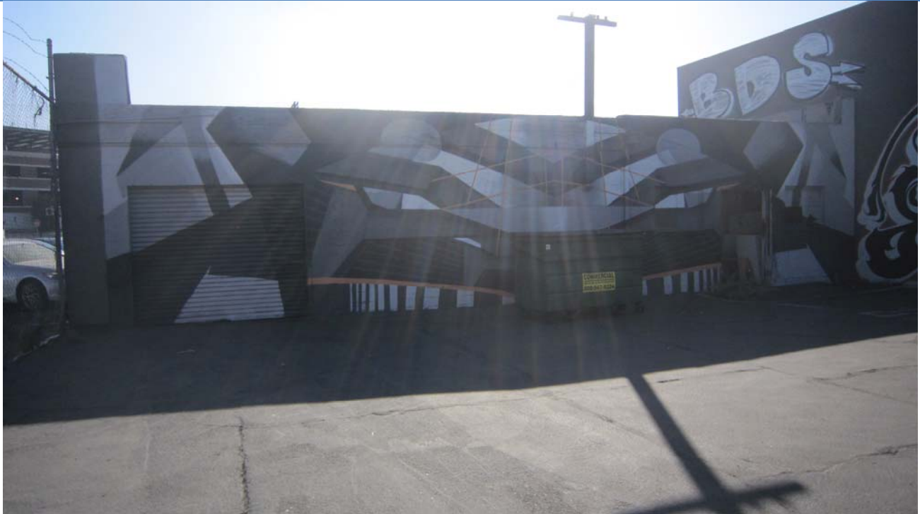
PHOTO 15: View of the storage structure, looking east.
