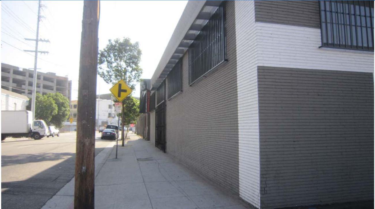
PHOTO 9: View of the museum building, looking east.
