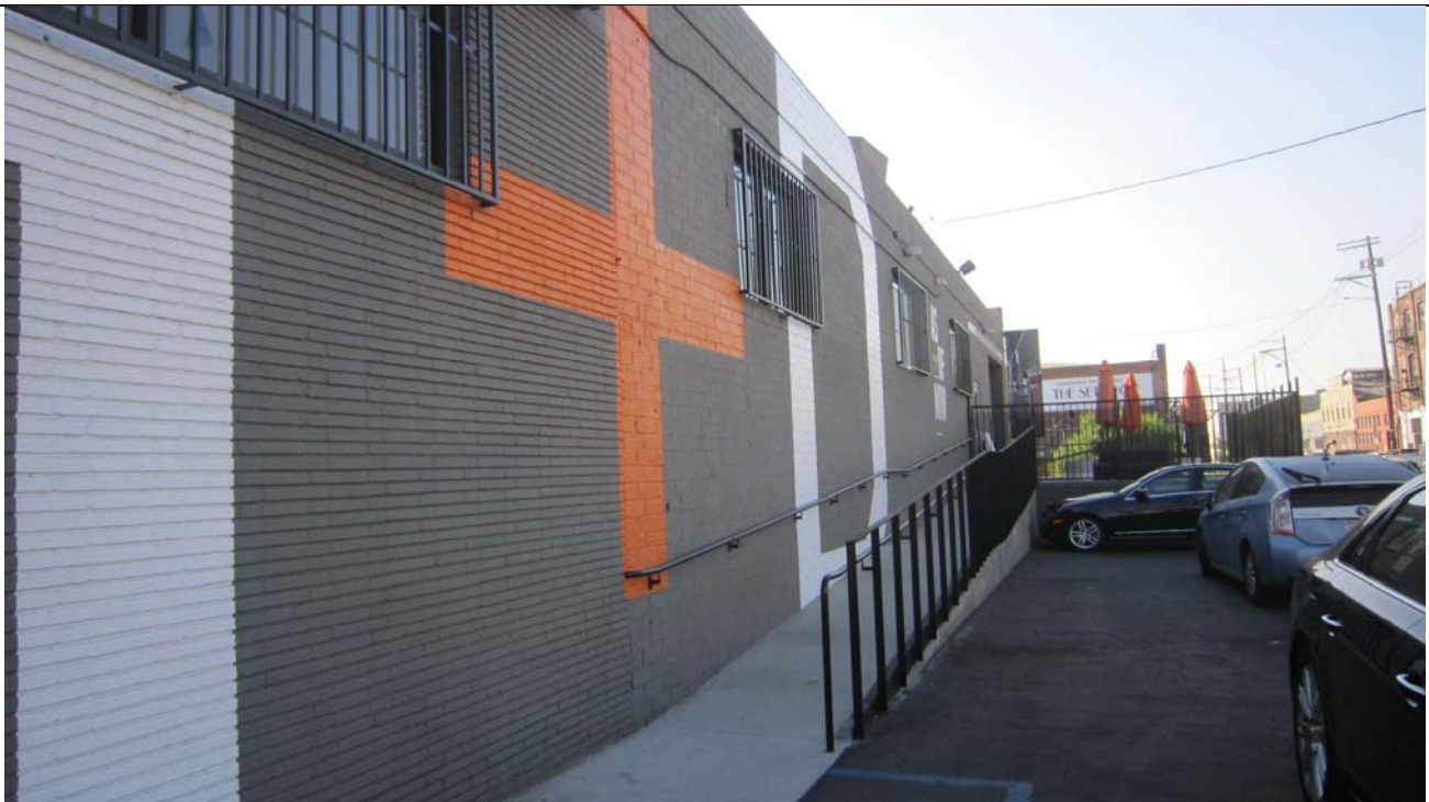
PHOTO 10: View of the museum building, looking south.
