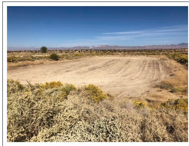
Dry basin at the Wastewater Treatment Plant.
