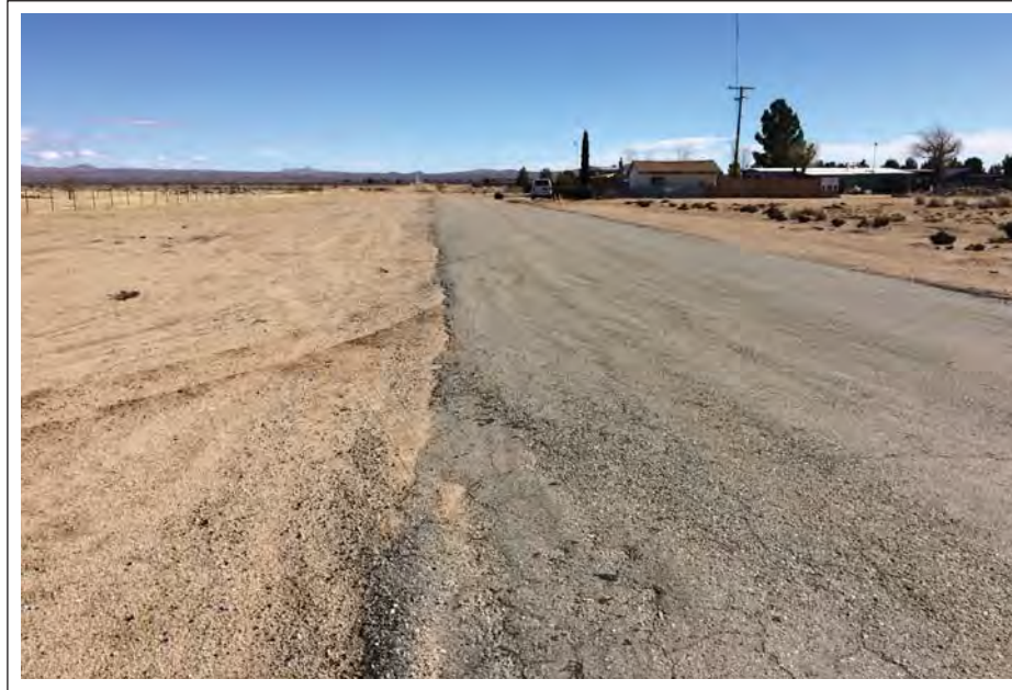
Disturbed (left) and developed (right) areas at the western end of the utility alignment.
