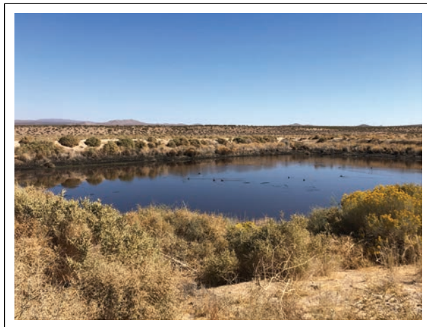
Inundated basin at the Wastewater Treatment Plant.
