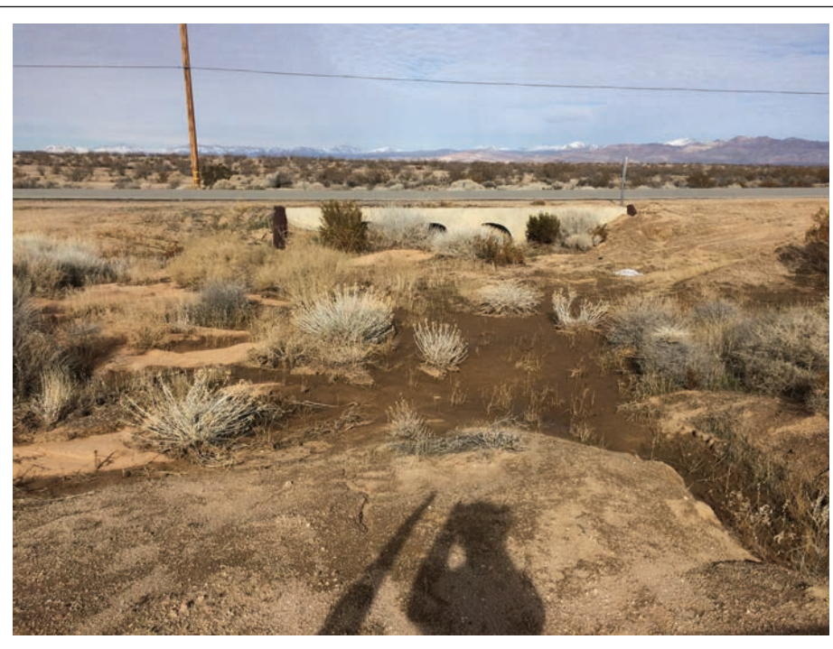
Utility Alignment Drainage 9.
