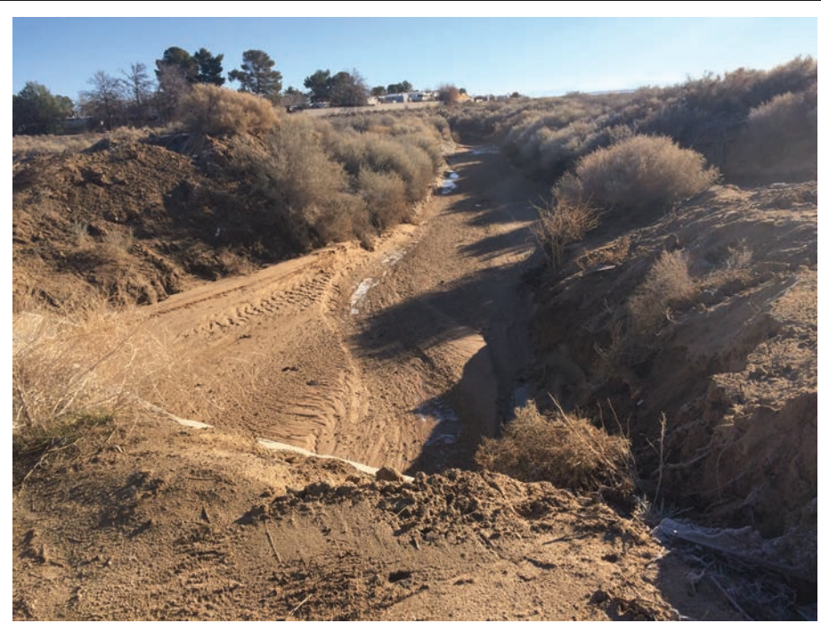
Utility Alignment Drainage 6.
