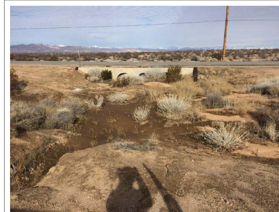
Utility Alignment Drainage 9.
