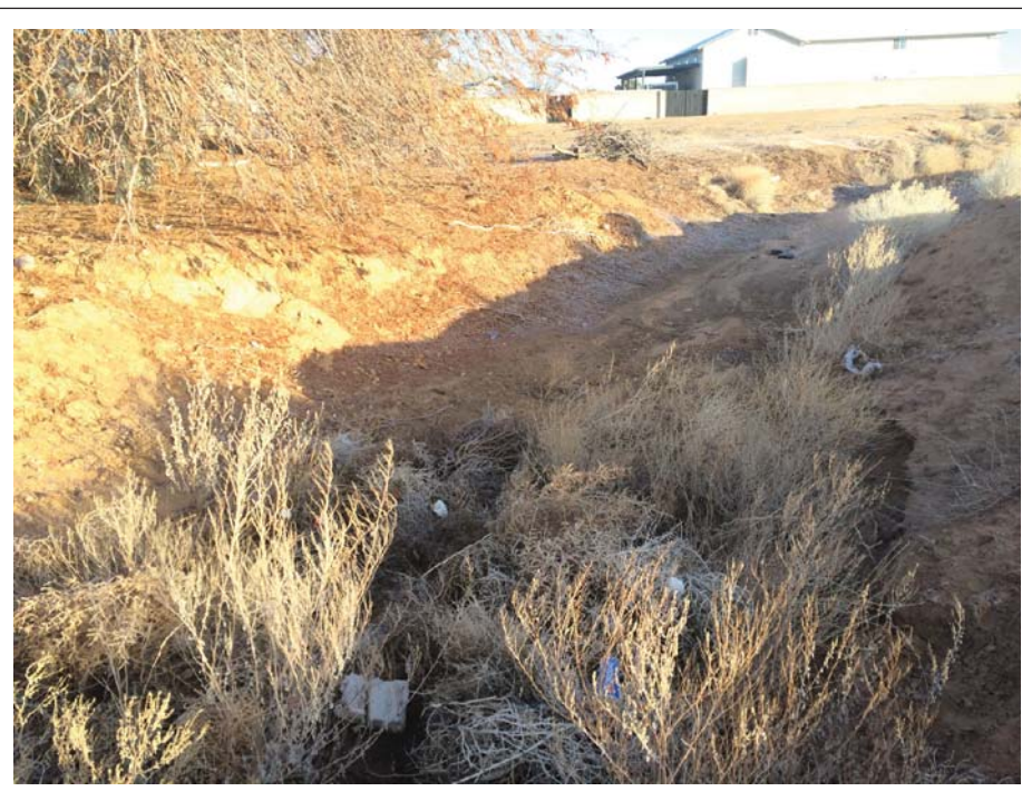
Utility Alignment Drainage 4.
