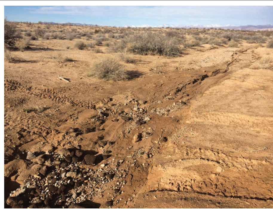
Utility Alignment Drainage 7.
