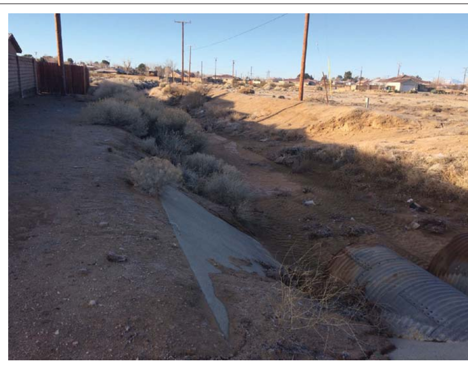
Utility Alignment Drainage 5.
