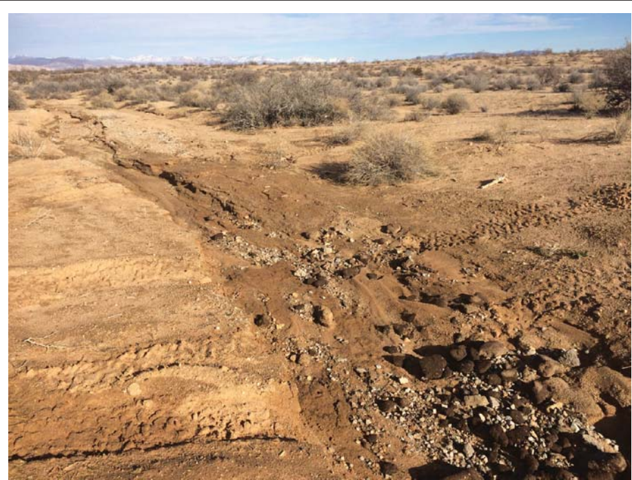
Utility Alignment Drainage 7.
