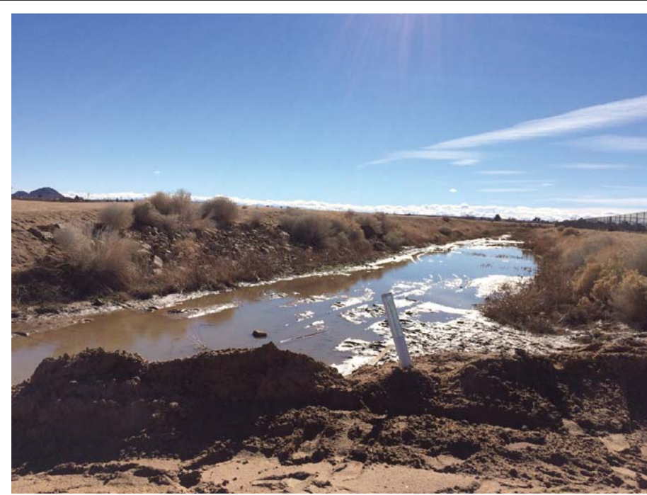
Utility Alignment Drainage 2.
