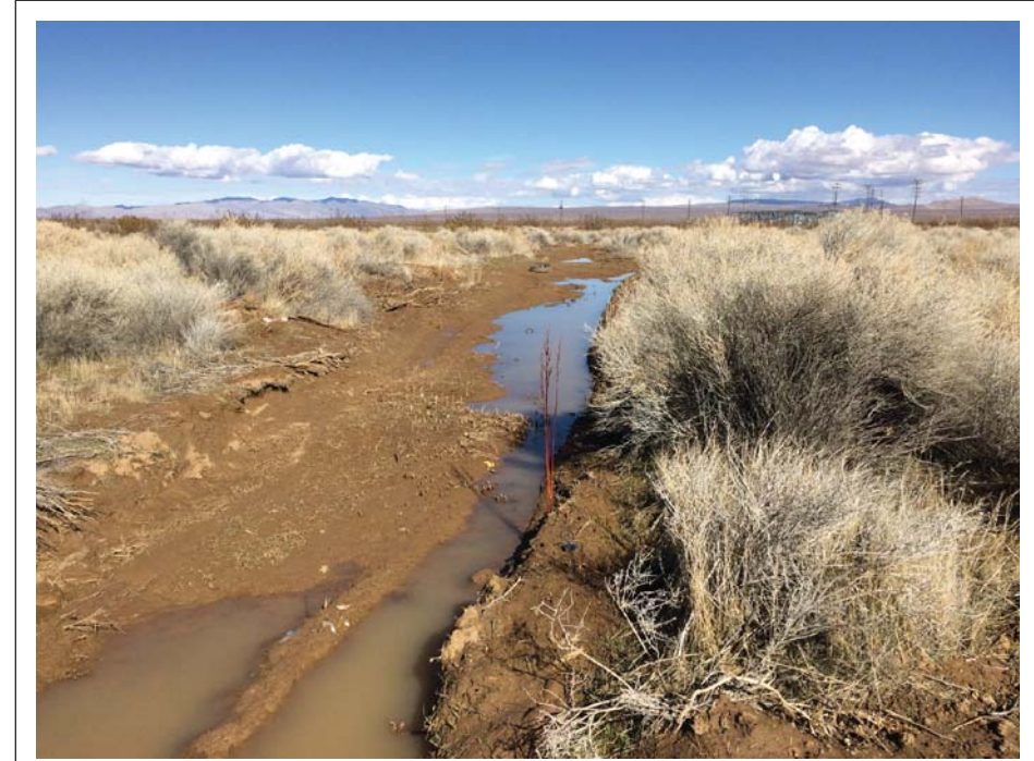
Utility Alignment Drainage 3.
