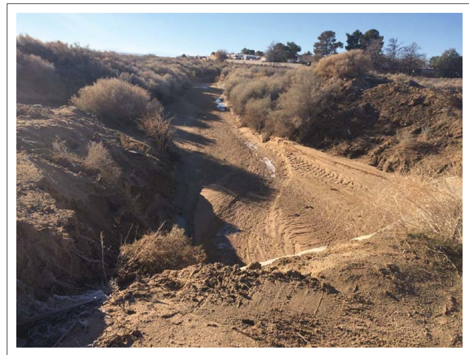
Utility Alignment Drainage 6.
