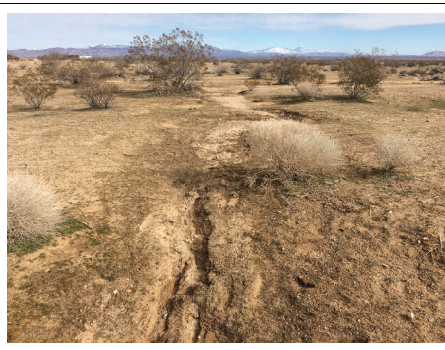
Utility Alignment Drainage 10.
