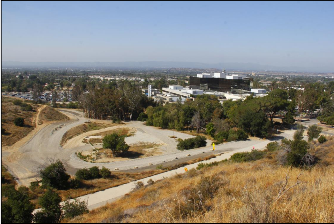
Photo 3B Alt. From Wilson Canyon Debris Basin, Facing Southwest toward Main Campus
