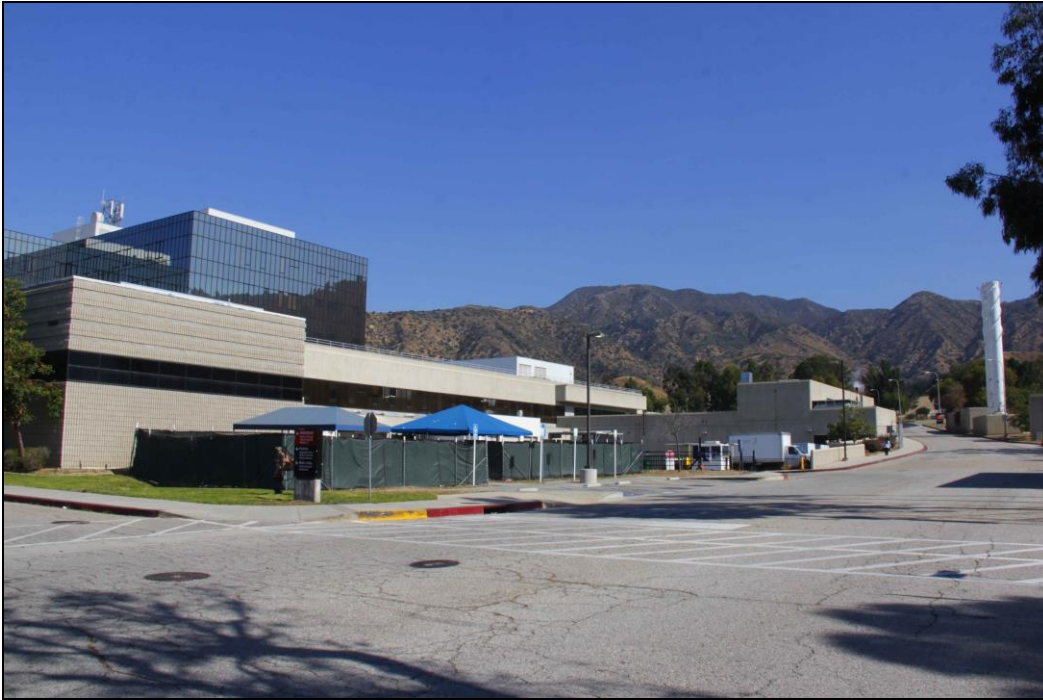
Photo 2A. From Reagan Road, Facing Northwest toward the Existing Hospital Building, Emergency Services, Central Plant, and San Gabriel Mountains
