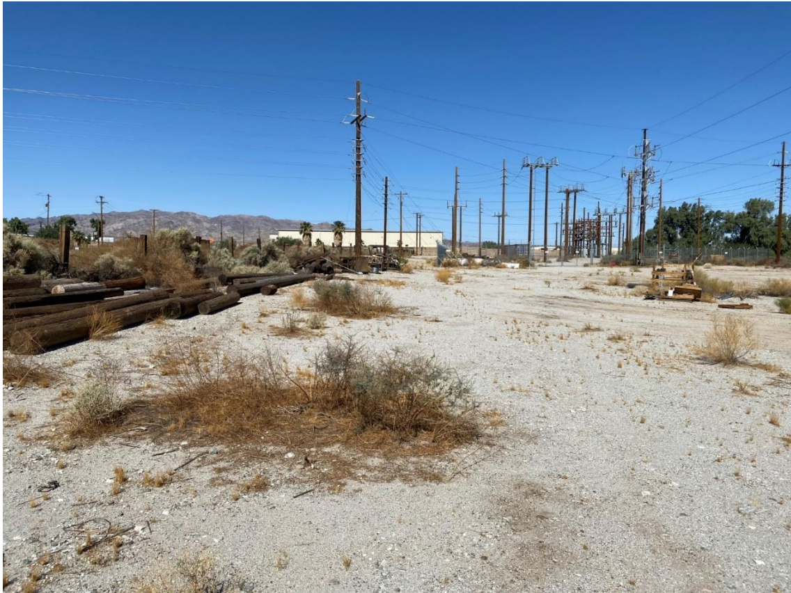
Photo 1 – Southern corner of Project site, facing west. Directly behind proposed concrete pad for pump.
