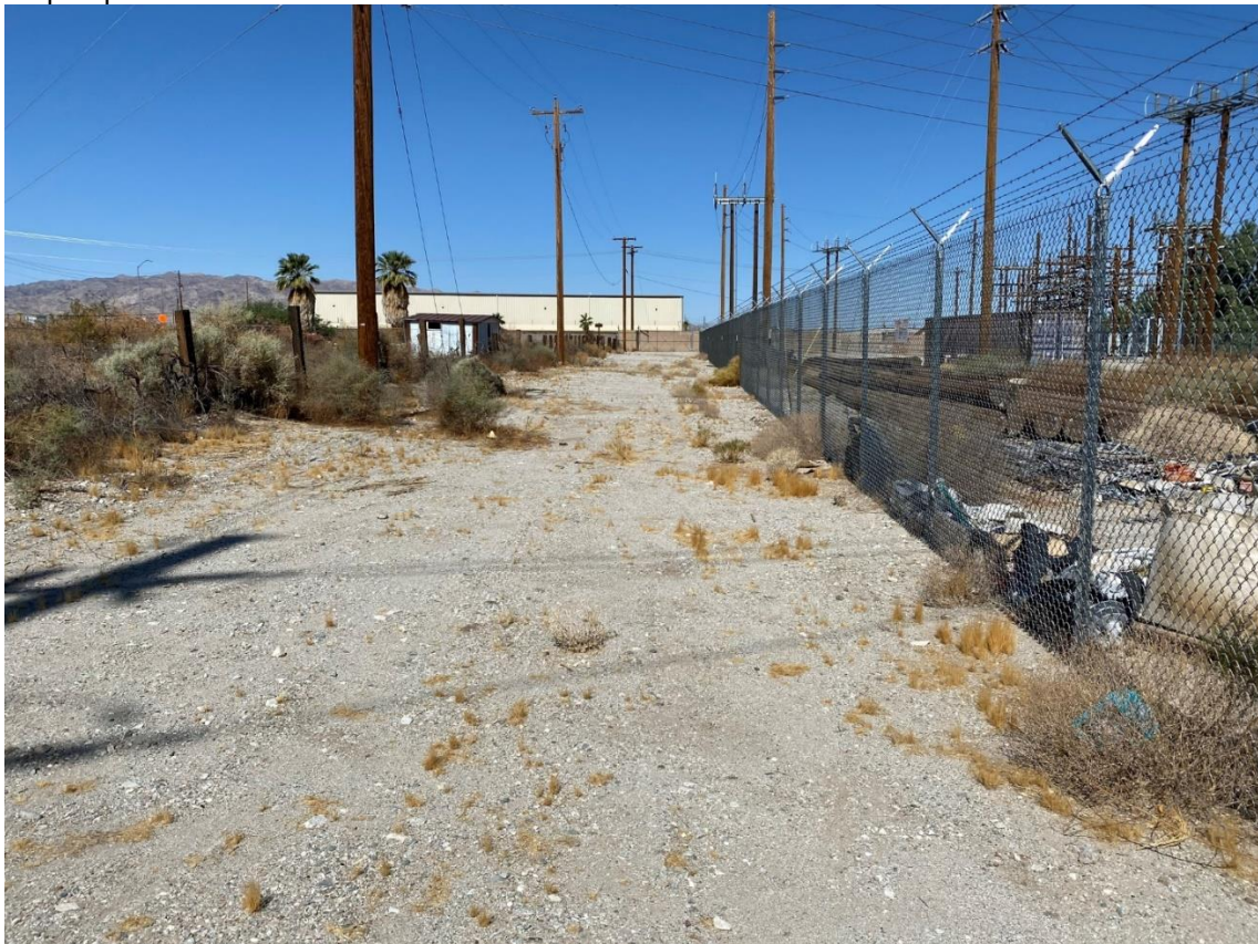
Photo 2 – Southern edge of Project site, facing west. Adjacent to the southern corner of the sub-station fence, along proposed access road.
